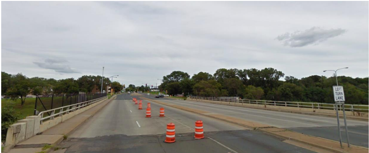
Figure 1. Photo. Existing Maryland Ave. bridge 6513 surface.
