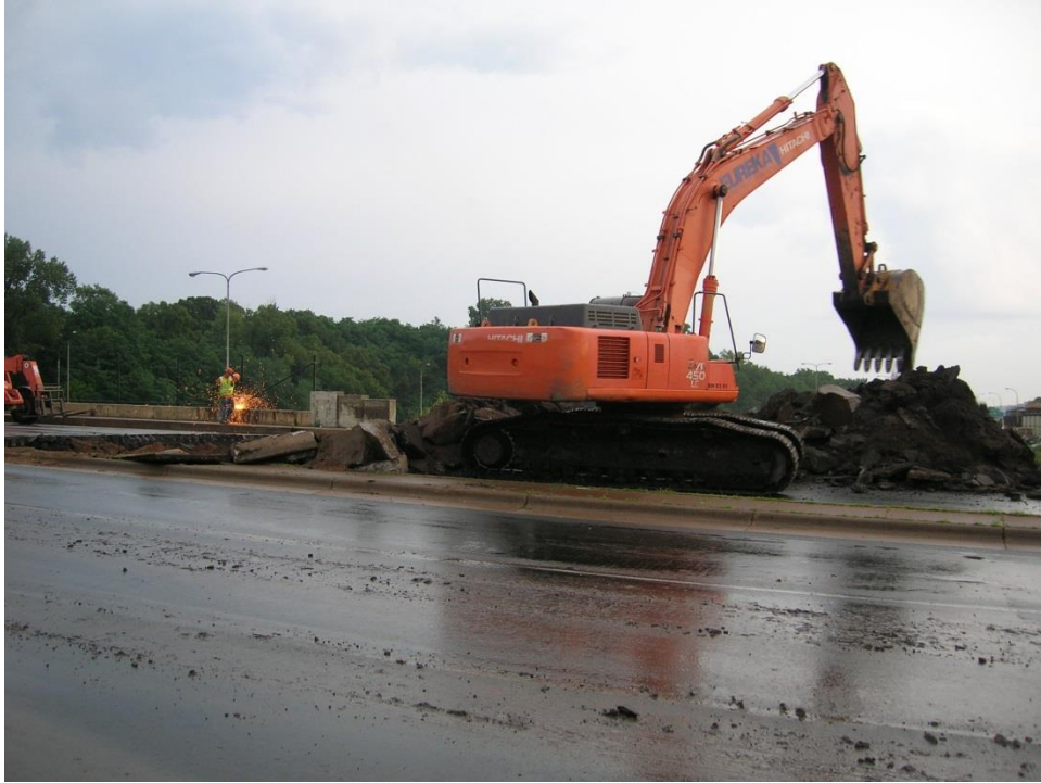
Figure 40. Photo. Demolishing Maryland Ave. bridge 6513.
