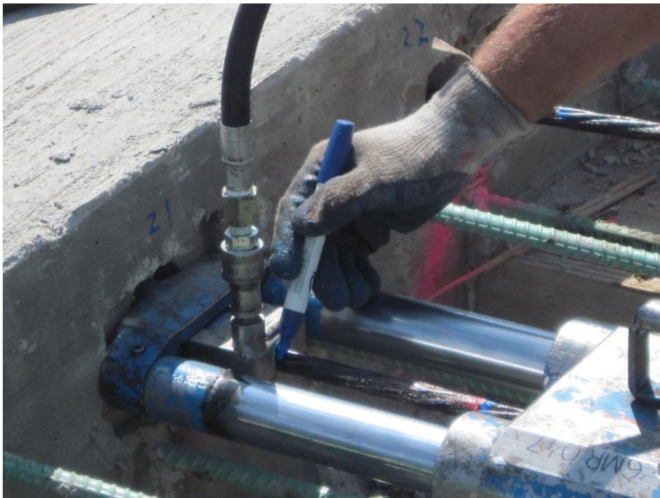
Figure 38. Photo. Close-up view of stressing the post-tensioning cables.
