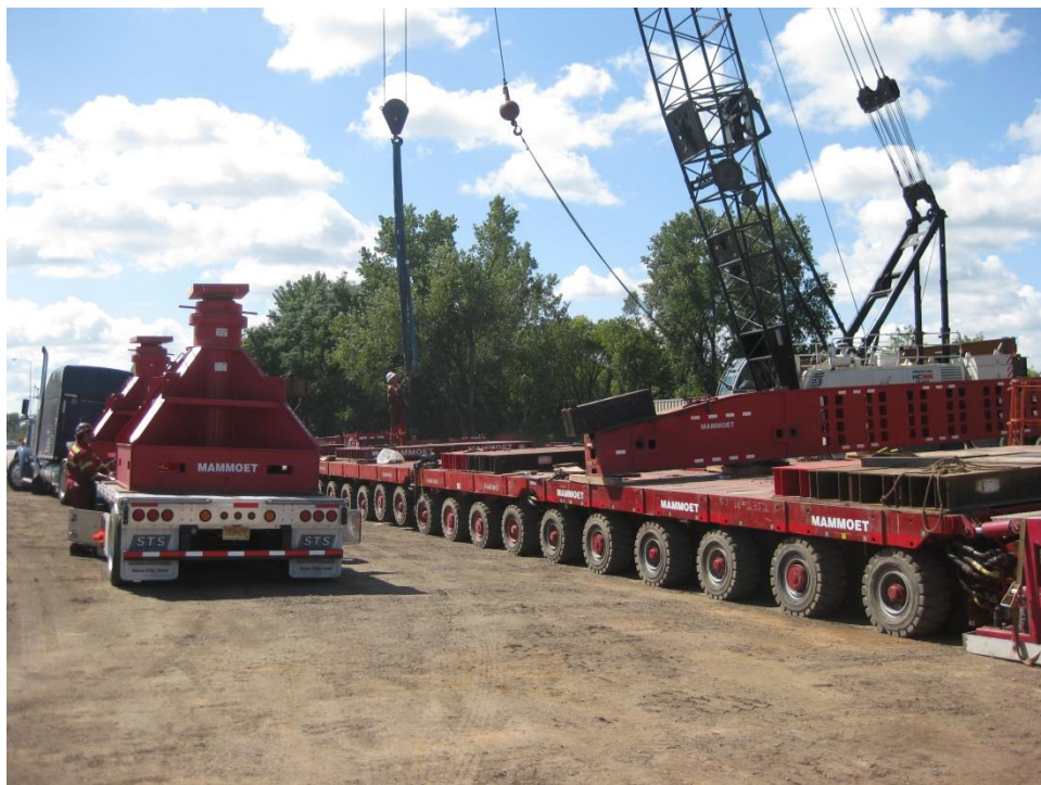
Figure 61. Photo. The SPMT was stripped down and shipped to the job site on a total of 30 flatbed trucks and reassembled at the job site for this project.
