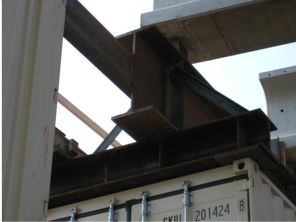
Figure 19. Photo. Girder resting on the bearing pads supported by the falsework.
