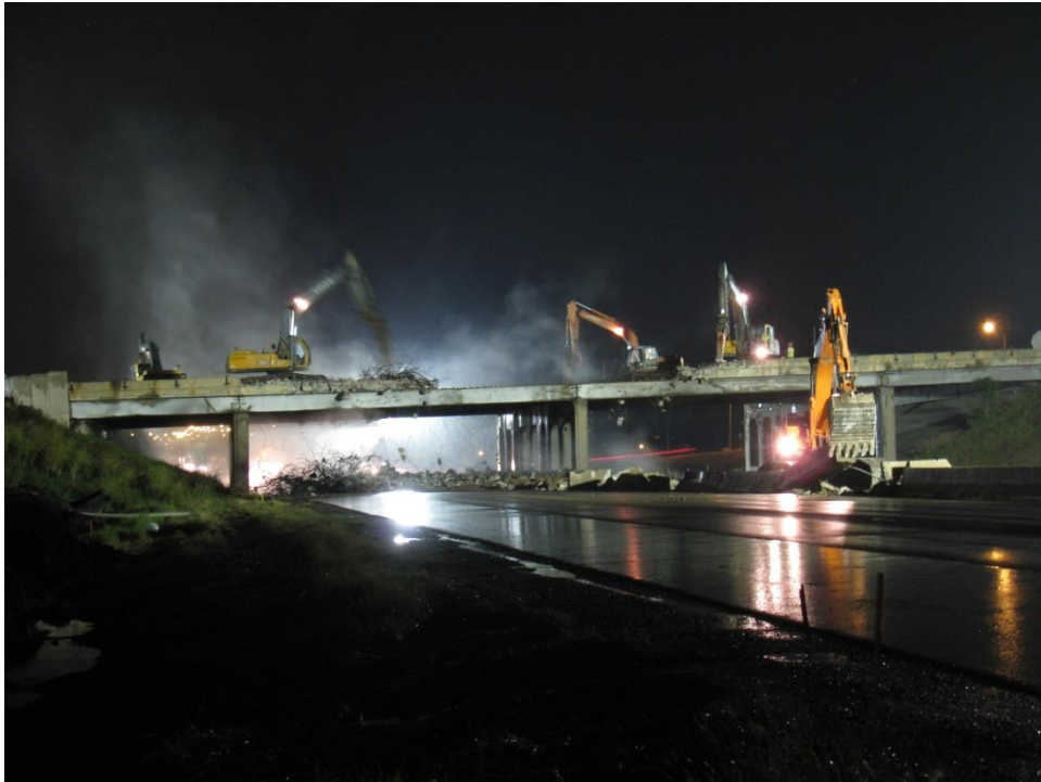
Figure 41. Photo. Demolishing Maryland Ave. bridge 6513 as seen from I-35E. The bridge was demolished over a weekend closure of I-35E, while traffic was diverted through the Maryland Ave. off- and on-ramps.
