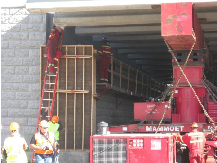
Figure 70. Photo. The vertical and horizontal positions of all girders of the span were carefully monitored from the abutment to ensure that it was lowered uniformly so as to not excessively stress the girders, deck, and pier columns, which could potentially cause cracking or other distresses.
