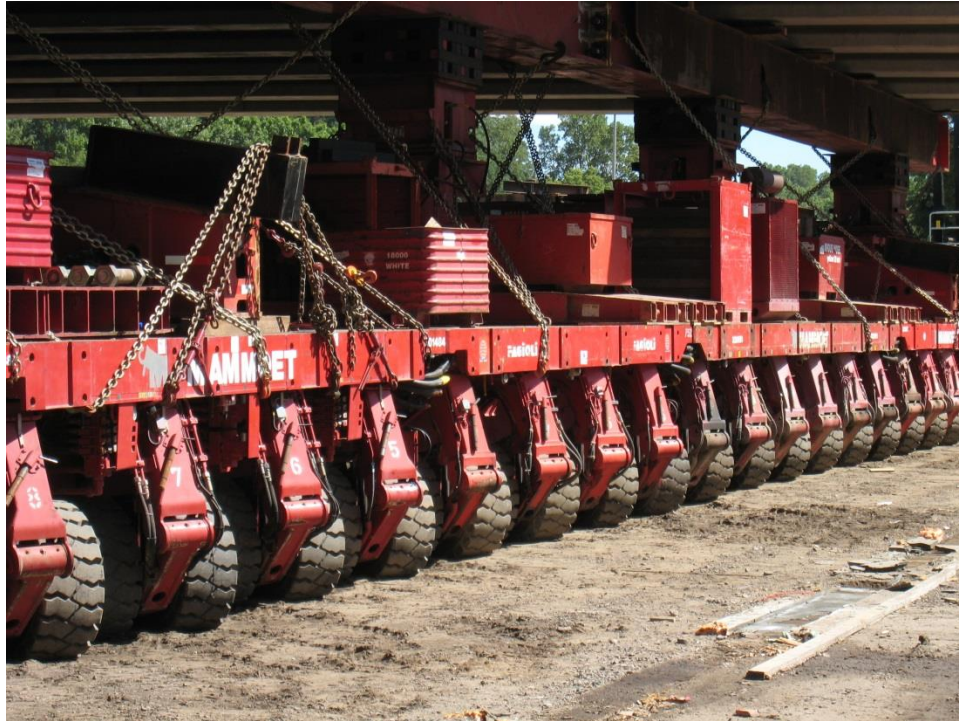
Figure 59. Photo. An SPMT is a computer-controlled platform vehicle with a large array of articulating wheels on the bottom. The SPMT used for this project had a total of 288 wheels on 2 sets of 18 axles.
