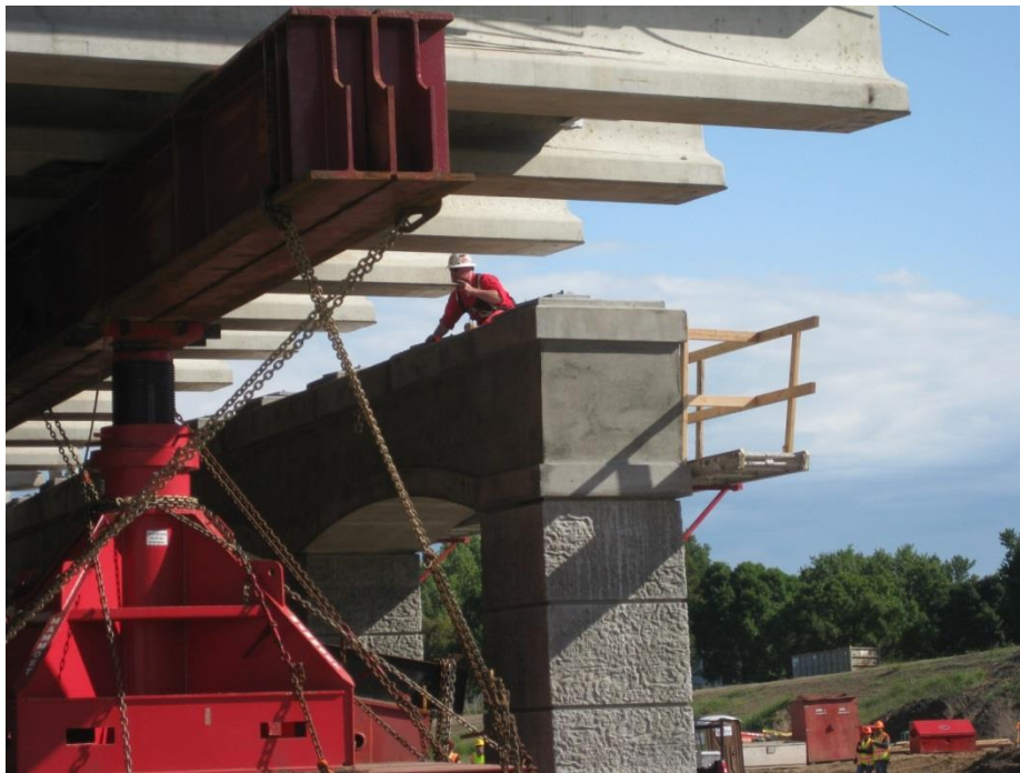
Figure 69. Photo. The vertical and horizontal positions of all girders of the span were carefully monitored from the pier to ensure that it was lowered uniformly so as to not excessively stress the girders, deck, and pier columns, which could potentially cause cracking or other distresses.
