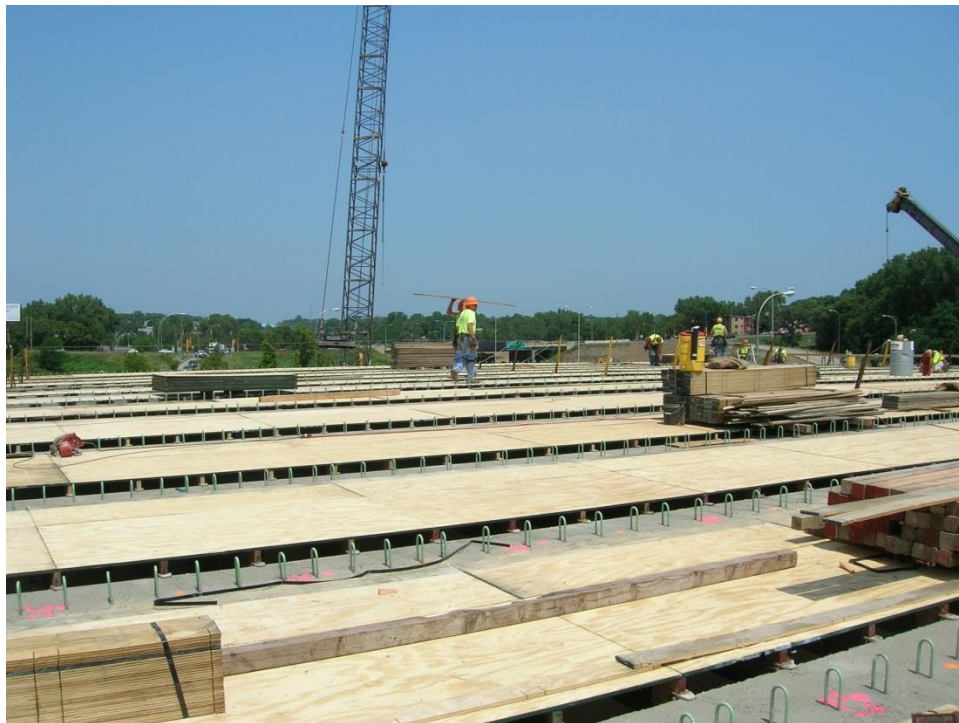
Figure 26. Photo. Placing the wooden forms for the deck concrete.
