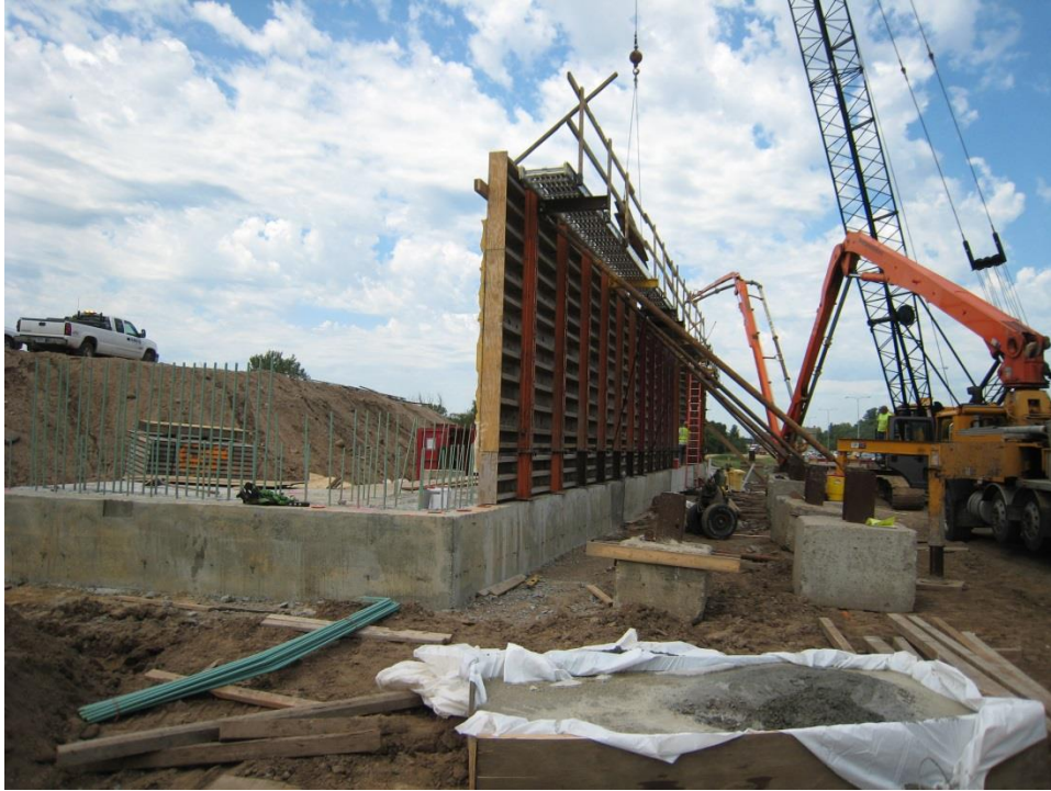
Figure 50. Photo. Close-up view of the construction of the west abutment.
