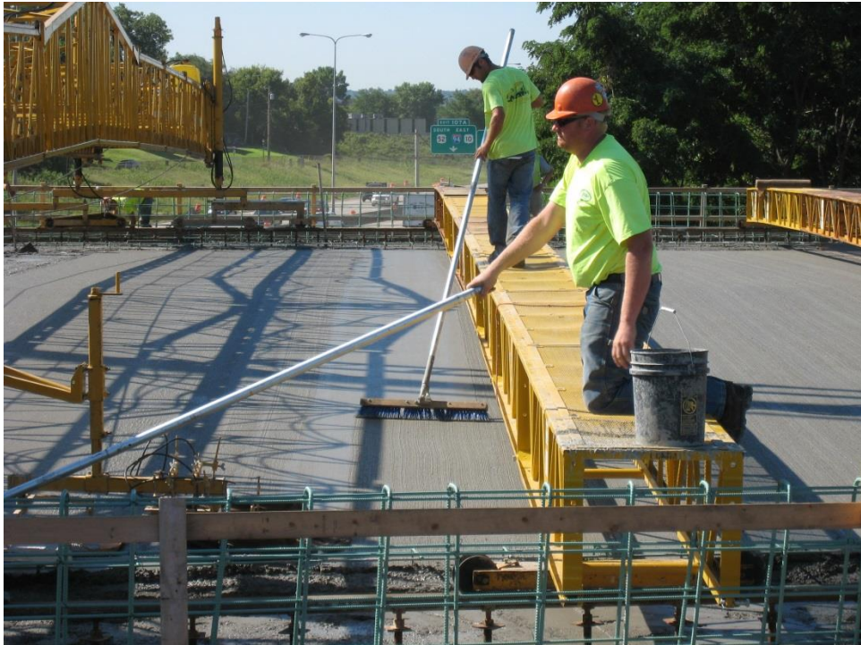
Figure 34. Photo. Finishing the bridge deck concrete surface from the finishing platform.
