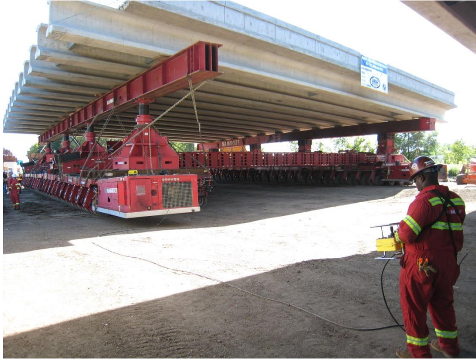
Figure 62. Photo. The SPMT movement was controlled by a single joystick operator who was in radio communications with strategically positioned personnel who provided directions and feedback.
