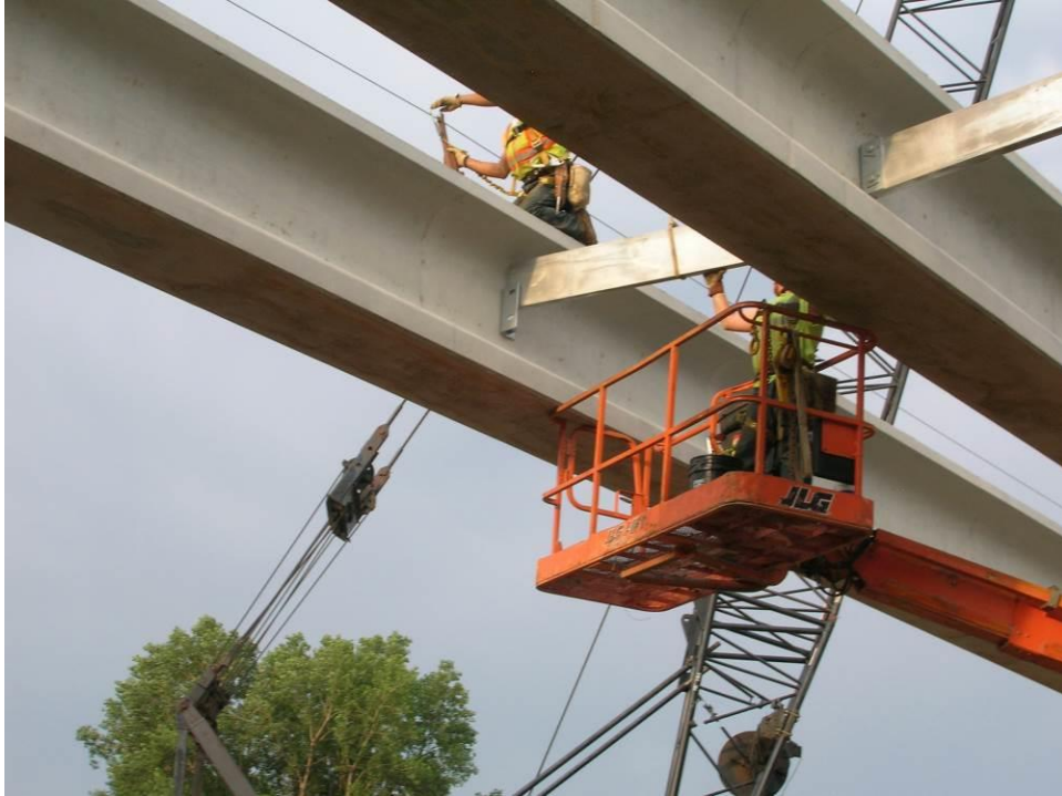
Figure 21. Photo. Bracing the girders to each other using steel braces.
