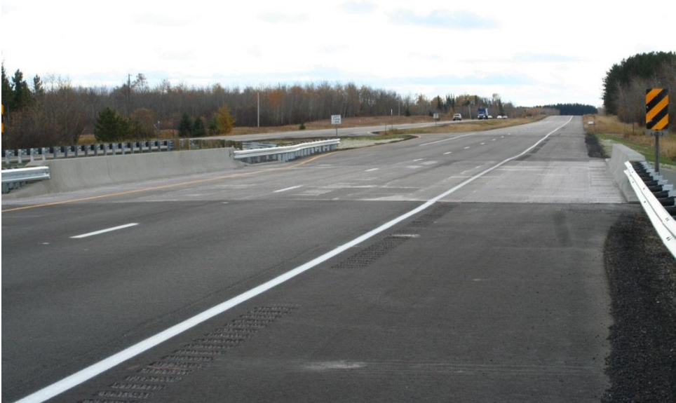
Figure 70. Overview of bridge 69071 after completion.
