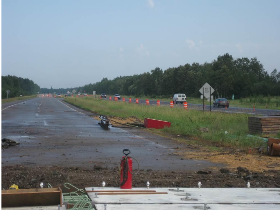
Figure 72. Closed Southbound Lanes.
