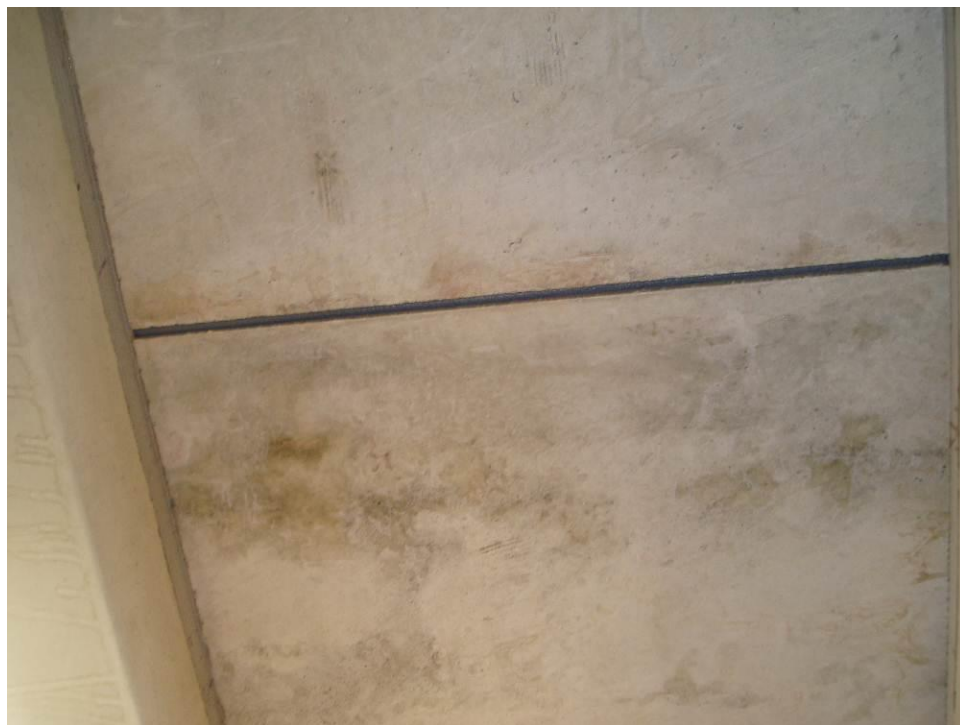
Figure 41. View of the backer rods from beneath the deck panels.
