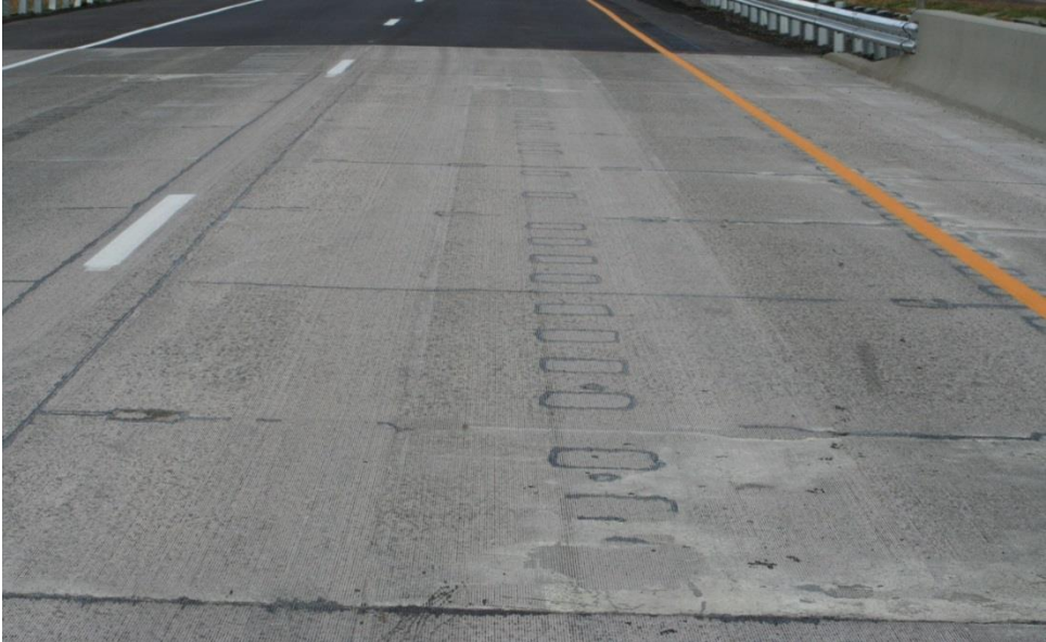
Figure 71. Close-up view of bridge 69071 deck surface after completion.
