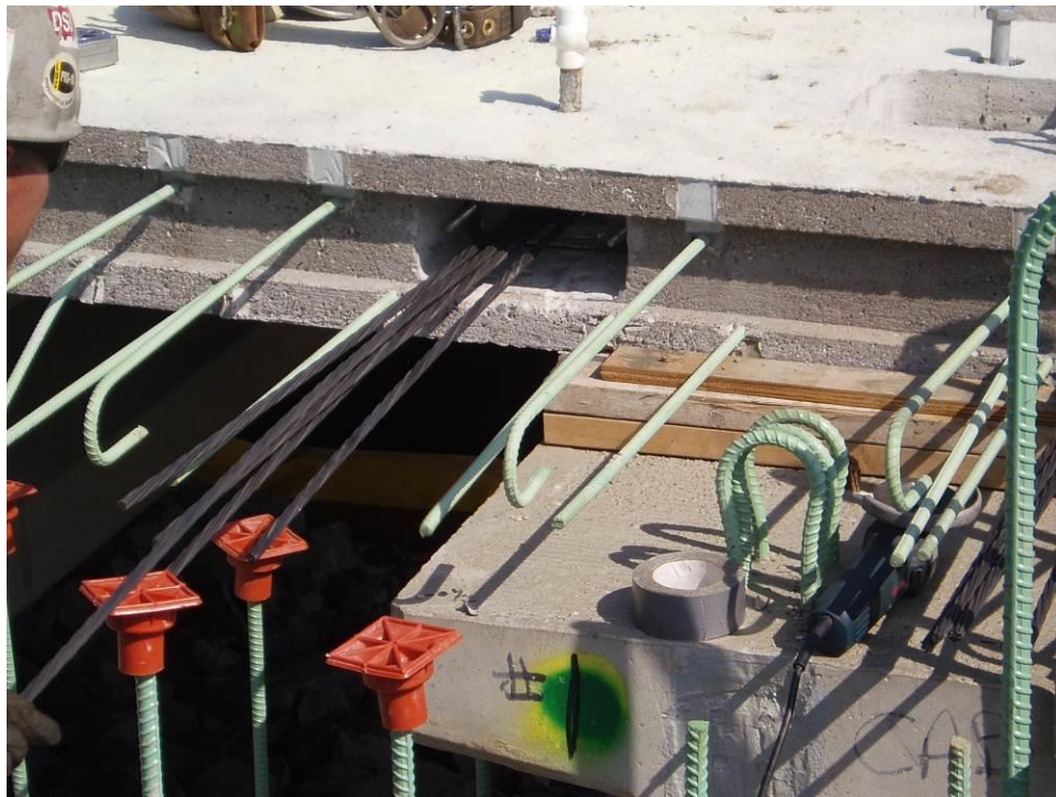
Figure 59. Four post-tensioning steel strands were installed through each duct.
