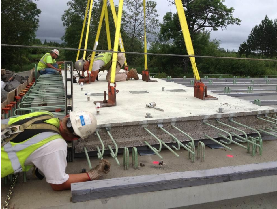
Figure 30. Aligning the deck panel and ensuring proper horizontal placement.
