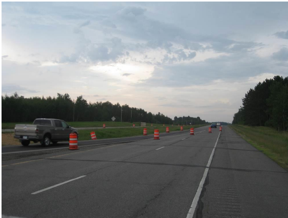
Figure 75. Taper and south bypass due to closure of the southbound lanes.
