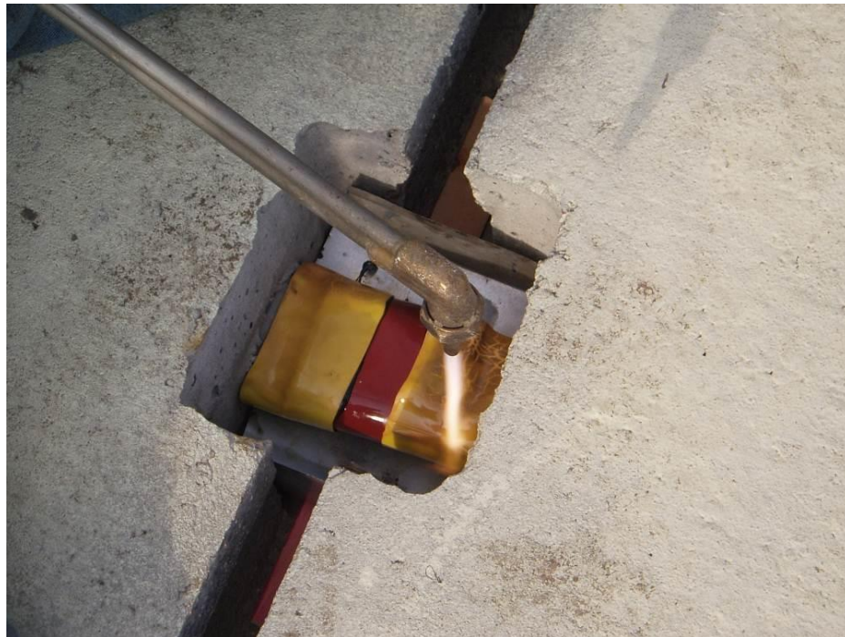
Figure 43. Corrugated plastic ducts that hold the post-tensioning cables.
