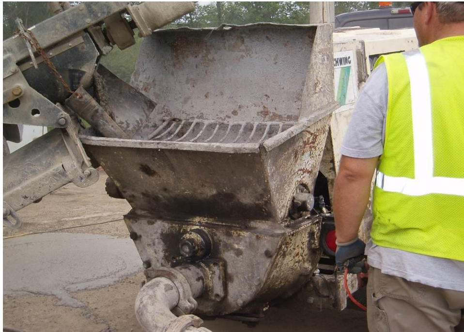
Figure 67. Mixing the grout for the haunches and the shear pocket blockouts.
