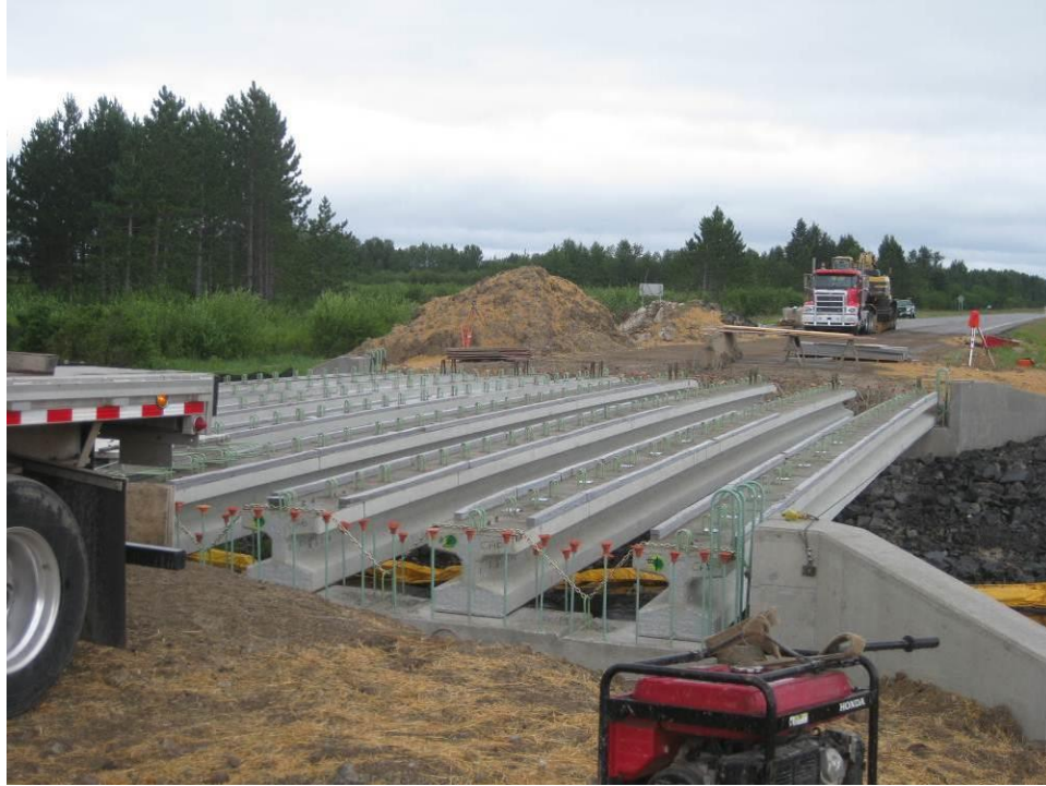
Figure 19. Girders for bridge 69071 prepared for placement of deck panels.
