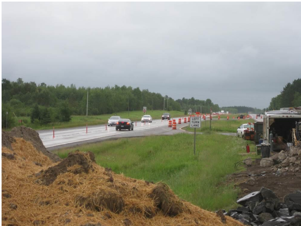
Figure 73. Traffic diverted to the northbound lanes from southbound lanes.
