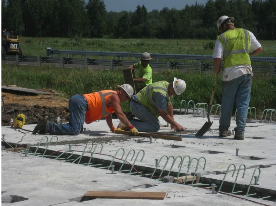
Figure 54. Floating the placed grout to remove excess material.
