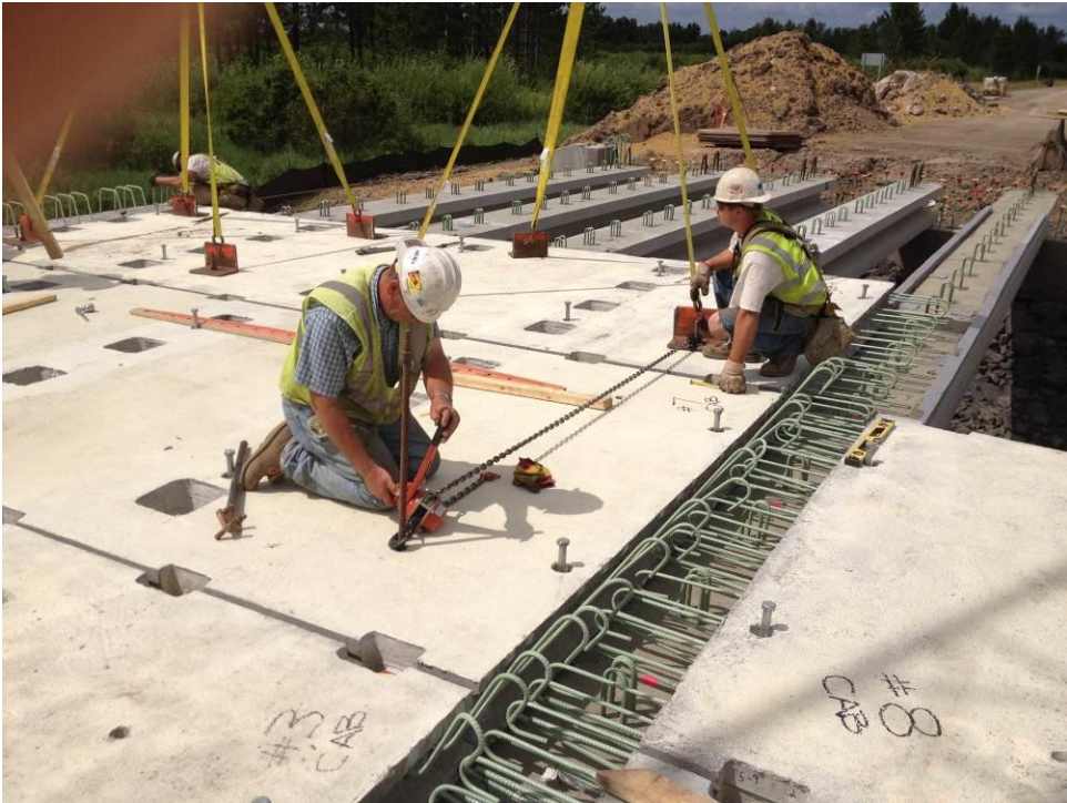
Figure 35. Positioning deck panels into place using the placed deck panels.
