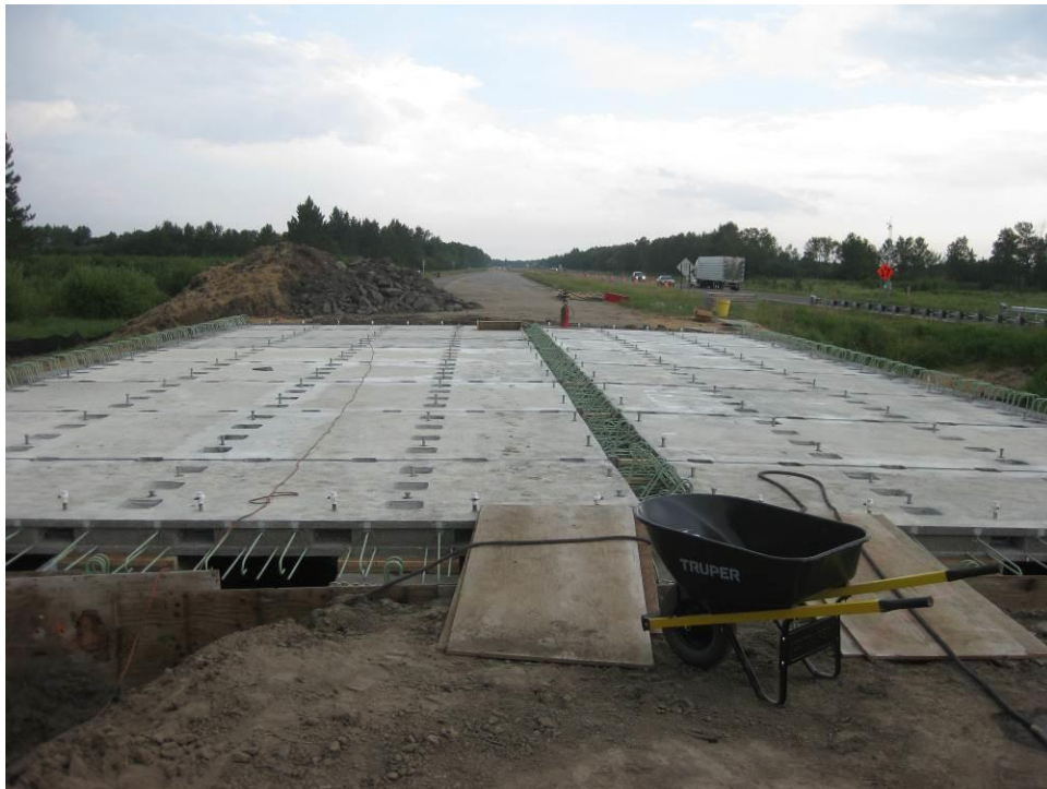
Figure 37. View of bridge deck following placement of all deck panels.
