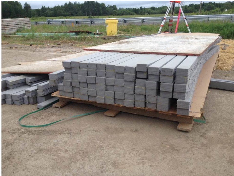
Figure 15. Haunch forming material for bridge 69071.
