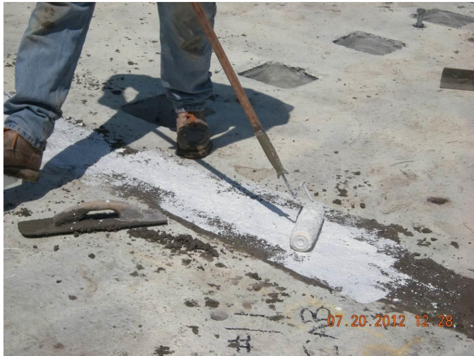
Figure 55. Applying curing compound to the grout to control shrinkage cracks.
