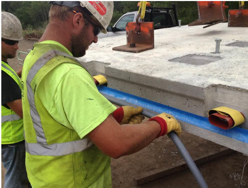
Figure 39. Installation of backer rod to form the joints between the panels.
