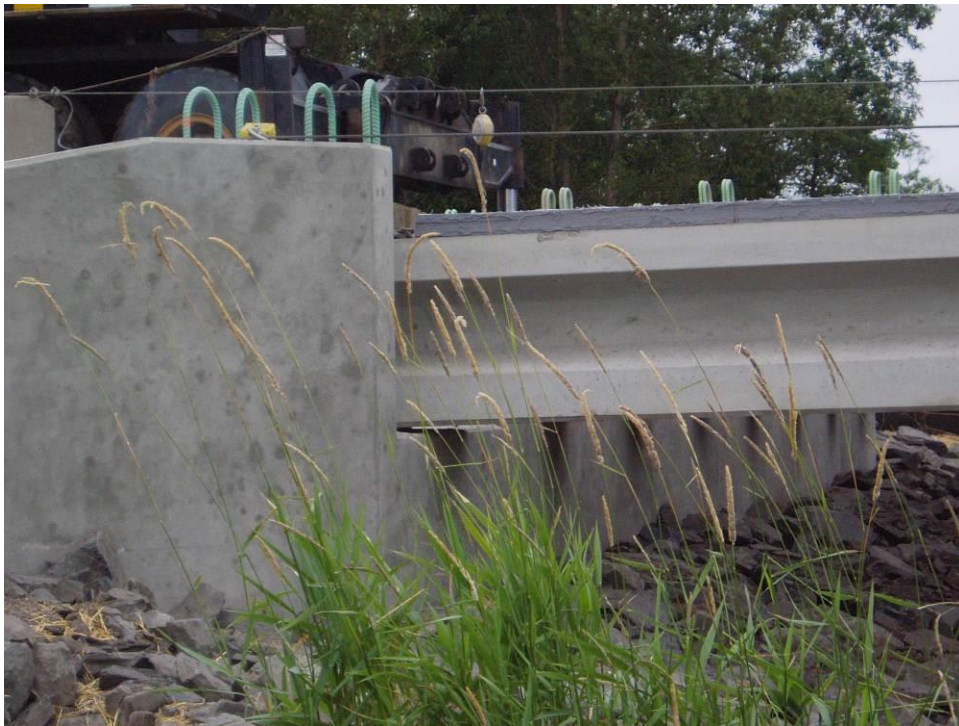
Figure 18. End girder placed on top of the abutment wall for bridge 69071.
