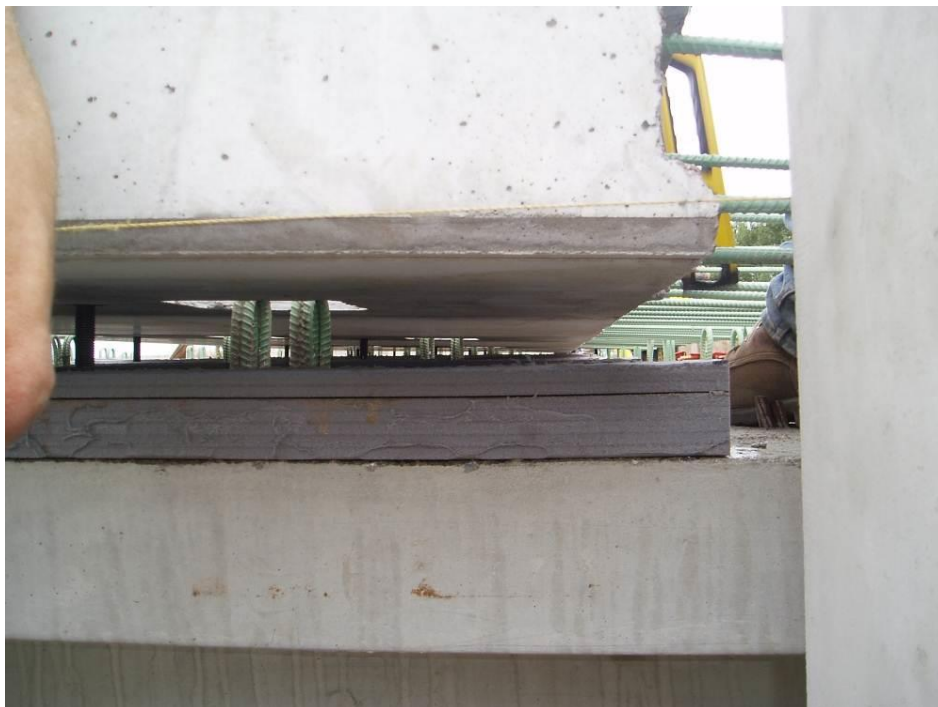
Figure 27. Placing the deck panel onto the haunch forming material.
