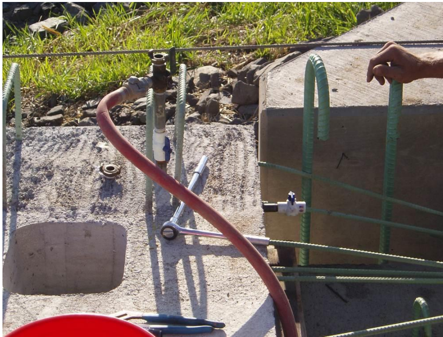
Figure 65. Pumping neat grout into the corrugated post-tensioning ducts.
