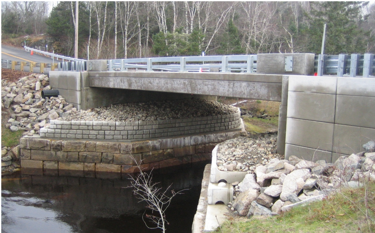
Figure 11. The completed Lamson Bridge Project.
