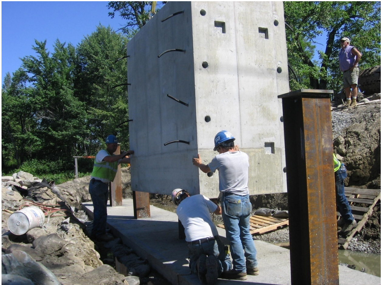
Figure 15. Installation of the precast bridge abutment.
