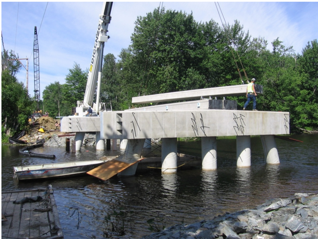
Figure 17. Placement of the superstructure beams.
