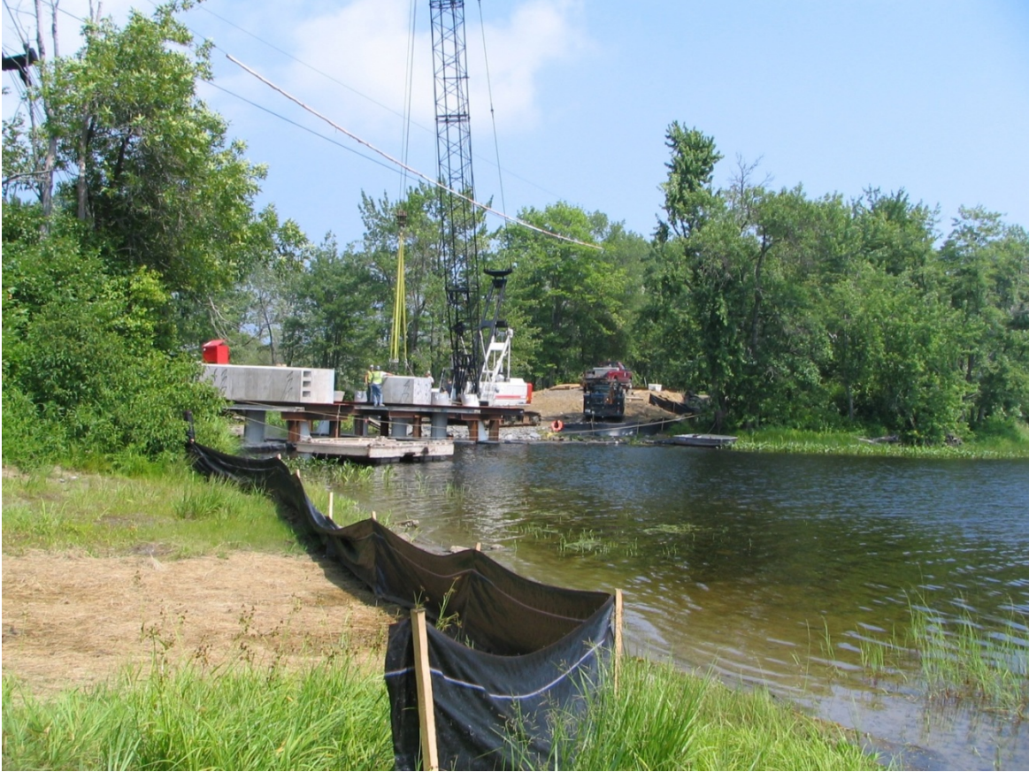
Figure 16. Installation of the precast post-tensioned pier caps.
