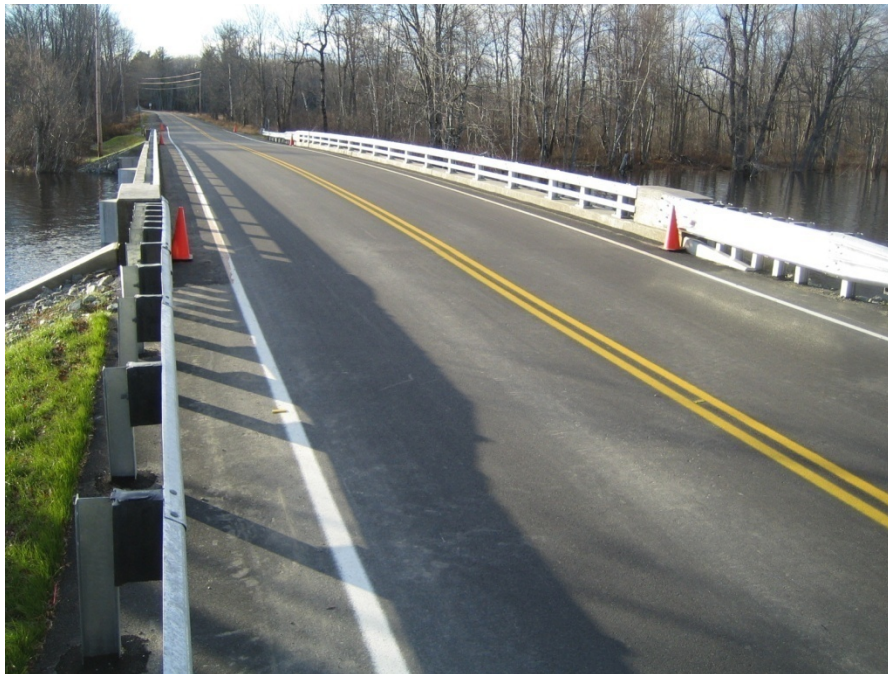
Figure 26. Boom Birch post-construction pavement.
