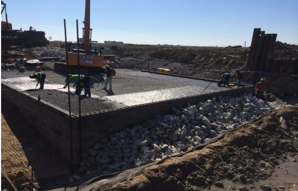
Figure 15. Photo. Installation of riprap (courtesy: LADOTD).
