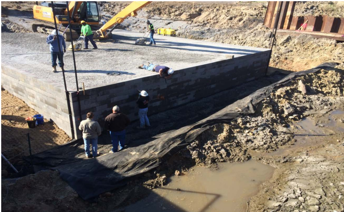
Figure 14. Photo. Installation of eleventh row of blocks (scour line) (courtesy: LADOTD).
