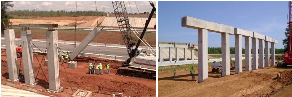
Figure 2. Placement of precast columns.
