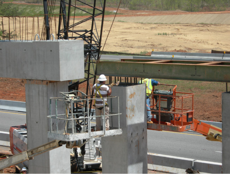
Figure 8. Workers check alignment of prefabricated columns with template.
