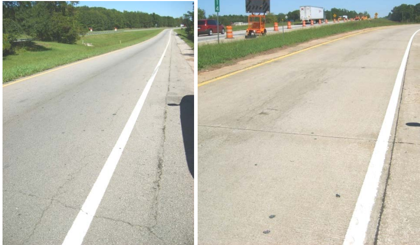
Figure 14. Comparison pavements (left to right): Exit 13 ramp and Exit 14 ramp.
