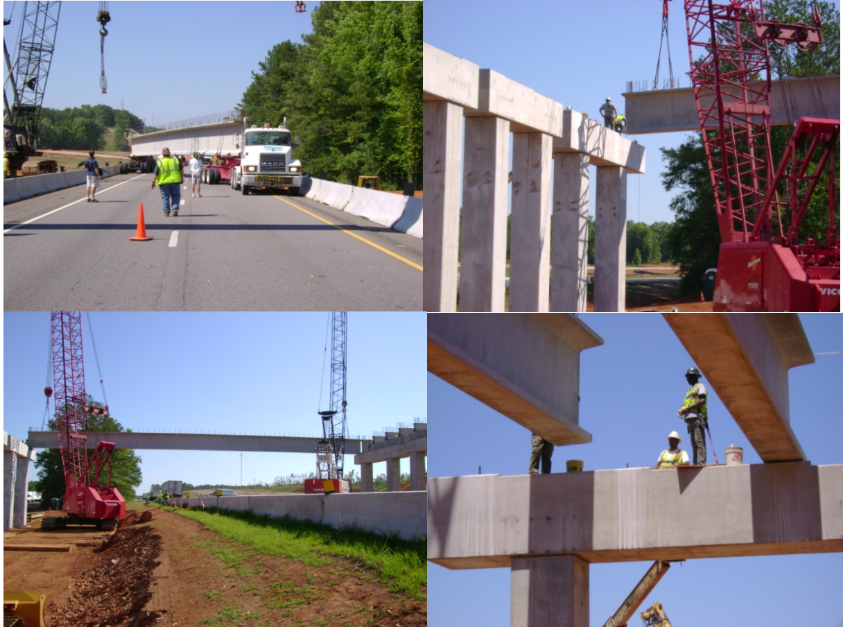
Figure 10. 130 ft long Prestressed “bulb-I” beam installation.
