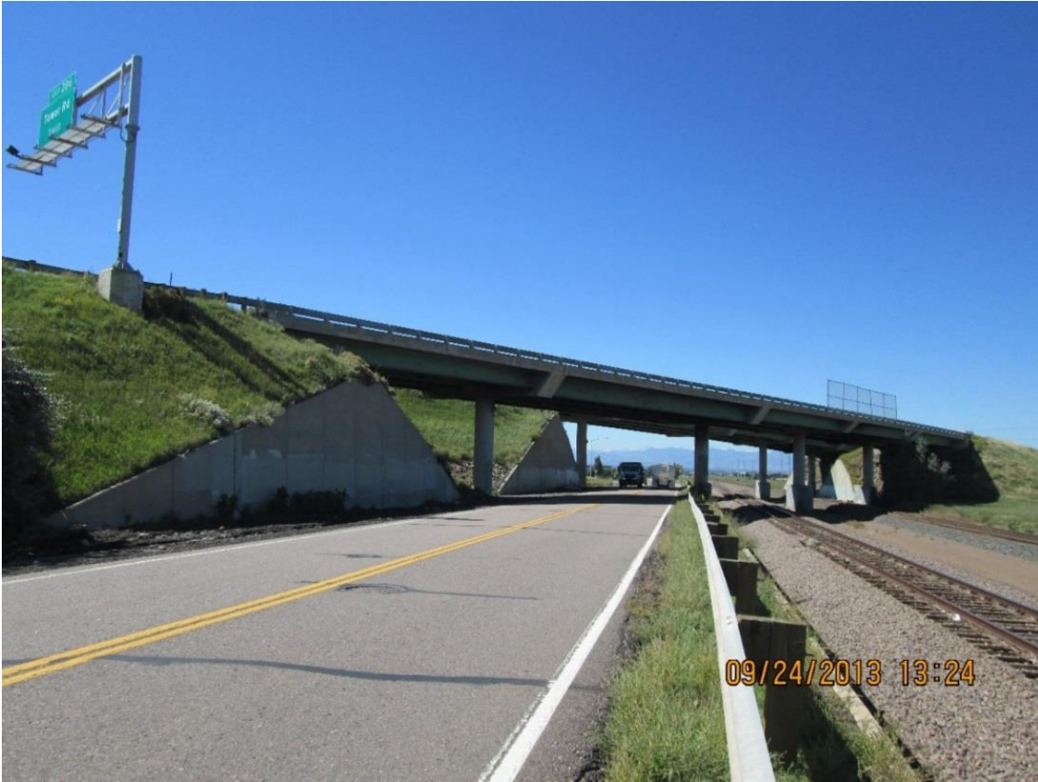
Figure 4. Photo. Bridge E-17-JX (westbound).
