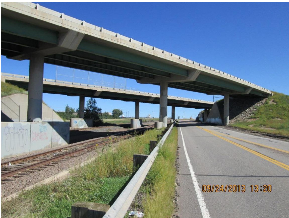
Figure 3. Photo. Bridge E-17-JW (eastbound).
