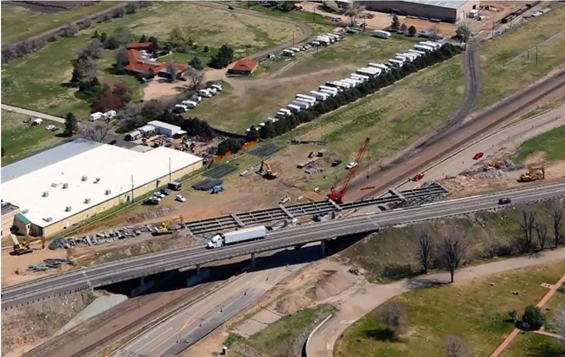
Figure 16. Photo. Steel girder installation for E-17-AEK.
