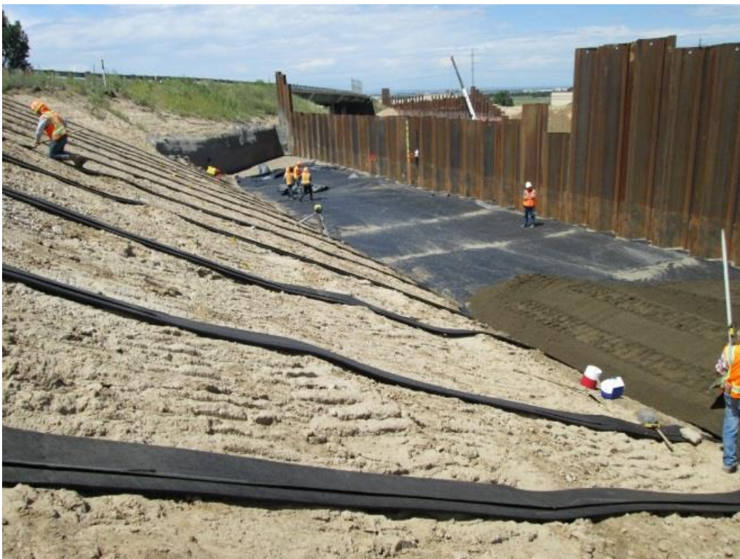
Figure 14. Photo. GRS-IBS construction of abutment 4, E-17-AEK: sheet piling wall E-17-DF shown.
