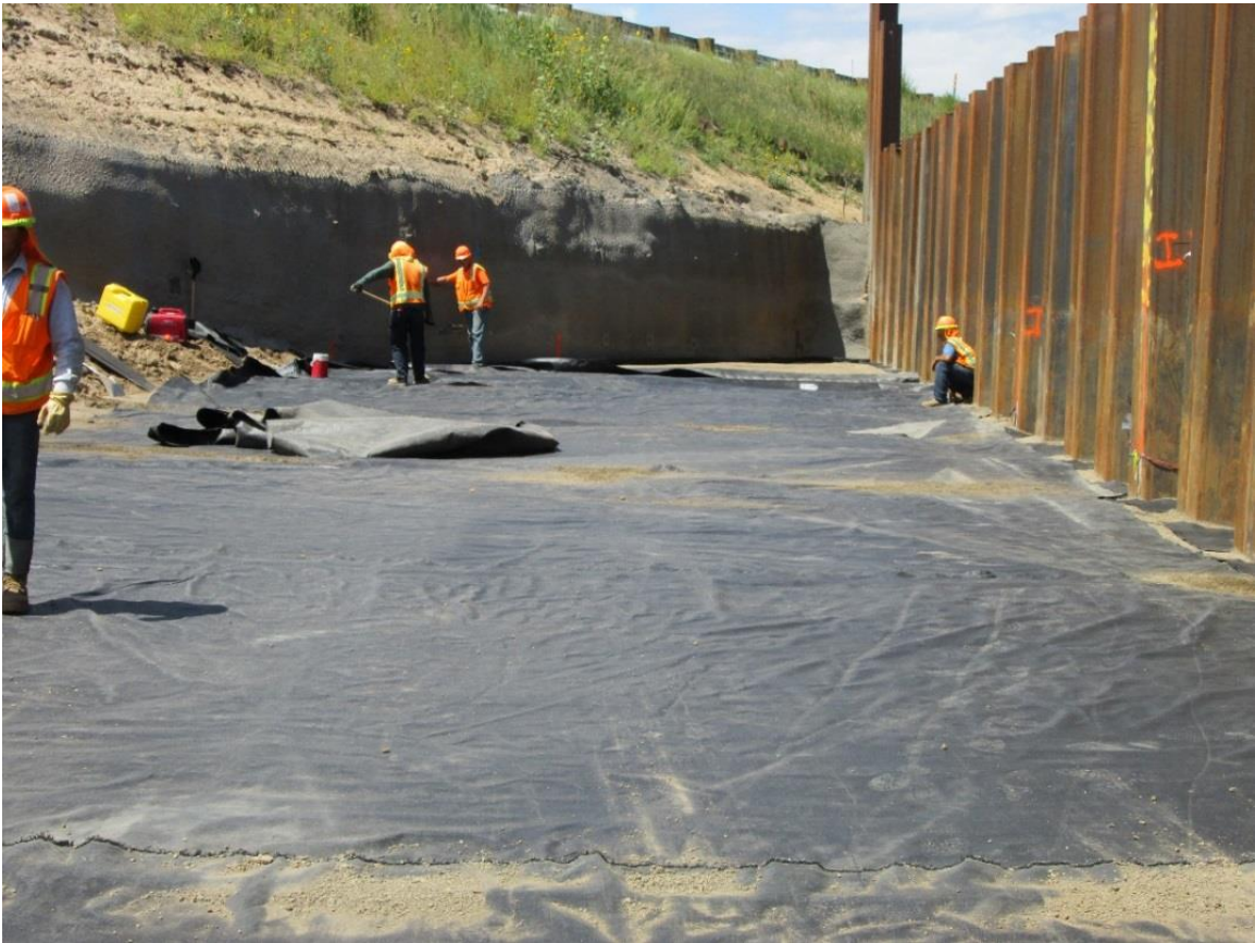
Figure 12. Photo. GRS-IBS construction of abutment 4, E-17-AEK: placement of geosynthetic fabric.
