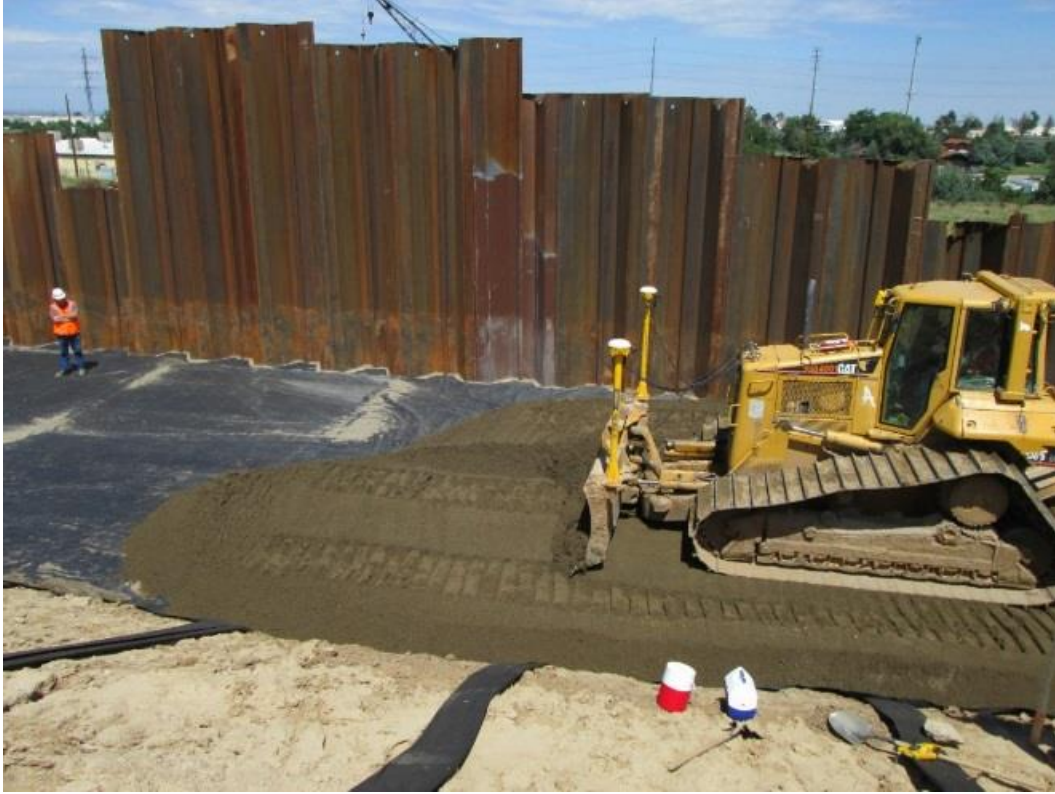
Figure 15. Photo. GRS-IBS construction of abutment 4, E-17-AEK (close-up view).
