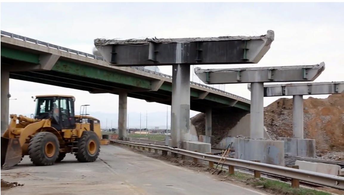
Figure 11. Photo. Old westbound structure, E-17-JX, being demolished.
