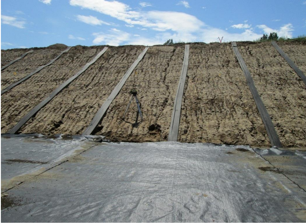
Figure 13. Photo. GRS-IBS construction of abutment 4, E-17-AEK.
