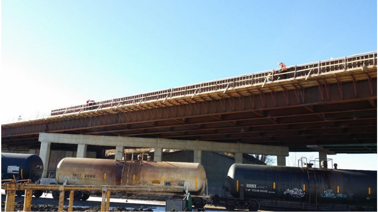
Figure 17. Photo. New bridge E-17-AEK, March 2015, facing abutment 4.
