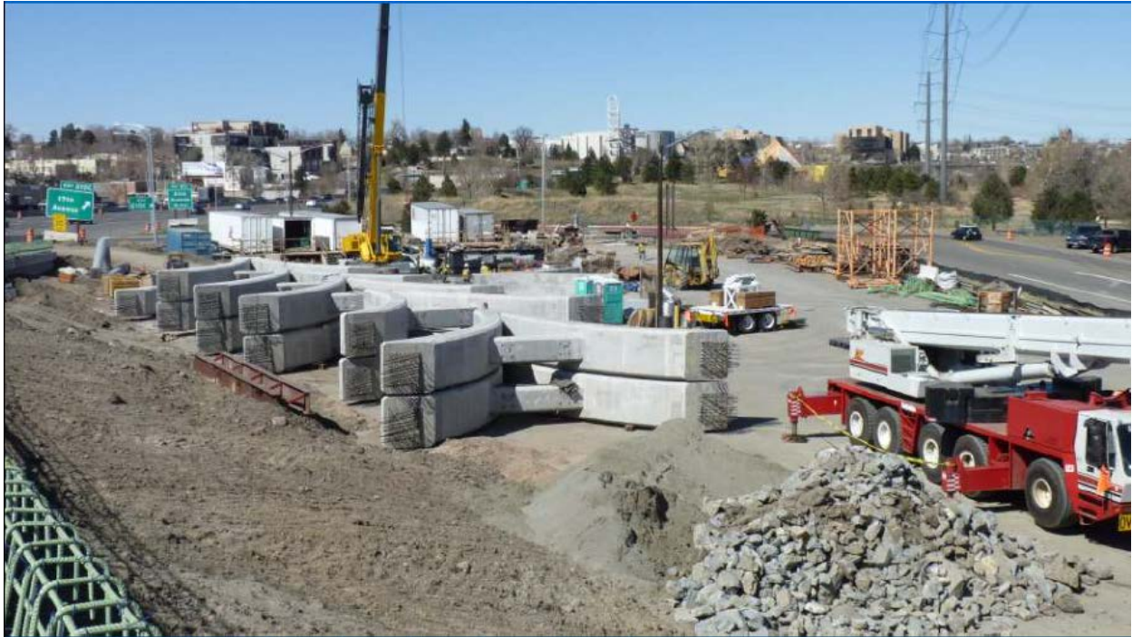
Figure 21. Photo. Prefabricated piers stacked in adjacent yard (courtesy: Colorado DOT).
