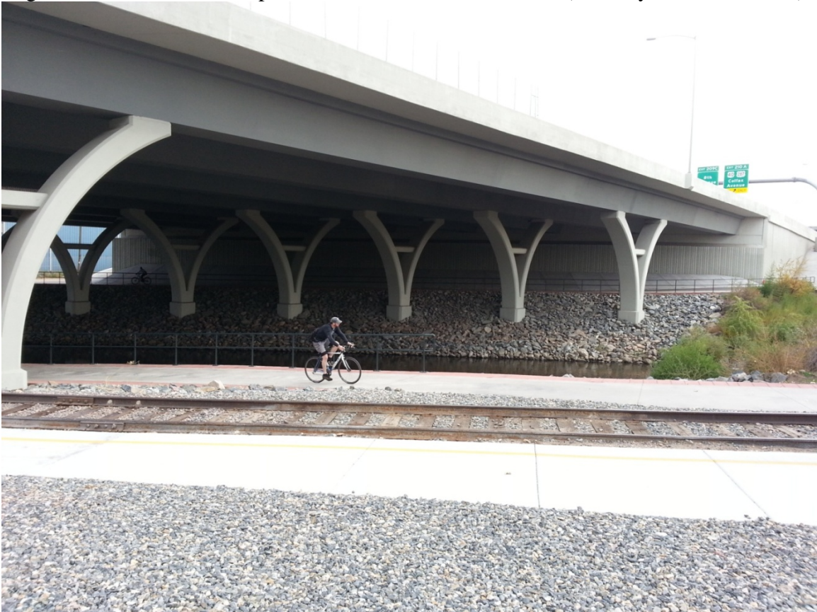
Figure 27. Photo. Photograph of completed structure (courtesy: Colorado DOT).
