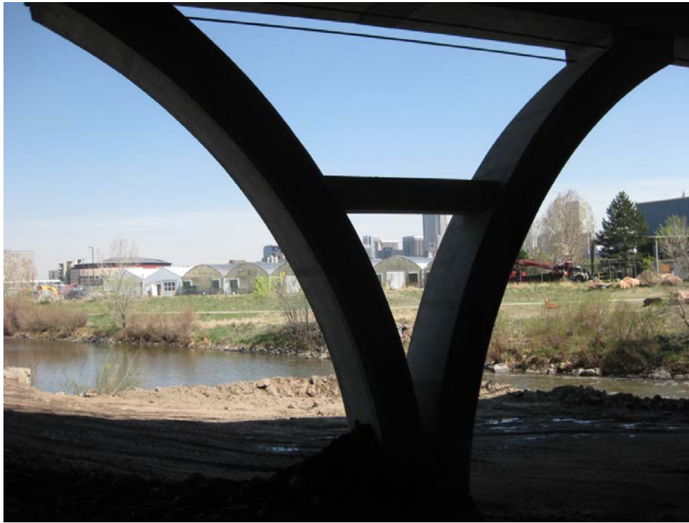
Figure 15. Photo. Arch shaft pier (courtesy: Colorado DOT).
