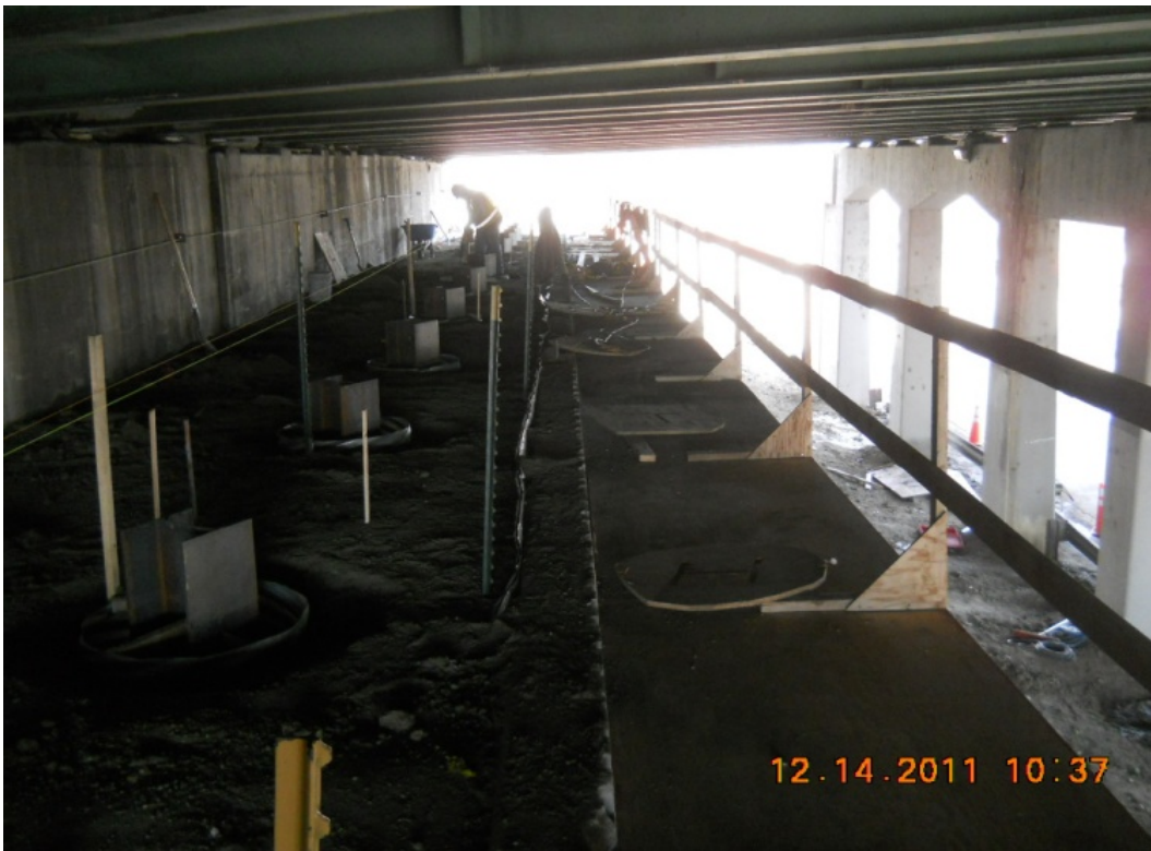
Figure 19. Photo. Walls backfilled and compacted around piling (courtesy: Colorado DOT).
