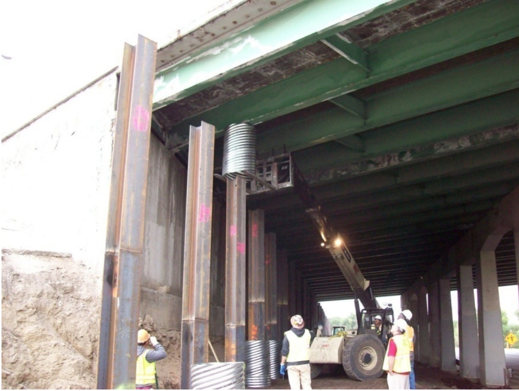
Figure 18. Photo. Piling for new bridge abutment (courtesy: Colorado DOT).
