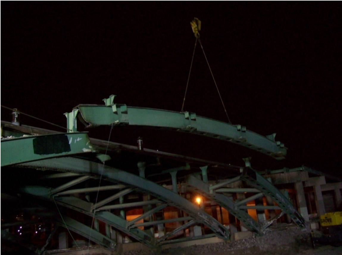
Figure 20. Photo. Center portion of the original steel arch being removed (courtesy: Colorado DOT).
