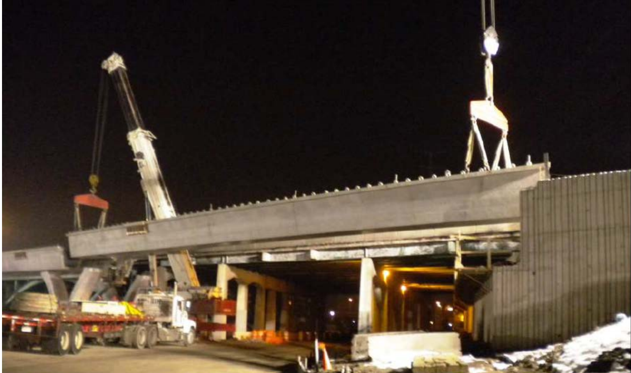
Figure 23. Photo. U72 girder being set in place (courtesy: Colorado DOT).
