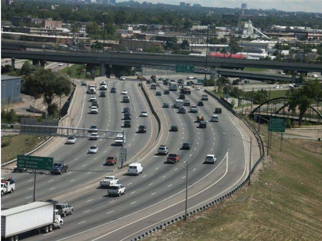
Figure 3. Photo. Four lanes and entry/exit ramp in each direction (courtesy: Colorado DOT).
