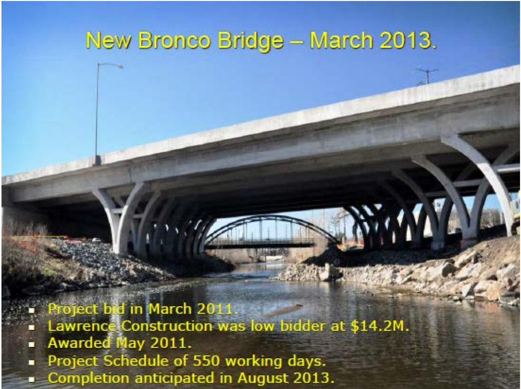
Figure 6. Photo. Elevation view of new structure (courtesy: Colorado DOT).
