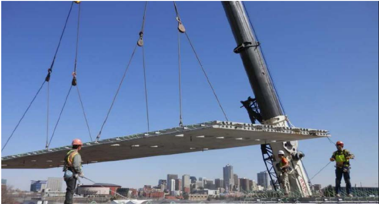
Figure 24. Photo. Placement of deck panels (courtesy: Colorado DOT).
