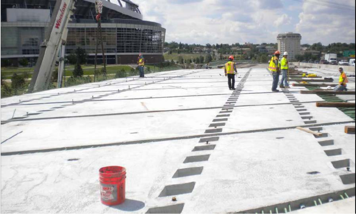
Figure 26. Photo. Panels in place from abutment to abutment (courtesy: Colorado DOT).
