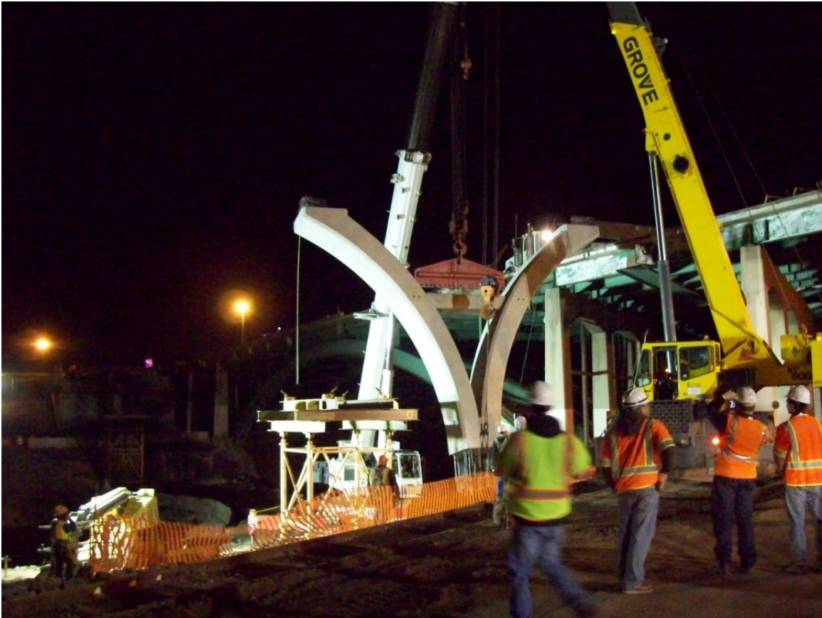
Figure 22. Photo. Pier being set on footing (courtesy: Colorado DOT).
