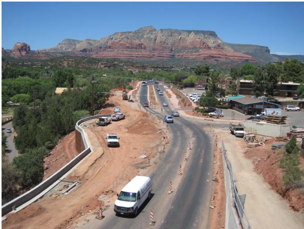
Figure 8. Half-and-half construction of roundabouts.
