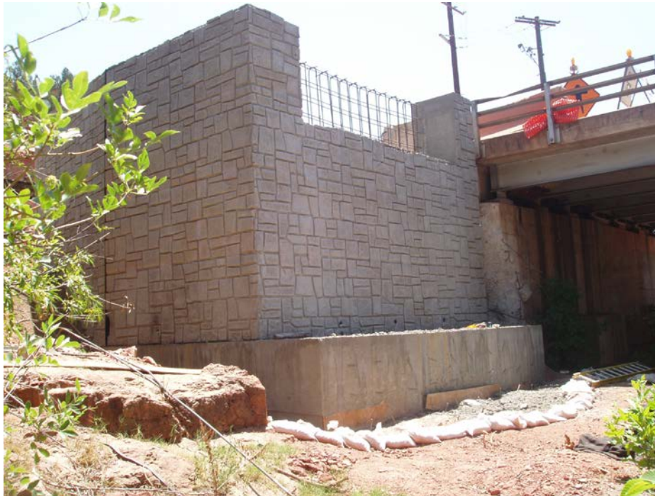
Figure 16. Front view of the pedestrian bridge abutment.
