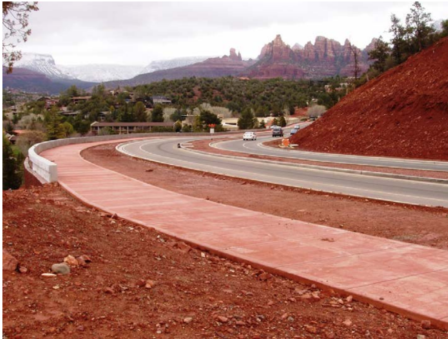
Figure 10. View of reconstructed SR 179 looking north.
