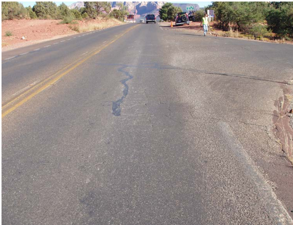
Figure 3. Existing SR 179 looking north at Meadowlark Drive.
