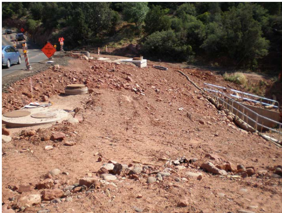
Figure 15. Stormceptors after installation at Morgan Wash.
