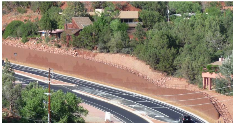
Figure 12. L-walls minimized right-of-way impacts.
