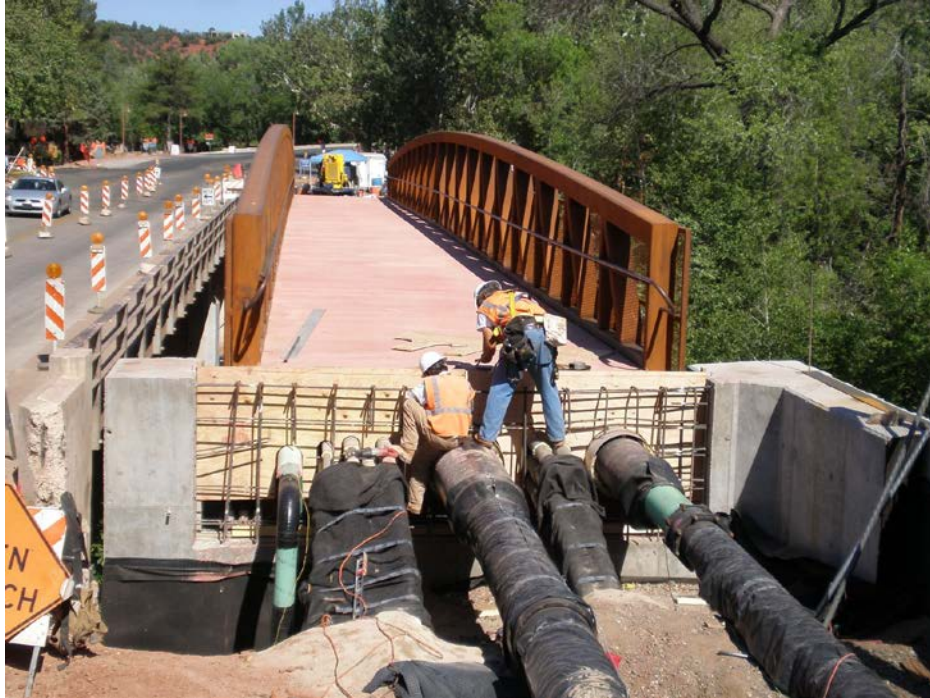
Figure 17. The utilities and the prefabricated pedestrian bridge.
