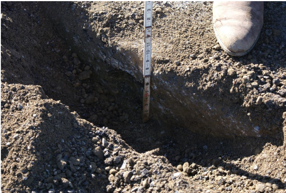
Figure 8. Photo. Target depth of reclamation process after initial milling.
