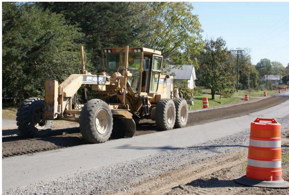
Figure 10. Photo. Using motor grader to level milled surface.
