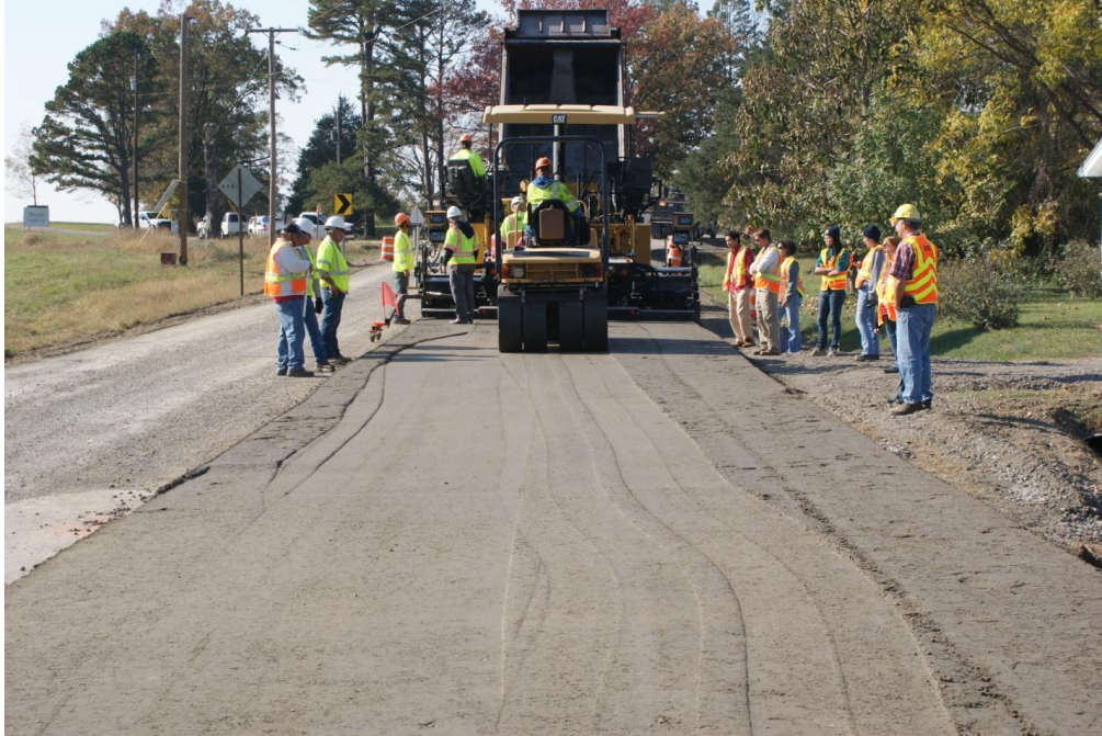
Figure 17. Photo. Initial light roller. Note rubber tire marks resulting in excessive roughness.
