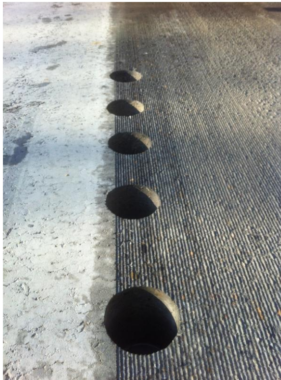
Figure 25. Photo. Diamond ground surface at core sample locations (courtesy University of Arkansas).
