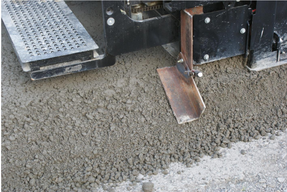
Figure 21. Photo. Adjustable jig used to create safety edge behind paver.
