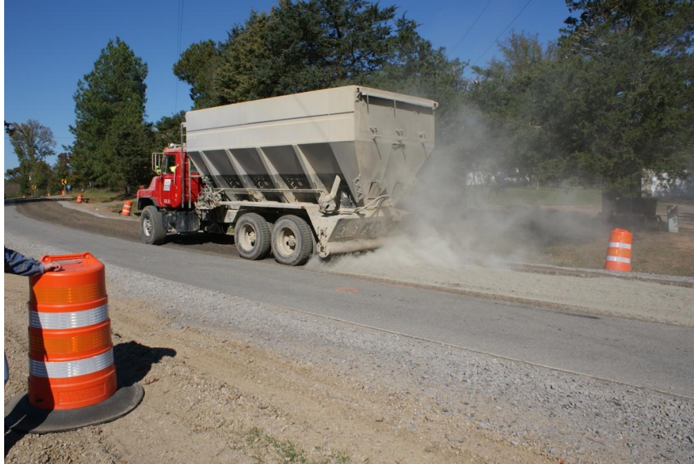
Figure 9. Photo. Application of cement to milled surface.
