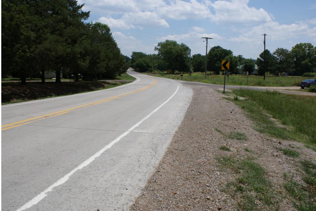
Figure 23. Photo. Completed safety edge after project completion.
