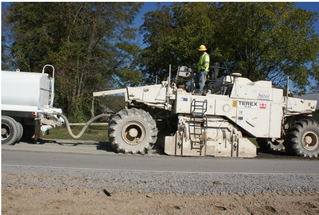
Figure 12. Photo. Side view of water truck coupled to reclamation unit.
