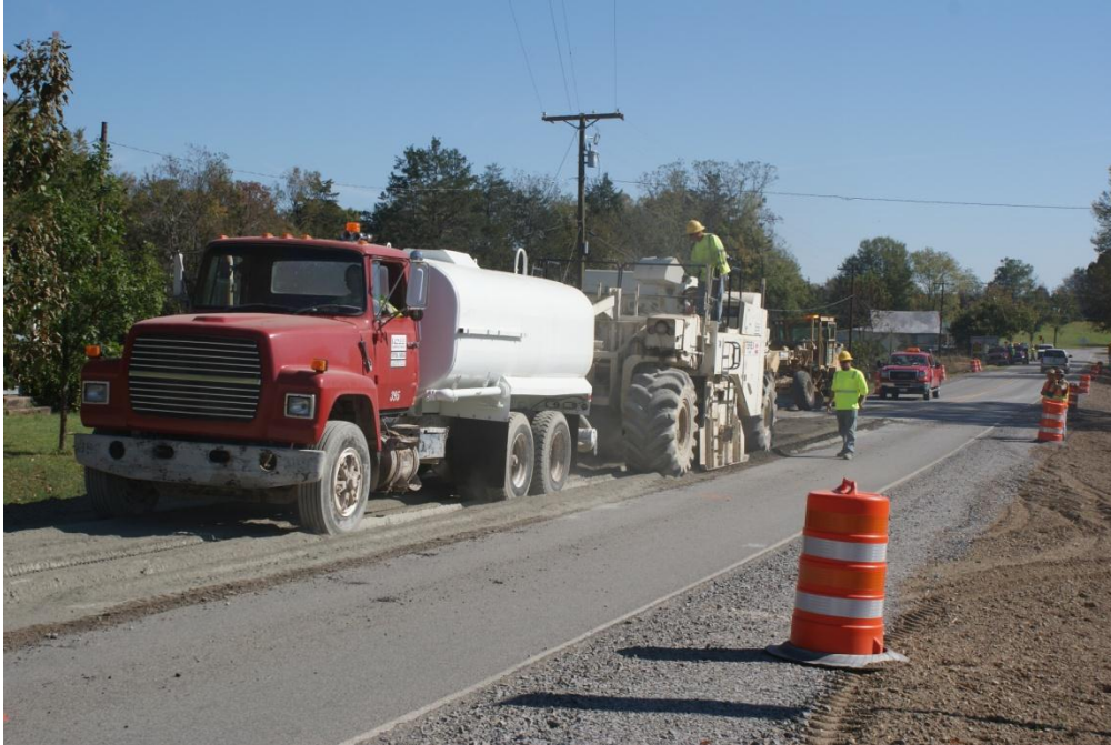
Figure 11. Photo. Water truck coupled to reclamation/stabilization unit.
