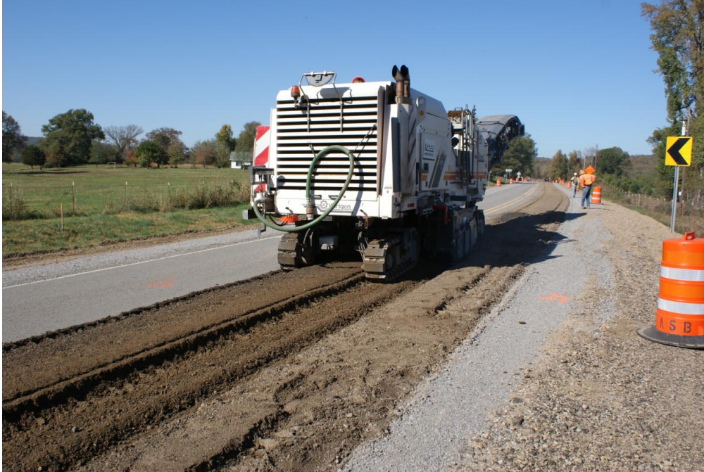
Figure 7. Photo. Milling machine on second pass of reclamation process.
