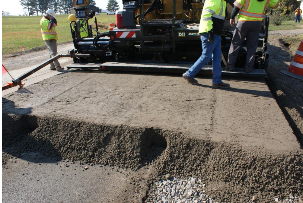
Figure 16. Photo. RCC construction behind paver.
