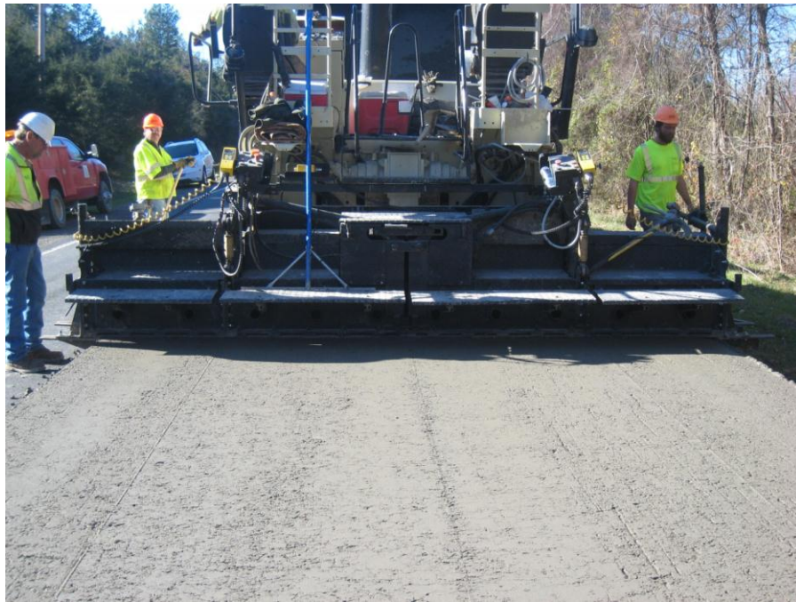
Figure 19. Photo. RCC surface immediately behind paver (courtesy University of Arkansas).
