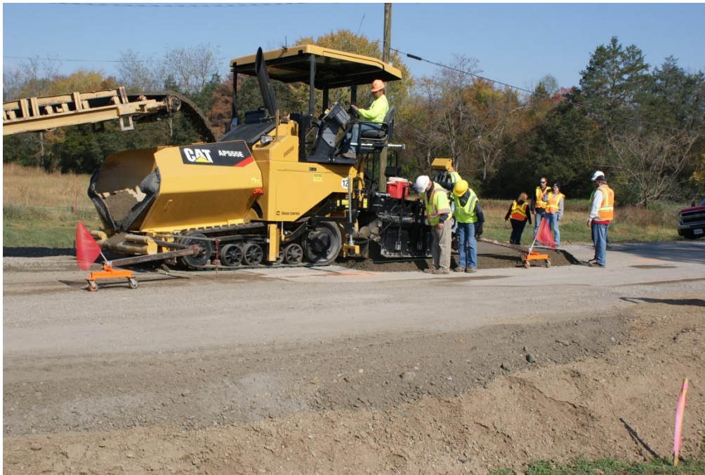
Figure 15. Photo. Placement of RCC using traditional AC paver.
