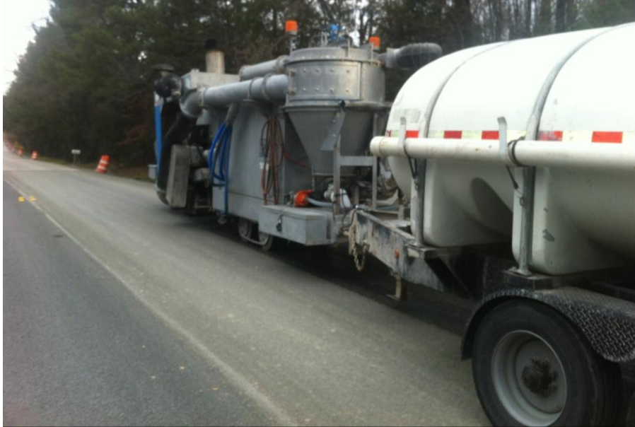
Figure 24. Photo. Traditional diamond grinding operation (courtesy University of Arkansas).
