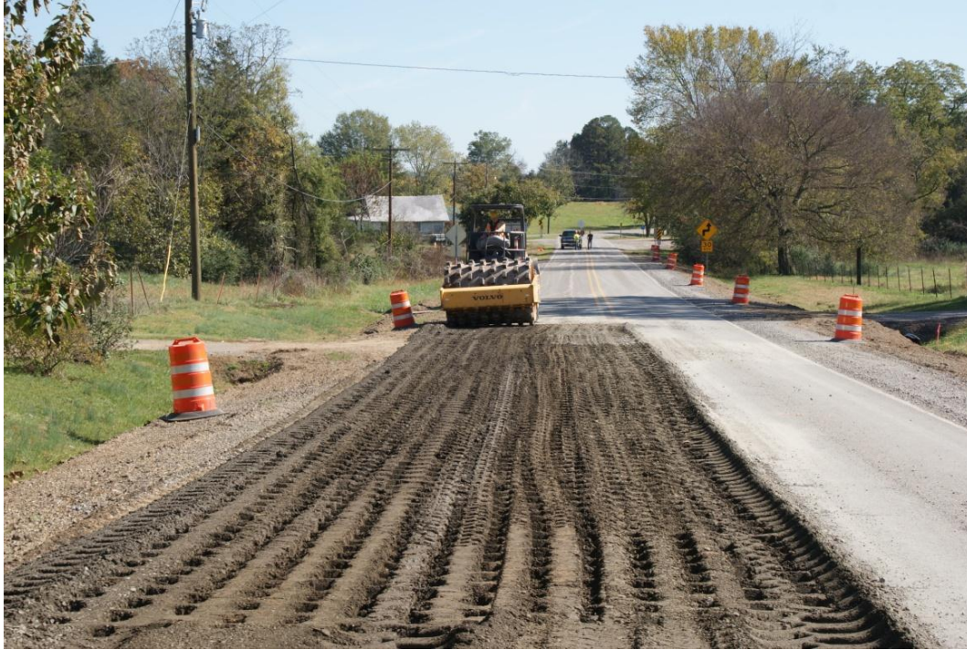
Figure 13. Photo. Cement stabilized material during compaction process.
