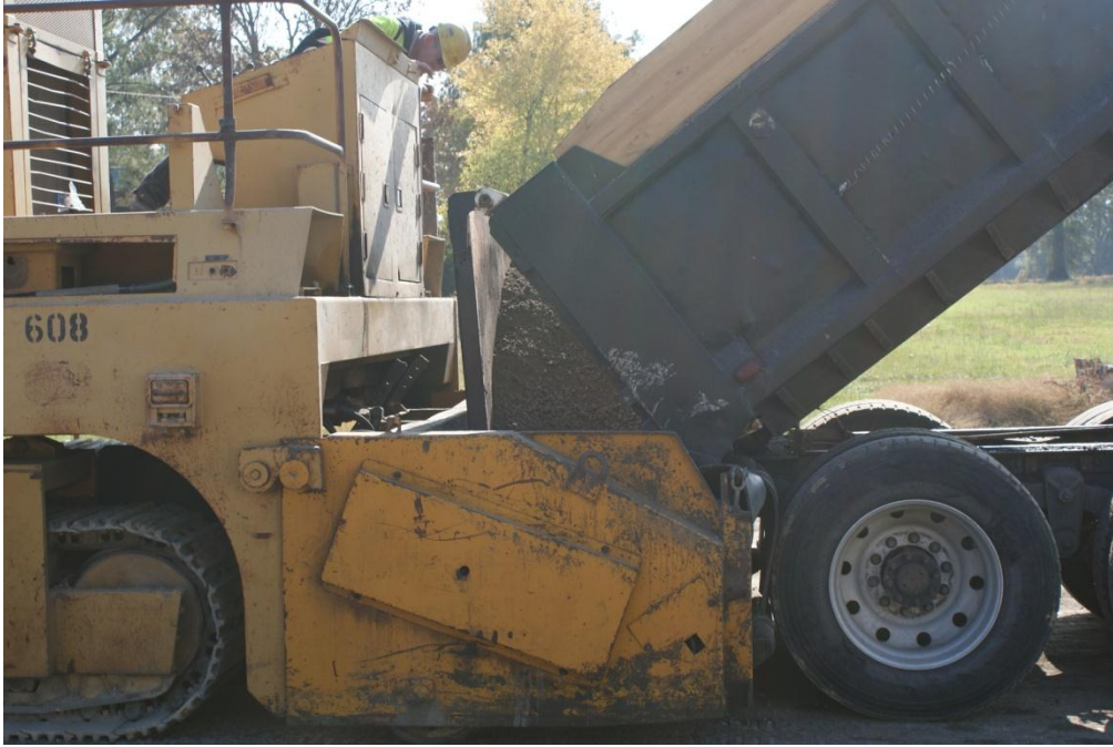
Figure 14. Photo. RCC mix emptied into transfer vehicle.
