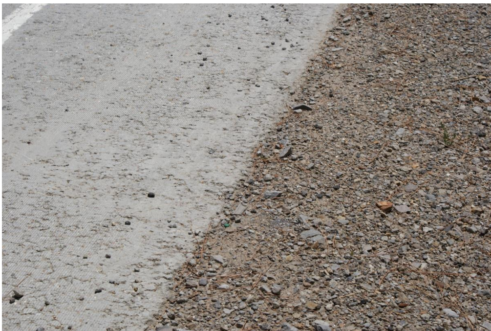
Figure 22. Photo. Close-up of completed safety edge.
