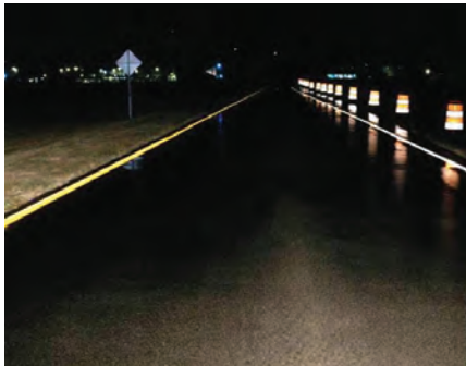
All-Weather Pavement Markings
