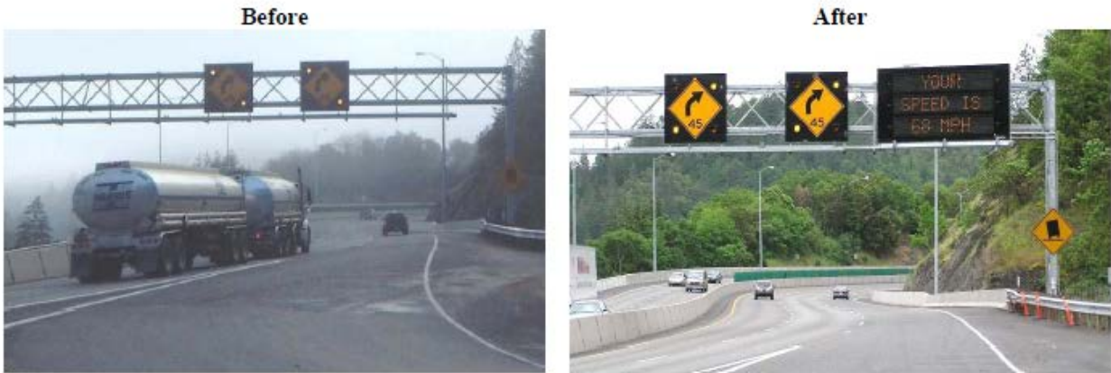
Figure 2. Photo. Southbound Interstate 5 DSFS systems in Oregon. (22)
