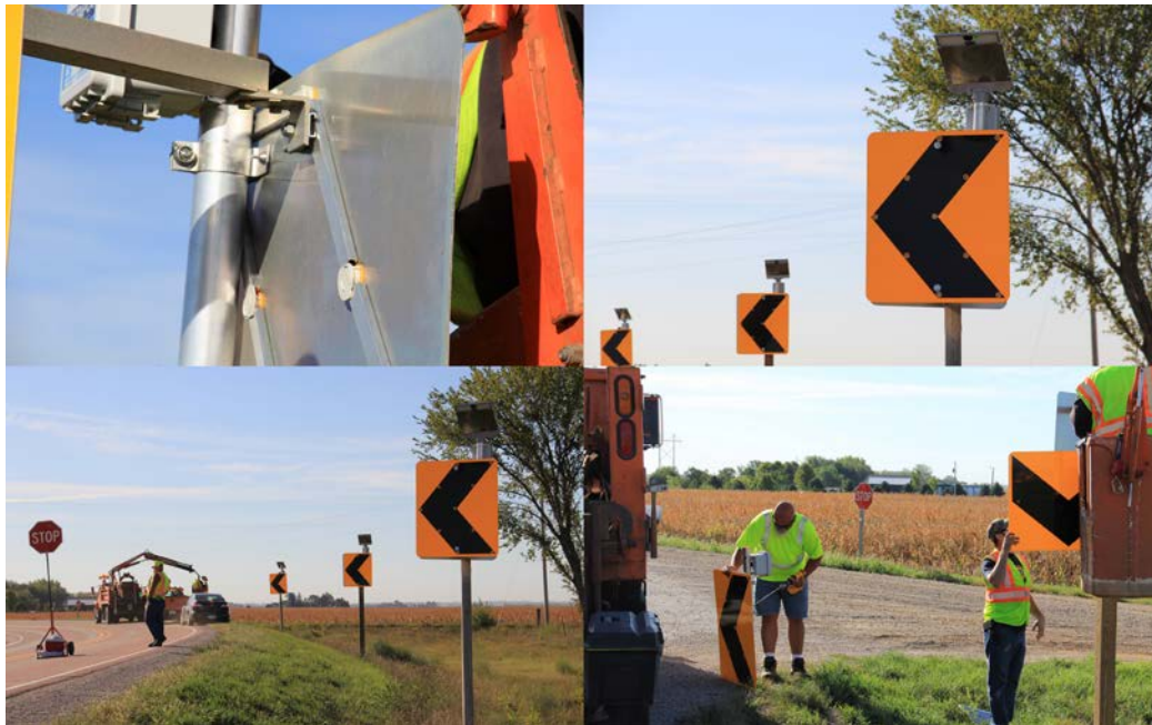
Figure 13. Photos. Installation of the SDCWS.
