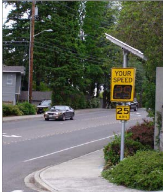
Figure 4. Photo. DSFS system in Bellevue, Washington. (24)
