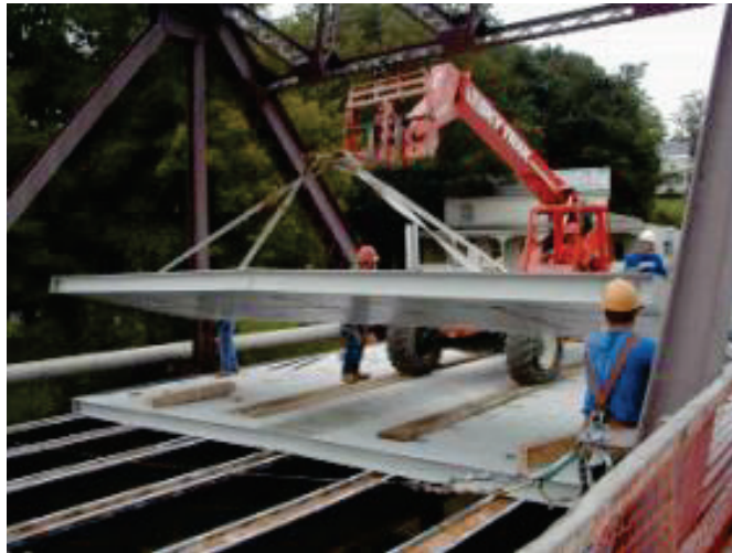
Figure 1. Photo. Typical installation of FRP deck panels on an existing bridge.
