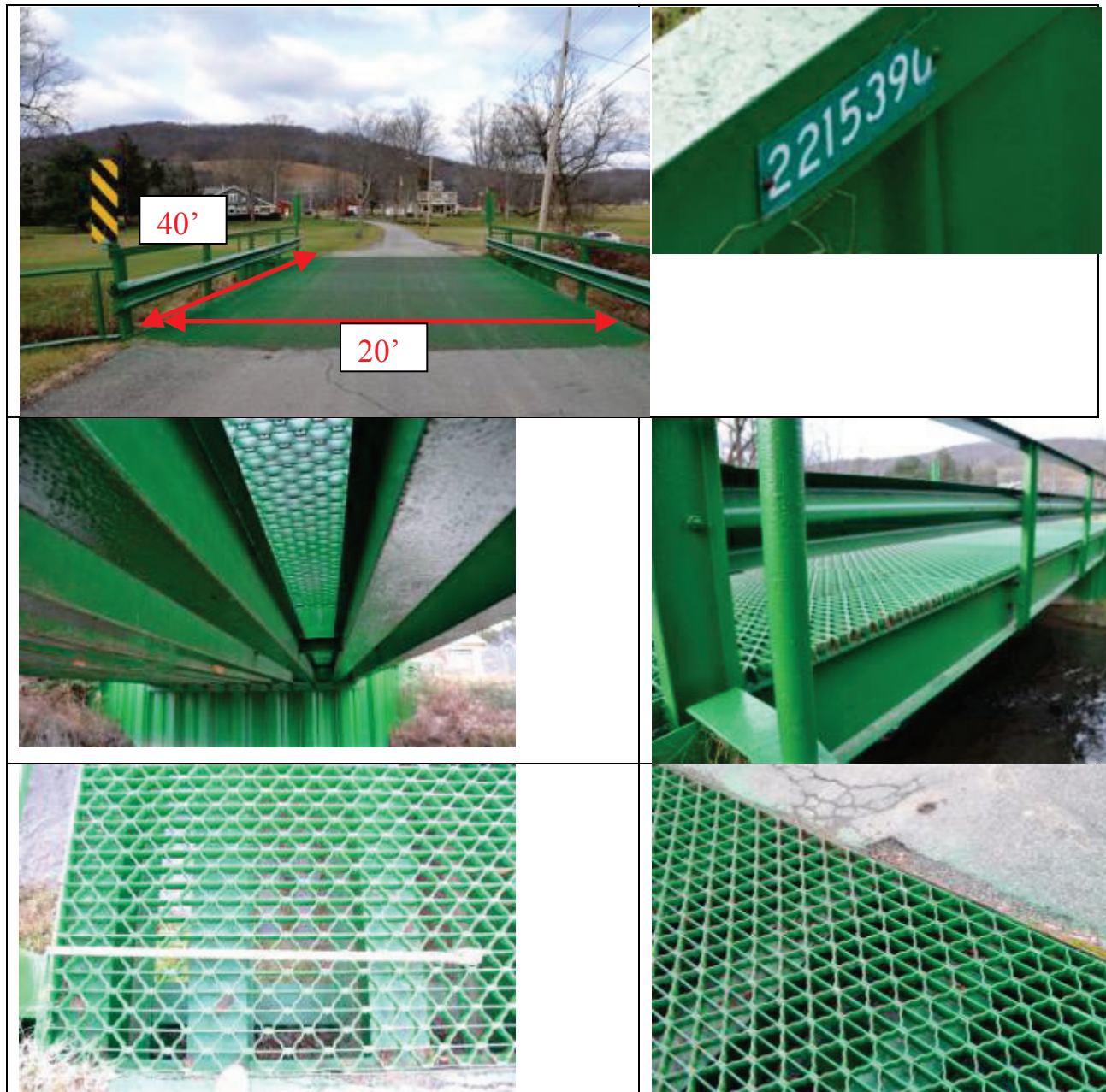
Figure 16. Photos. Existing conditions as of November 2010.
