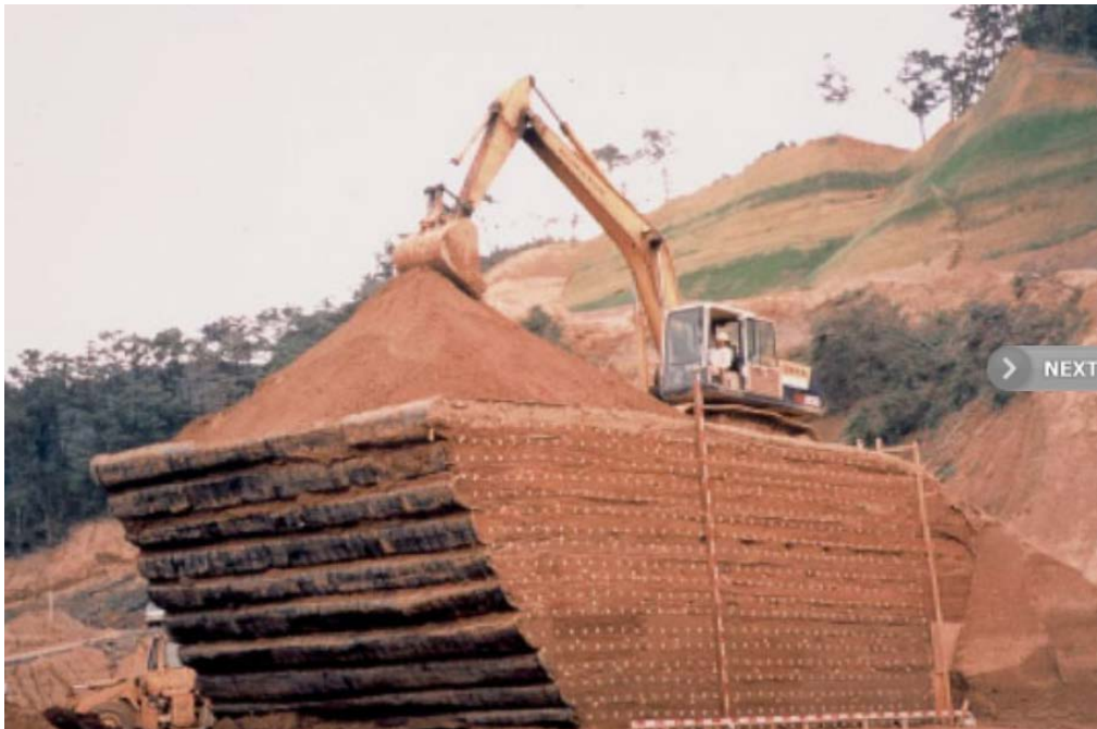
Figure 24. Photo. GRS wall in New Zealand with a negative. (59)
