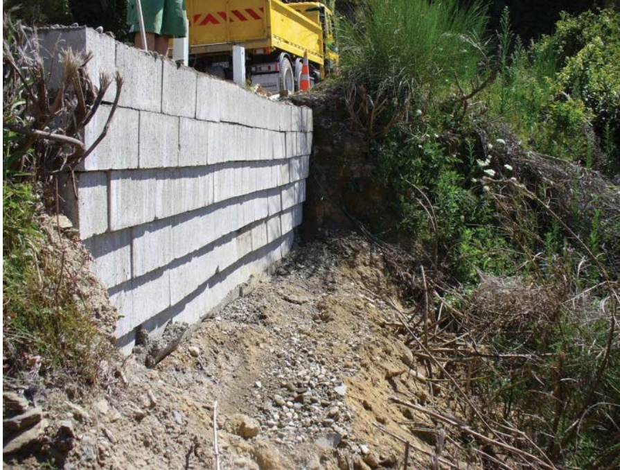
Figure 24. Photo. GRS wall in New Zealand with a negative. (59)
