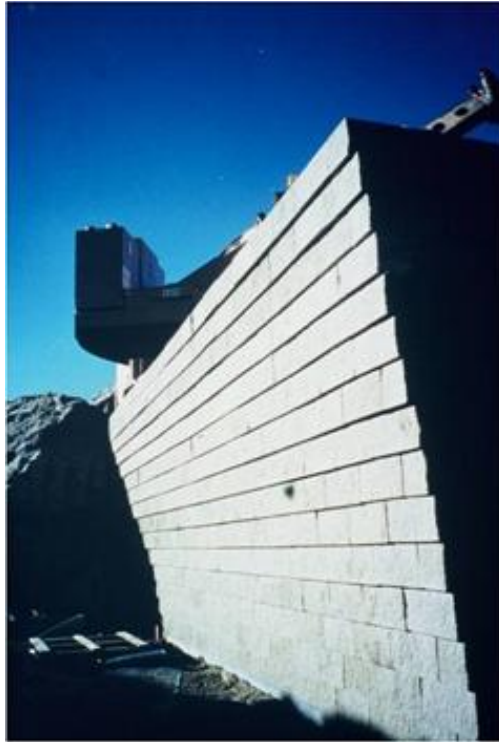
Figure 23. Photo. First negative batter GRS wall constructed in Colorado for CDOT. (59)
