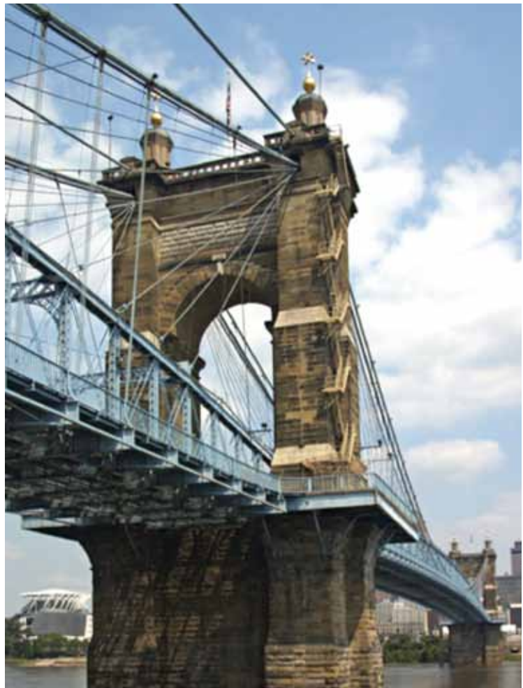
Figure 10. Kentucky's Charles Roebeling suspension bridge is an example of a unique asset.
