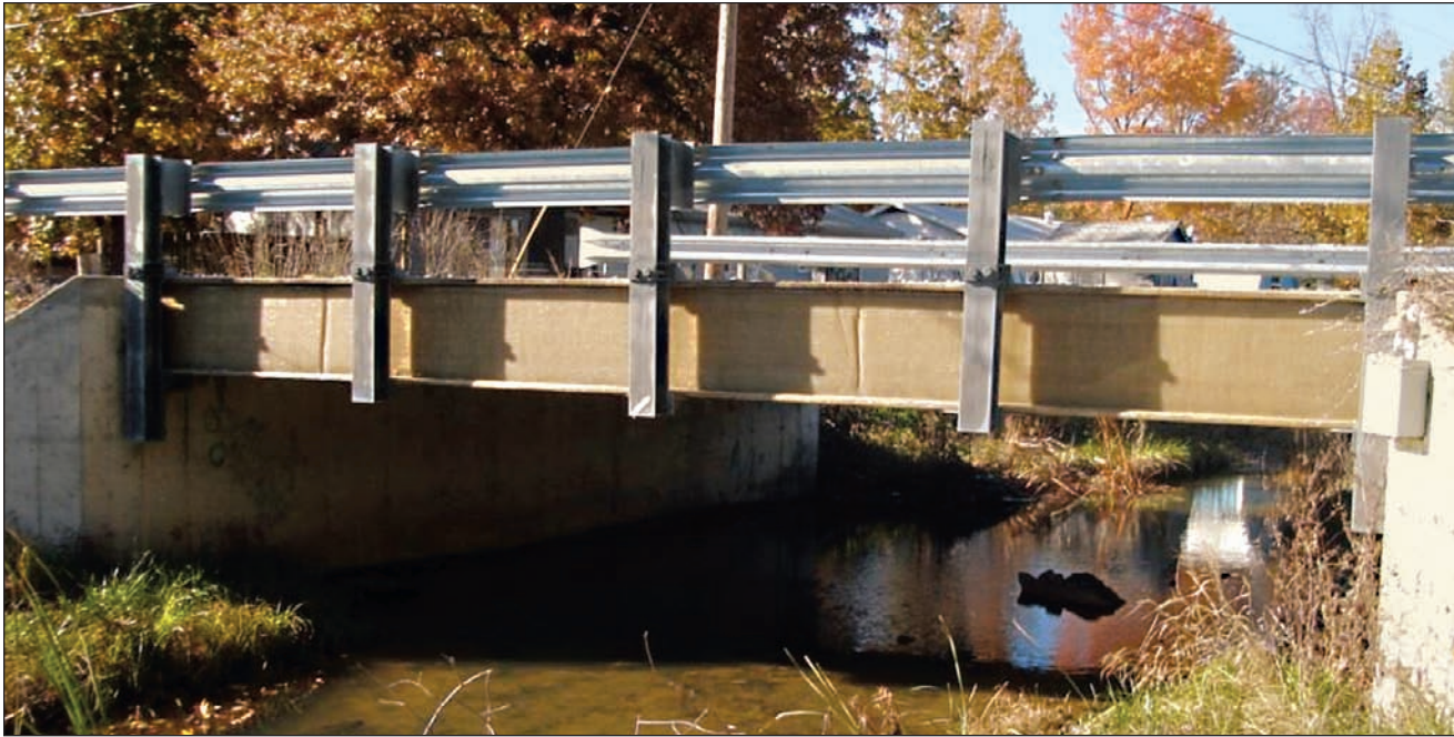
Fiber-reinforced polymers composite bridge. (photo: Dr. John J. Myers)
