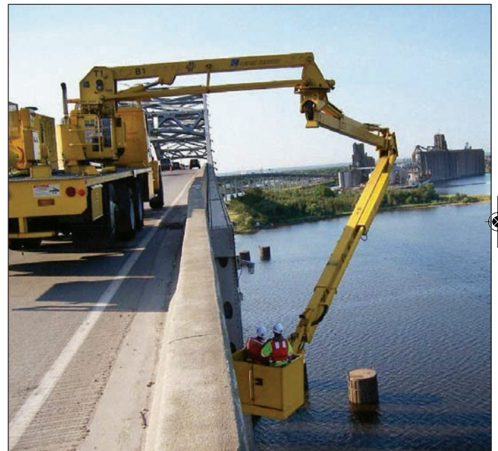
Long-term bridge performance researchers are conducting detailed bridge inspections using visual inspection as well as nondestructive evaluation techniques. (photo: Parsons Brinckerhoff)
