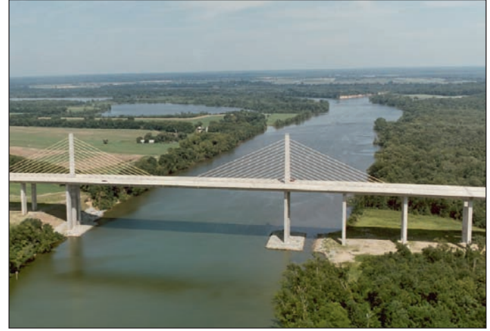
Varina-Enon Bridge. The structural “health” of this cable-stayed bridge was evaluated using acoustic emission sensors. Corrosion of single-stay cables can be determined by this method. (photo: Virginia DOT and Virginia Transportation Research Councils)
