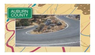
Here is an example of how a county created an action plan that aligned with the State's SHSP. Many of the roads in Auburn County have sharp curves. The roads are former wagon trails and had been transformed over time without addressing roadway alignment, clear zones or lighting. Consequently, many road departure crashes at curves occur throughout the county.
