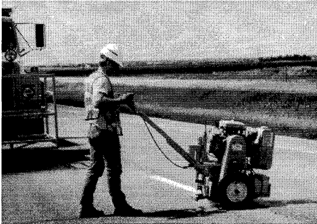
Figure 16. Carbide-tipped rotary-impact router.
