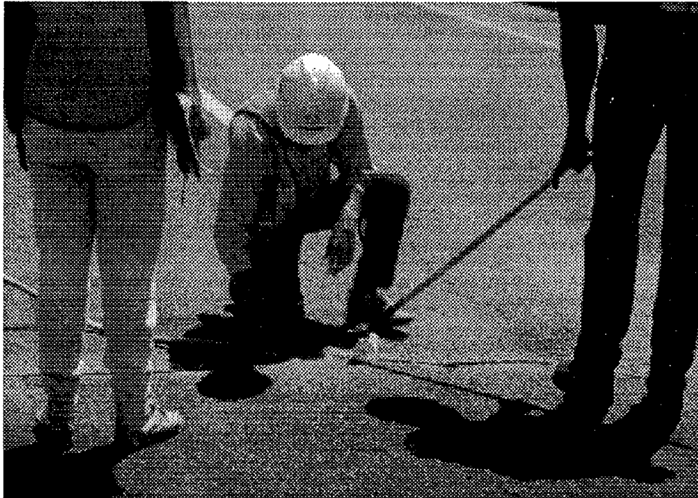
Figure 13. Backer rod installation.
