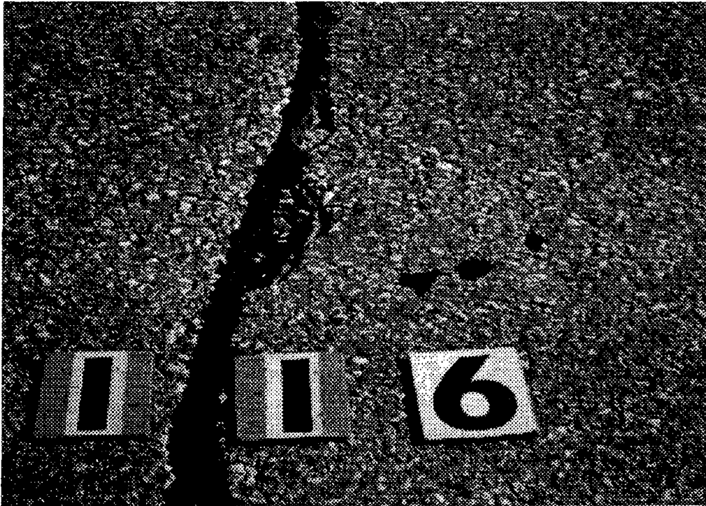
Figure 35. Typical spall and secondary crack adjacent to 890-SL silicone seal.
