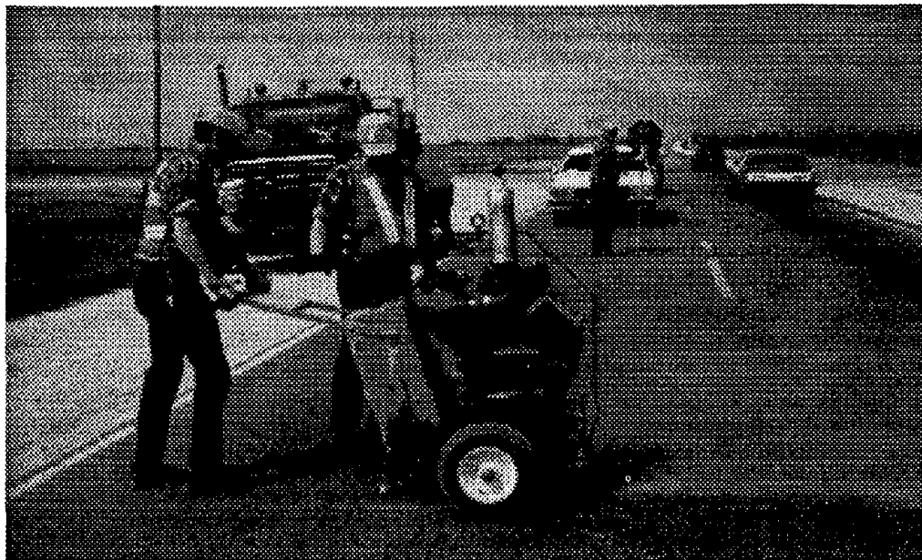
Figure 17. Random crack saw with 200-mm diamond blade.
