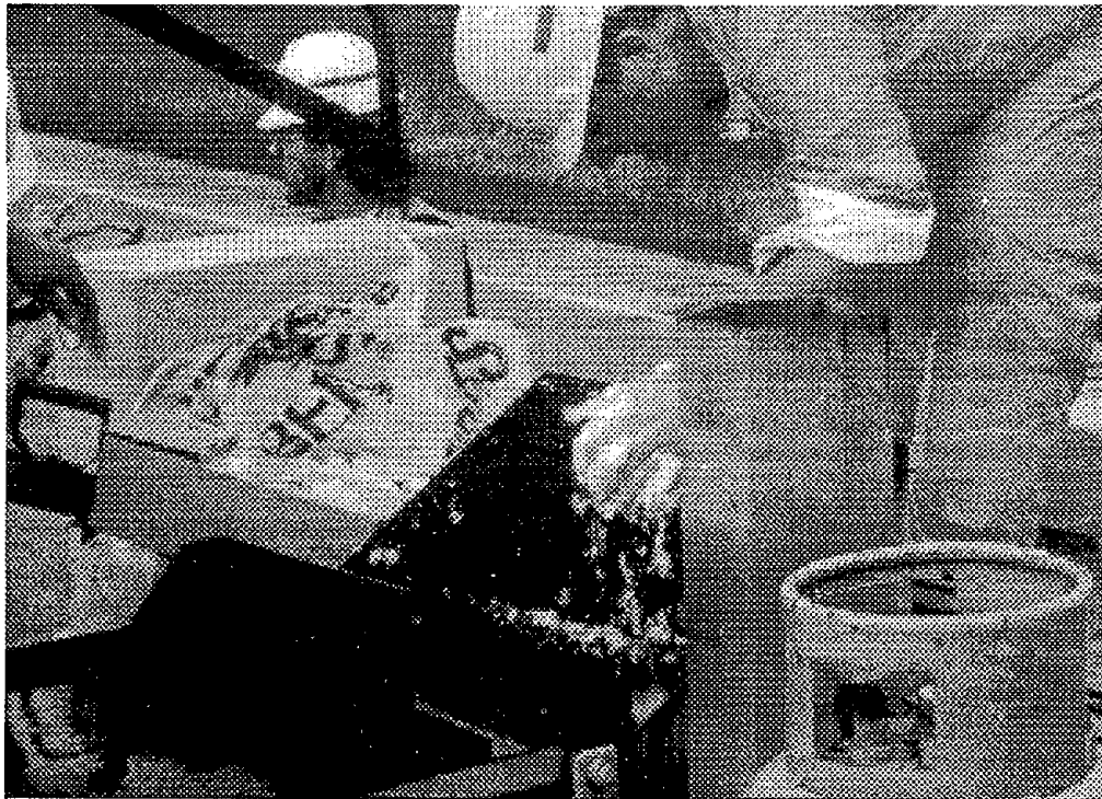
Figure 12. Addition of BoniFiber polyester fibers to asphalt cement.
