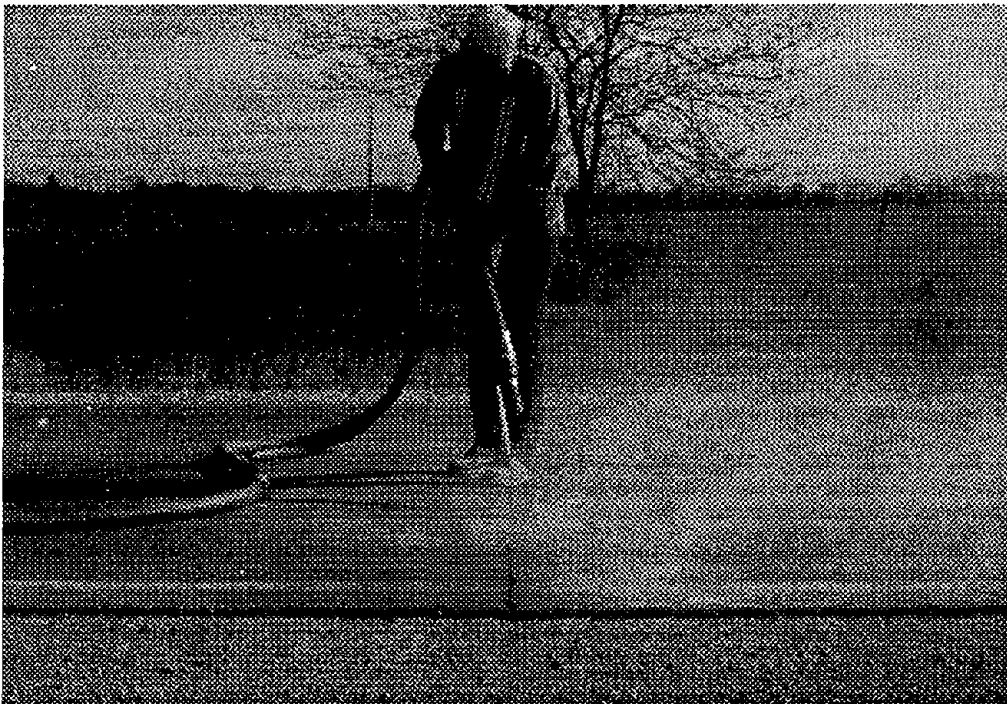
Figure 19. Light sandblasting using wand with attached wooden guide (crack preparation procedure 5).
