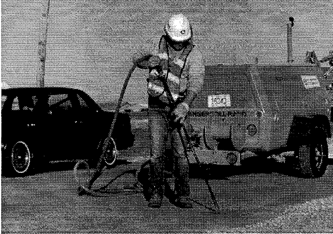
Figure 14. Airblasting operation.
