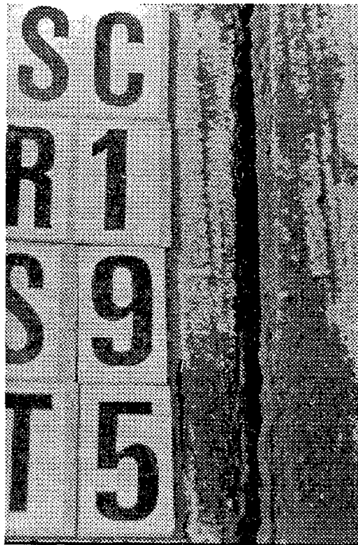
Figure 26. Overband wear.
