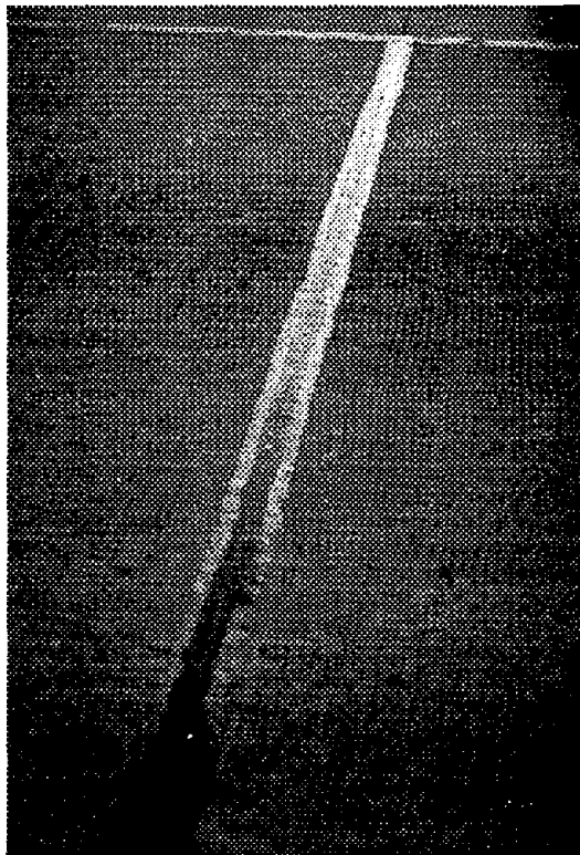
Figure 18. Overbanded sealant installation.
