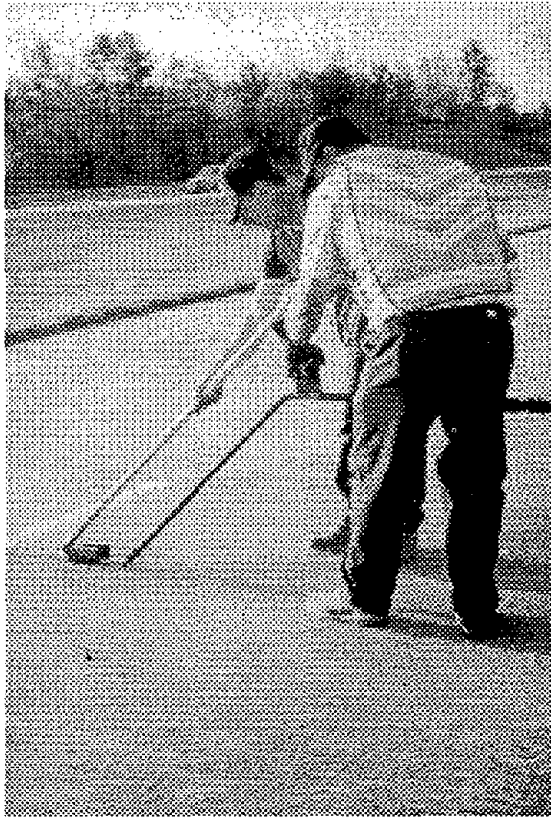
Figure 18. Overbanded sealant installation.
