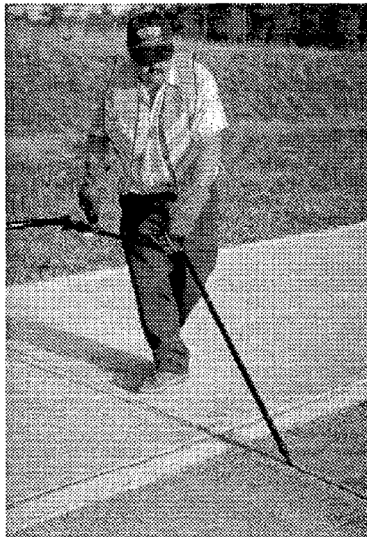
Figure 16. Recessed sealant installation.
