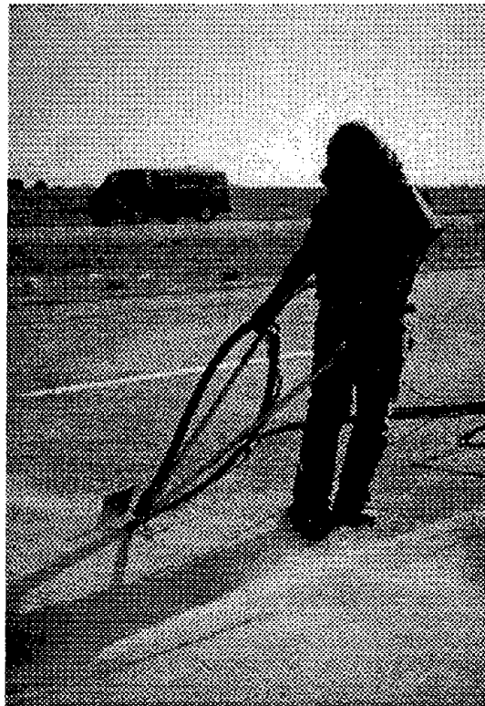
Figure 13. Sandblasting operation.
