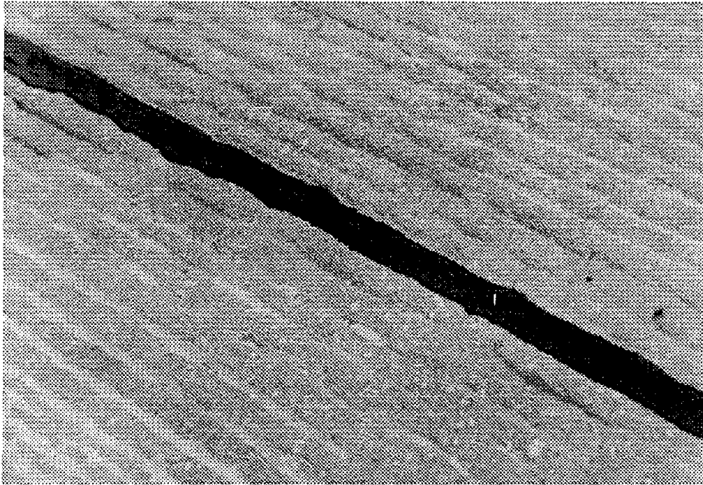
Figure 17. Installed flush-filled sealant.
