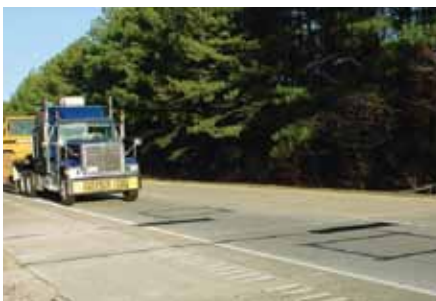
Truck approaching a WIM installation in Arkansas.
