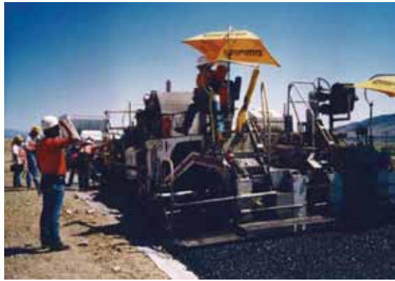
Above: Construction of an Arizona SPS-1 site in 1993.
