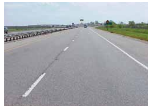
Above: A pavement test section with a 2-in. recycled asphalt overlay.
