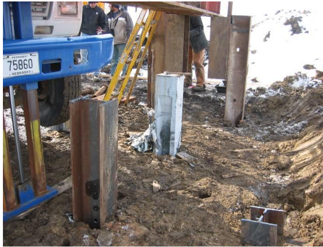
Figure 22. Photo. Experimental precast pile made of UHPC
