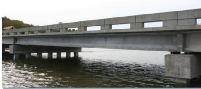
Figure 14. Photo. Route 64 over Cat Point Creek, Richmond County, VA
