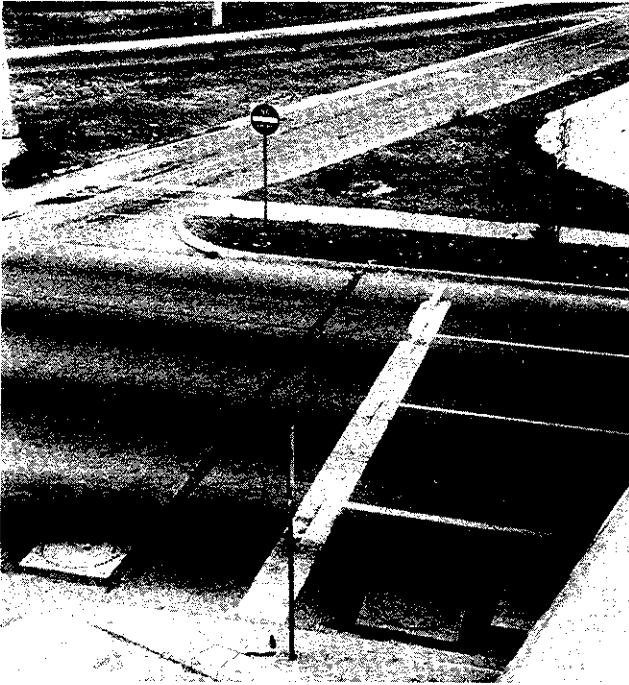
Figure 136. Slab loop installations.
