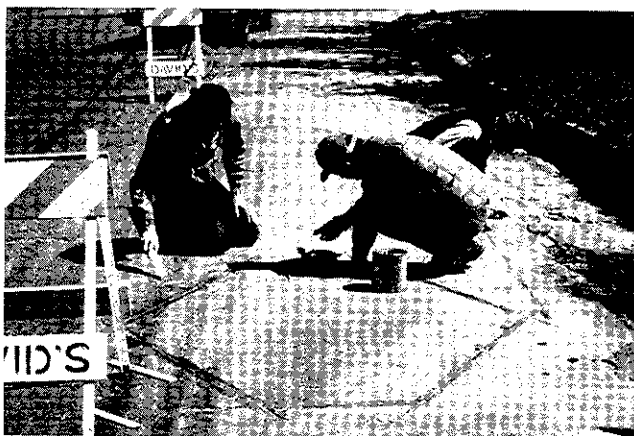
Figure 127. Finishing the sealant application.
