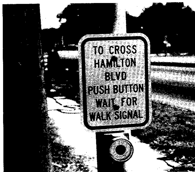
Figure 63. Passive pedestrian push button.
