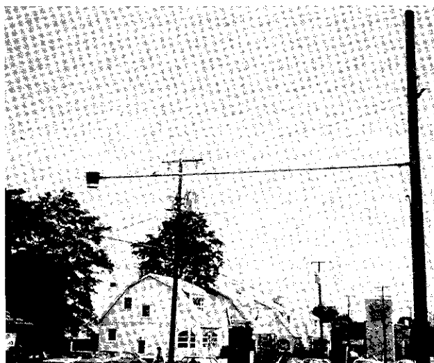
Figure 6. Overhead-mounted radar detector.
