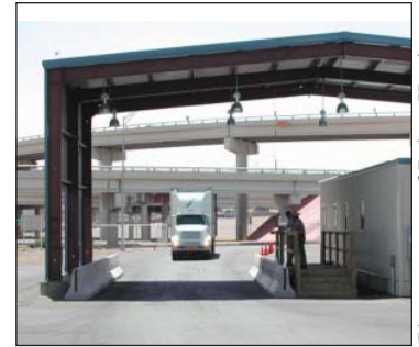
Entrance to the El Paso Border Safety Inspection Facility.
