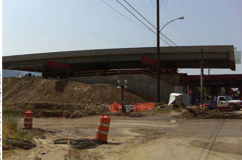
Bridge span nearing its final position
