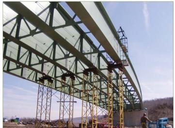
Superstructure of Bridge #207, carrying State Route 322 over Interstate 99 in Centre County, PA, showing shoring (yellow) used to stabilize horizontally curved steel girders during construction. Researchers from Penn State's Larson Institute are developing better approaches for designing and analyzing curved and skewed structures during construction to ensure that costly and hazardous fabrication mistakes are a thing of the past.
