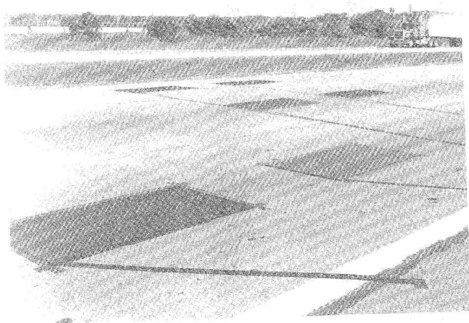
Figure 12. Typical Layout of Speed Mats on Three Lanes
