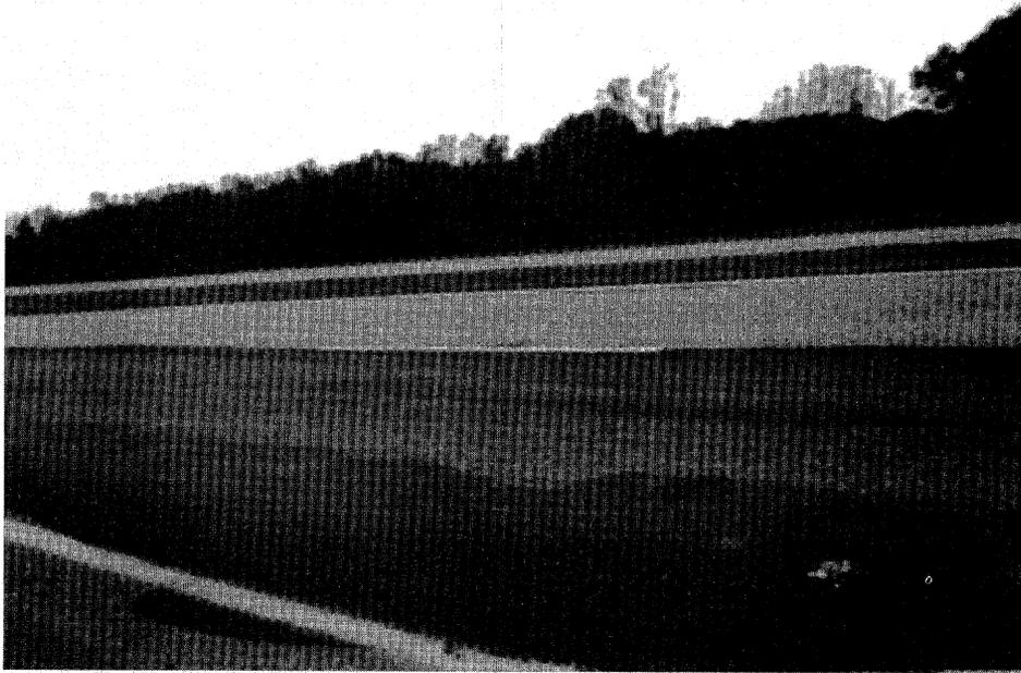
Figure 36. A typical rut in AC overlay of CRC pavement.
