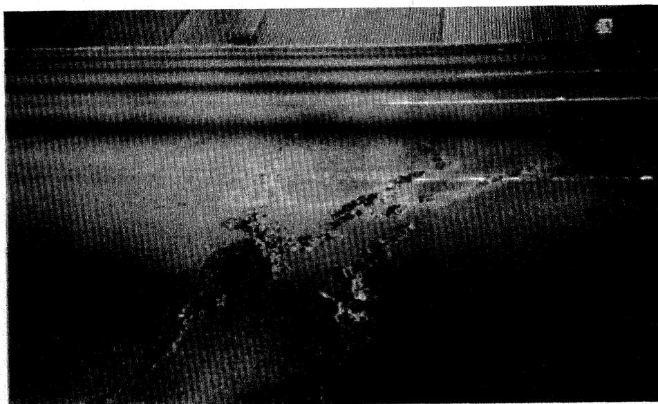
Figure 12. Close-up of crack spalling.
