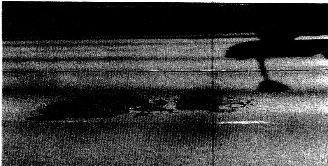
Figure 11. Bituminous patch in existing CRCP.
