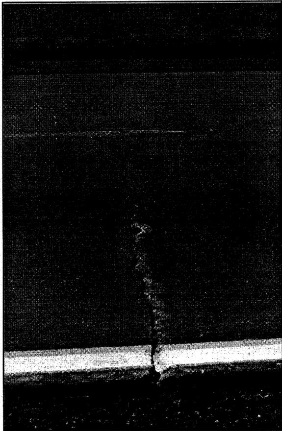
Figure 10. Extra wide crack in existing CRCP.
