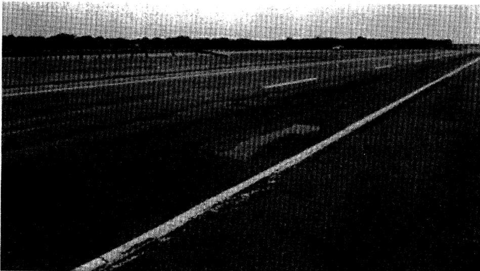
Figure 41. Wheelpath ruts in AC overlays of CRCP (I-45S).
