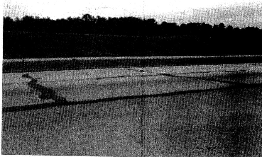
Figure 35. Reflection crack in AC-overlaid CRCP.
