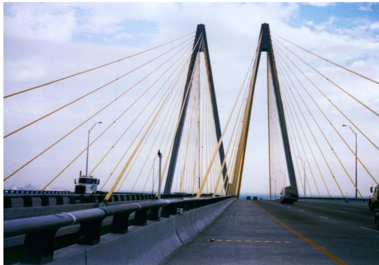
Figure 40. Photo. The cable network of the Fred Hartman Bridge in Houston, TX.
