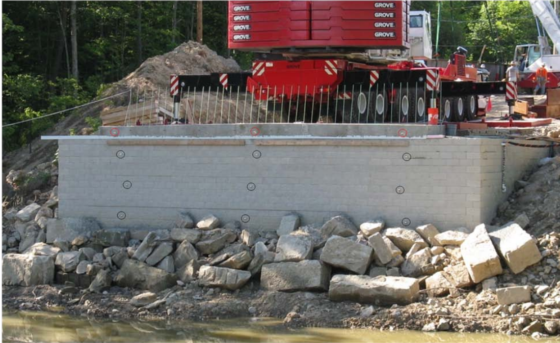
Figure 38. Photo. Location of survey targets on Tiffin River Bridge, Defiance County, OH.
