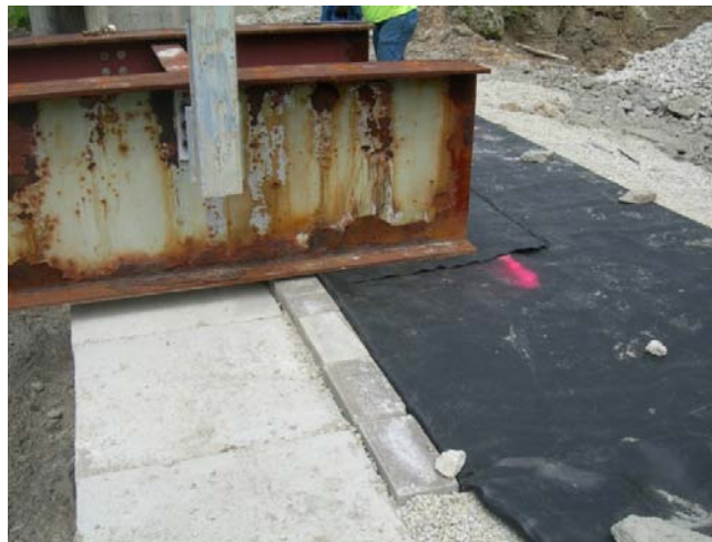
Figure 73. Photo. Additional reinforcement under beam.
