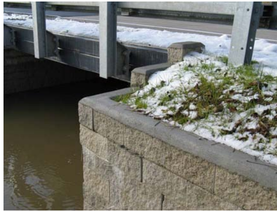
Figure 61. Photo. Rounded coping cap.
