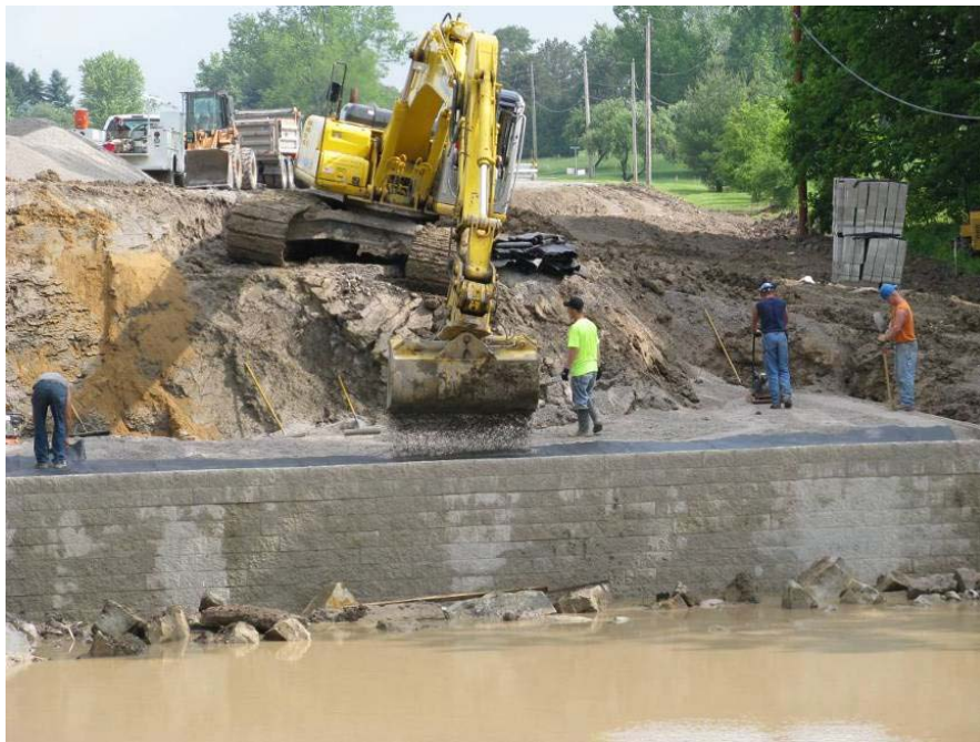
Figure 40. Photo. Typical labor crew with centrally located track hoe.
