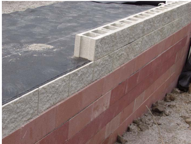
Figure 3. Photo. Split face CMU blocks.
