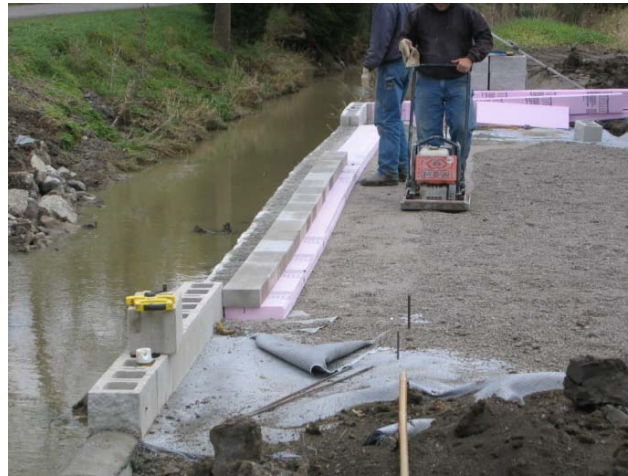
Figure 66. Photo. Foam board and 4-inch block assembly to form beam seat.
