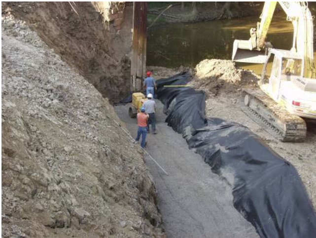
Figure 48. Photo. Encapsulation of fill in RSF.
