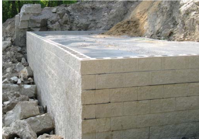
Figure 57. Photo. Right-angle wall corner.
