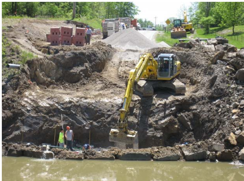
Figure 46. Photo. RSF excavation below stream level.
