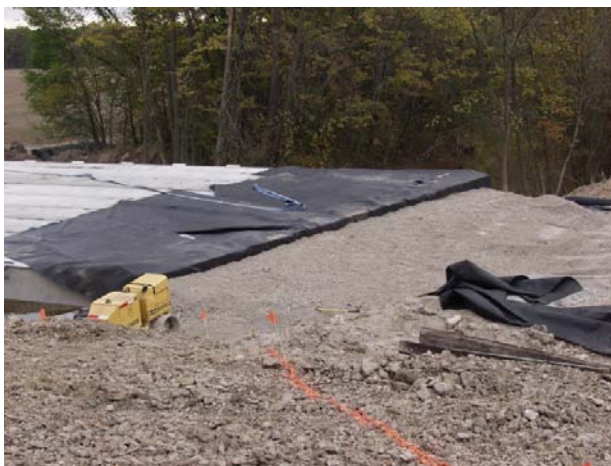
Figure 80. Photo. Second 6-inch fill lift.
