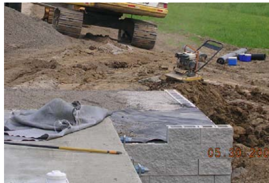
Figure 75. Photo. Parapet and wing wall construction, view 2.
