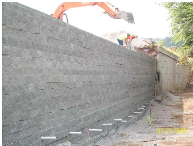
Figure 82. Photo. Use of GRS wall to repair damaged MSE wall.
