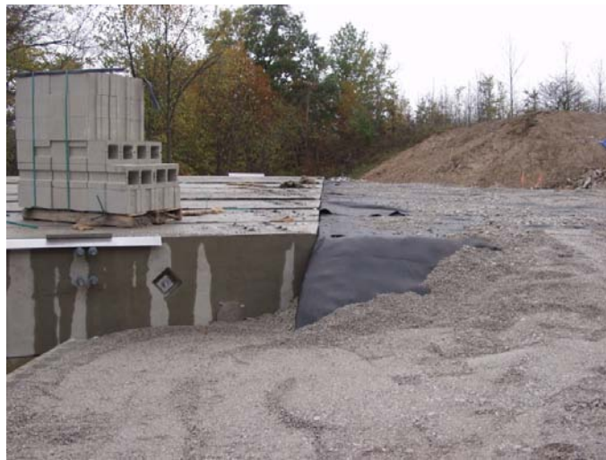
Figure 81. Photo. Completed approach fill.
