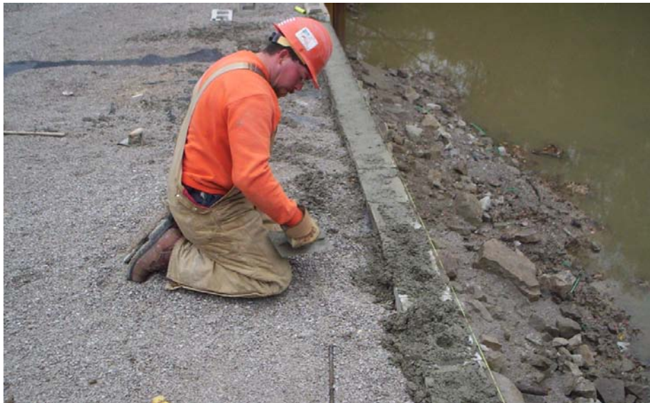
Figure 60. Photo. Connecting the top courses of blocks.
