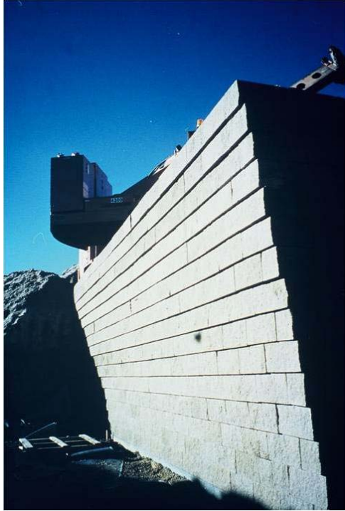
Figure 55. Photo. Negative batter wall face.
