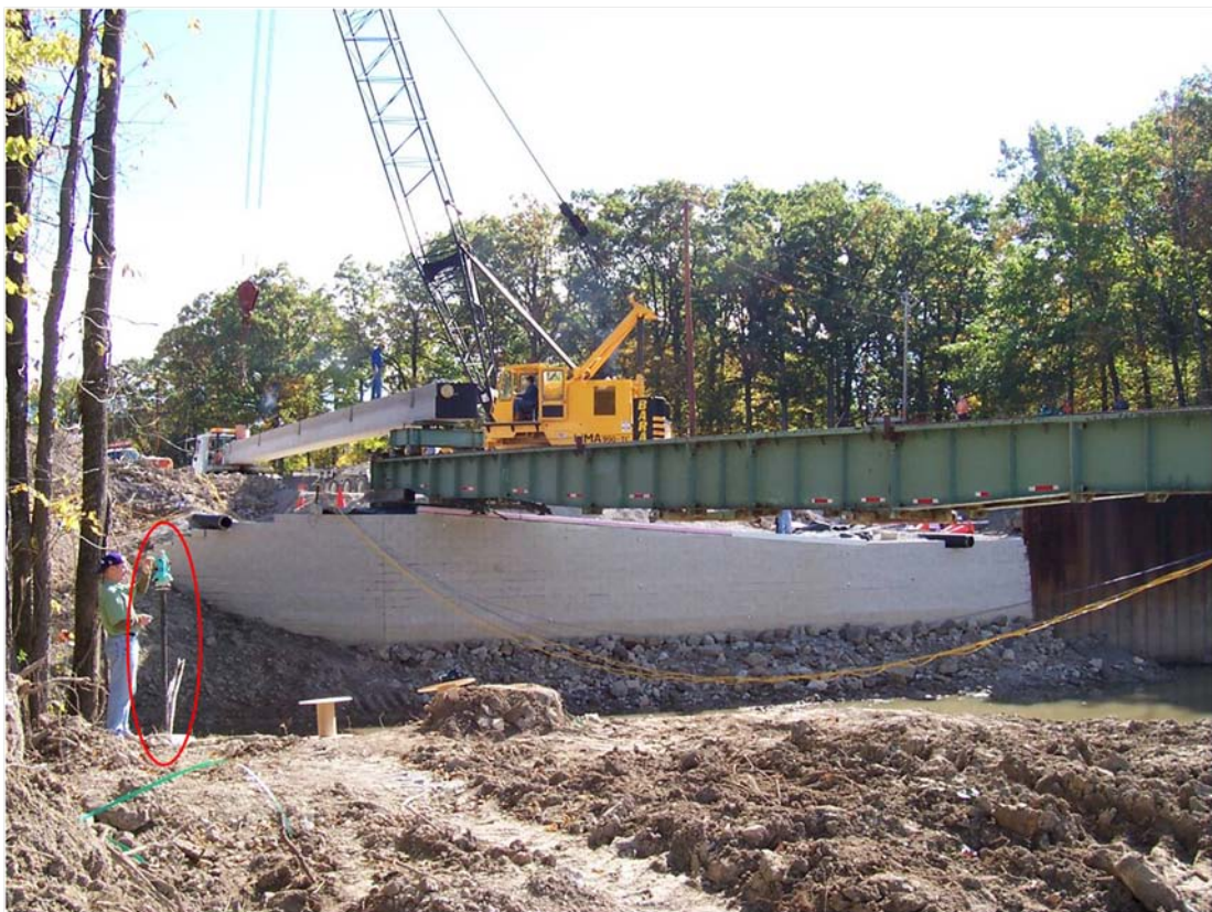
Figure 39. Photo. Location of total station reference pole.
