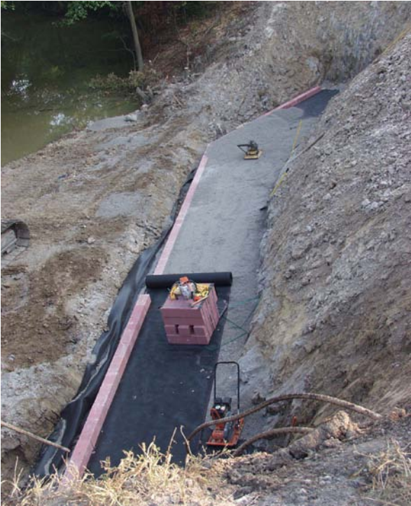
Figure 51. Reinforcement rolled out parallel to wall face.
