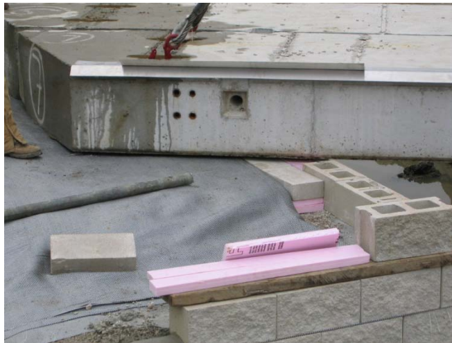
Figure 69. Photo. Top 4-inch wrap butted against 4-inch solid block.
