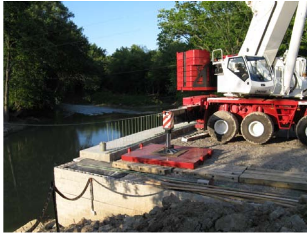
Figure 72. Photo. Outrigger pads near wall face.
