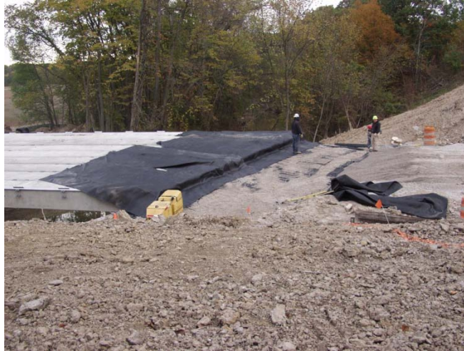
Figure 76. Photo. Placing reinforcement.
