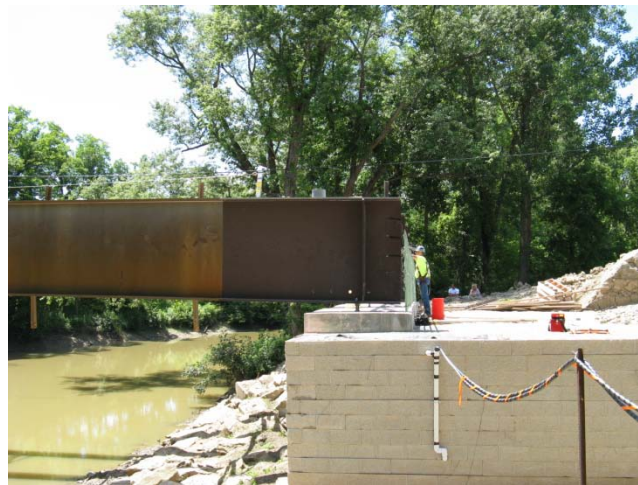
Figure 71. Photo. Steel girder on CIP footing.
