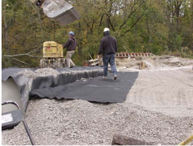
Figure 78. Photo. Secondary reinforcement sheet.
