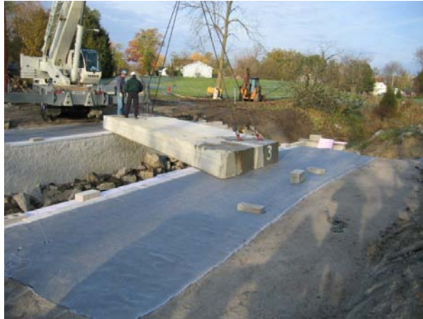
Figure 63. Photo. Box beam placed on beam seat.
