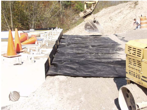
Figure 79. Photo. Completed wrapped approach layer.
