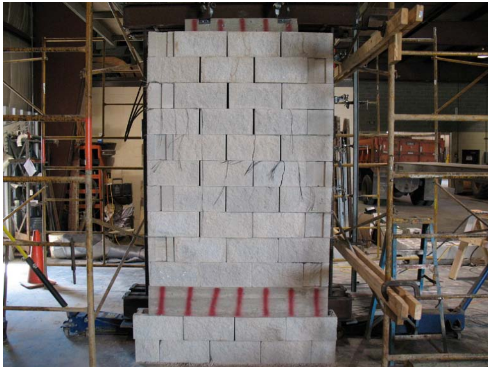
Figure 97. Photo. Defiance County experiment after testing.
