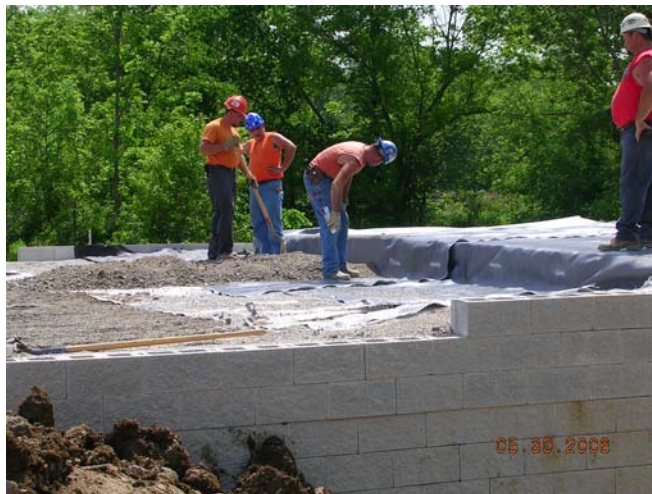
Figure 77. Photo. First 6-inch fill lift.
