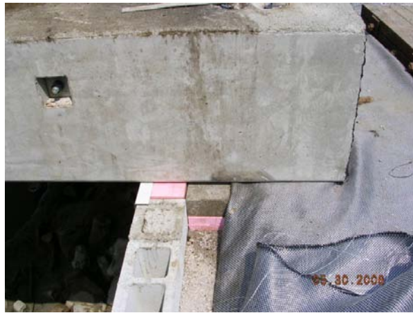
Figure 64. Photo. Detail view of box beam placed on beam seat.
