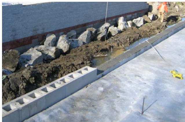
Figure 65. Photo. Bearing area block grouted prior to beam placement.
