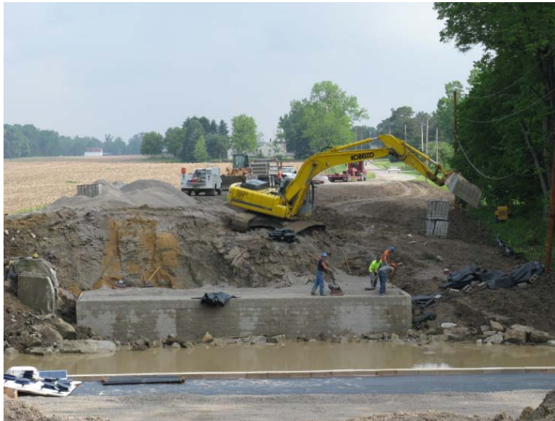
Figure 42. Photo. Horseshoe-shaped excavation with native soil still intact in middle.
