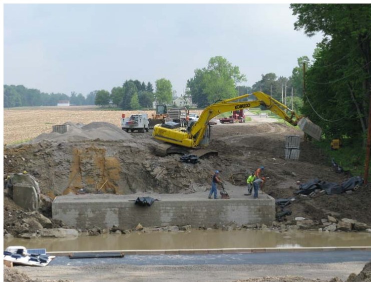
Figure 25. Photo. GRS abutment and wing walls built around core of native soil
