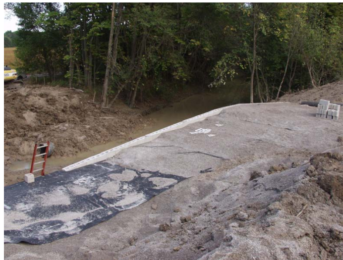
Figure 53. Photo. Superlevation reinforcement layers.
