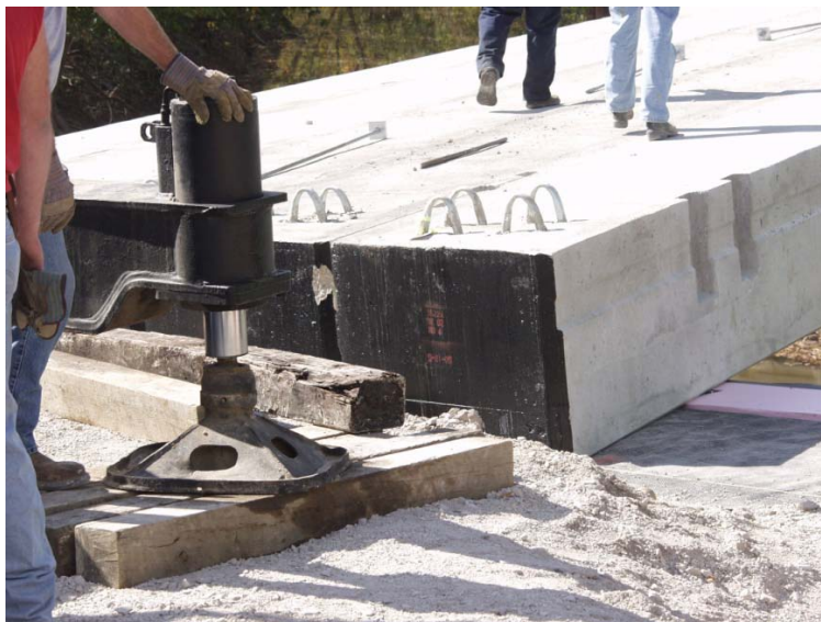
Figure 8. Photo. Bitumen coating on concrete beam ends.
