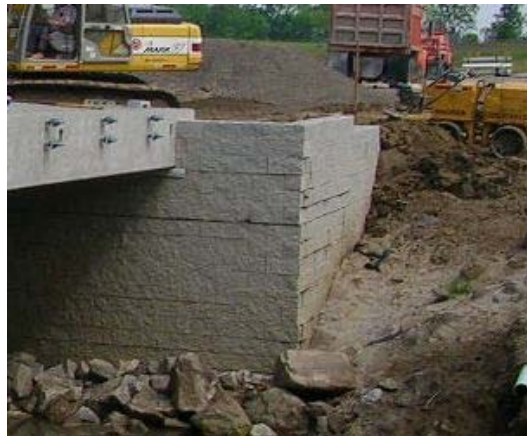
Figure 74. Photo. Parapet and wing wall construction, view 1.
