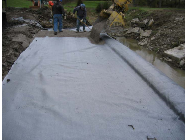
Figure 68. Photo. First 4-inch wrap butted against foam board.
