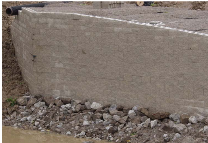
Figure 56. Photo. Blocks trimmed to match superelevation.
