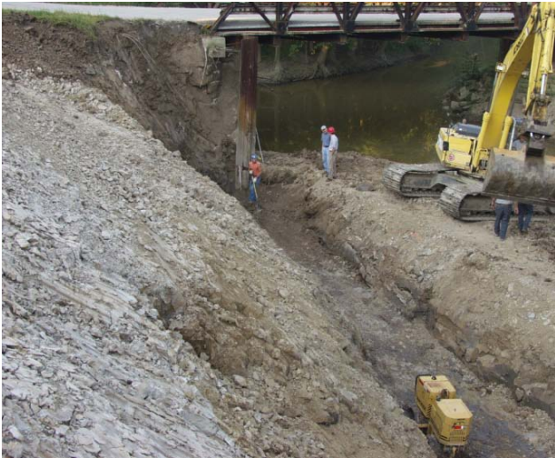
Figure 47. Photo. RSF cut preparation.
