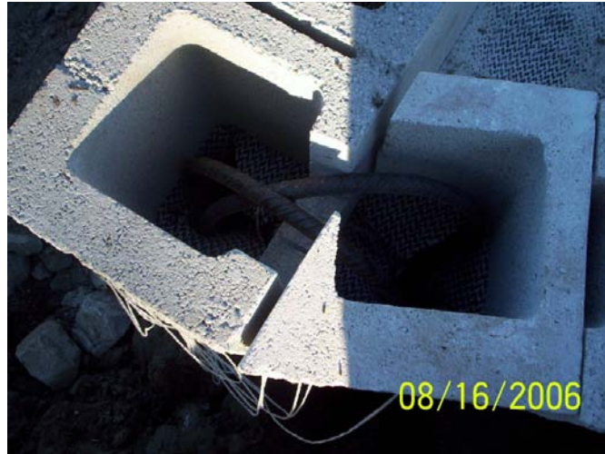
Figure 59. Photo. Rebar installed in vertical seam prior to grout.
