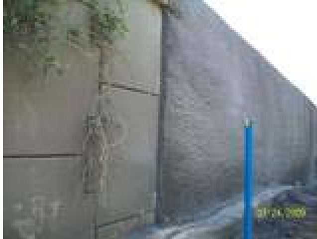
Figure 83. Photo. CMU GRS wall with a shotcrete face.
