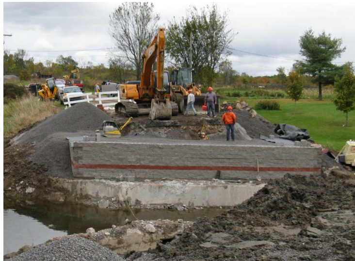
Figure 41. Photo. Cut slope of retained soil.
