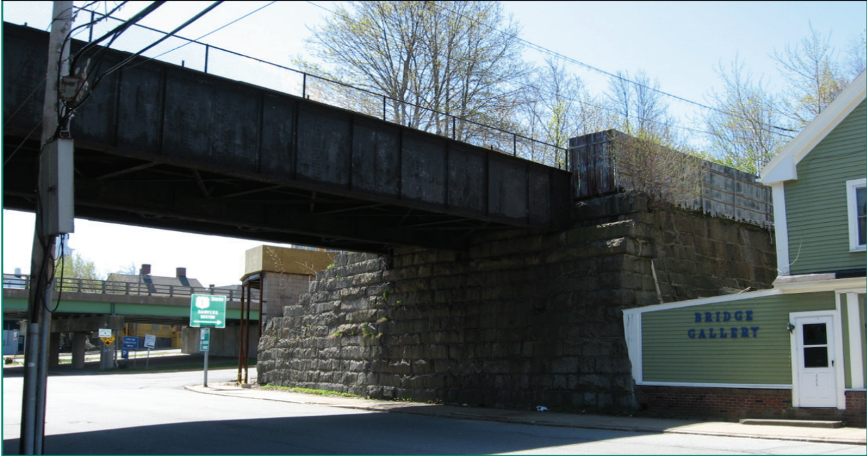
Figure 9. Clipper City Rail Trail Bridge.
