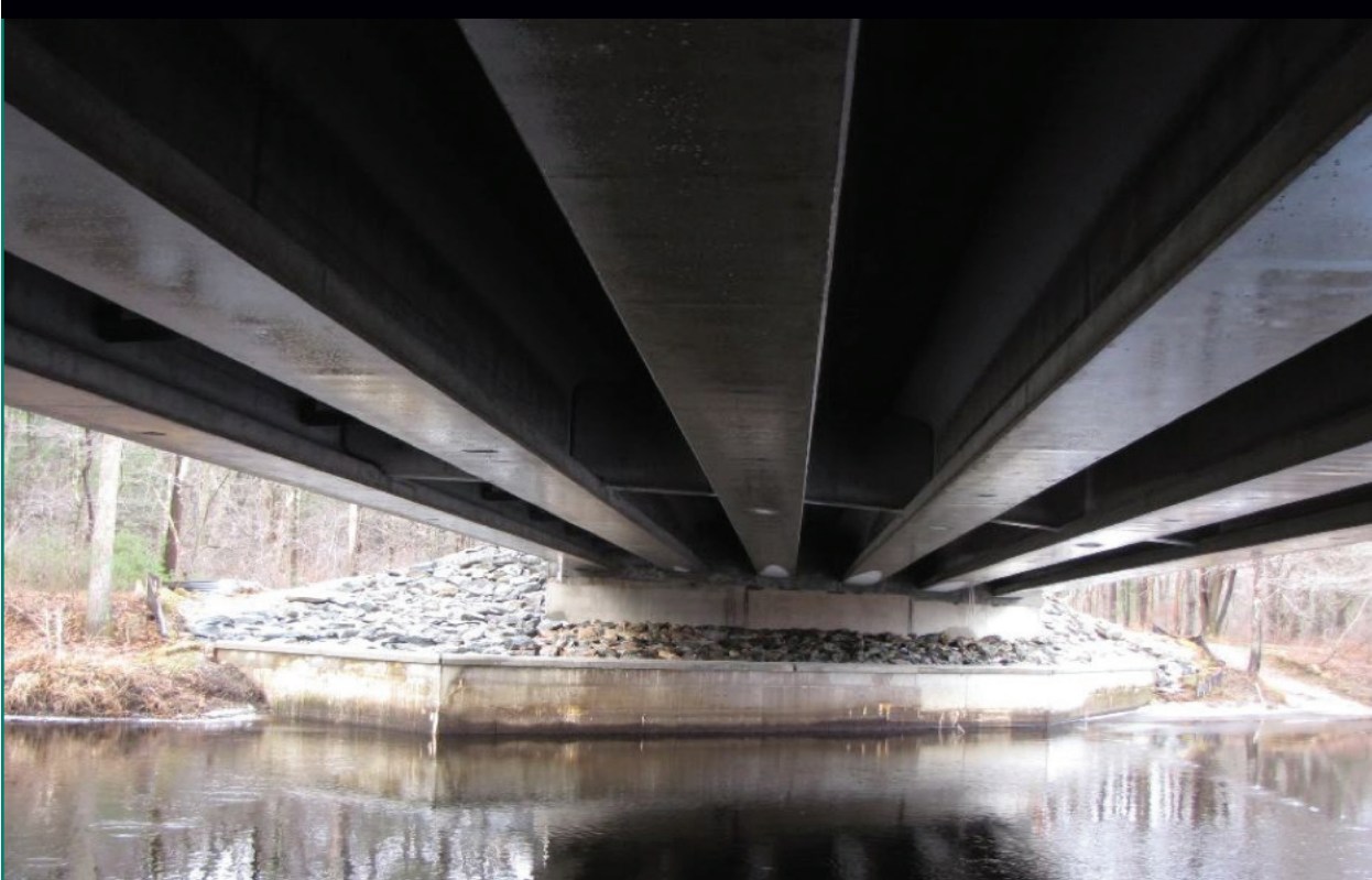
Figure 7. Bridge B-23-005-M-18-002, Bridgewater, MA.
