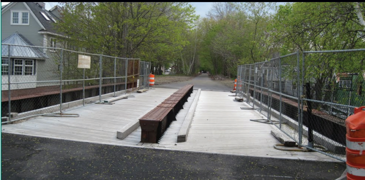
Figure 10. Clipper City Rail Trail bridge deck replacement.
