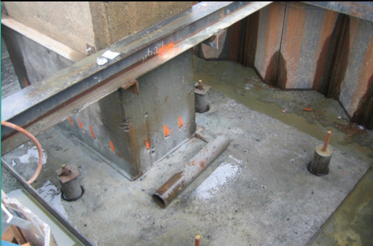
Figure 16. An existing foundation strengthened with micropiles.
