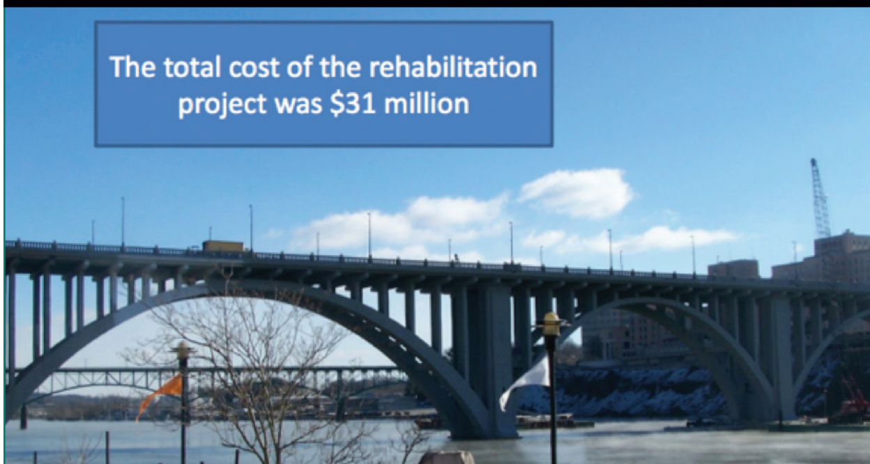
Figure 20. Henley Street Bridge after completion of the rehabilitation.
