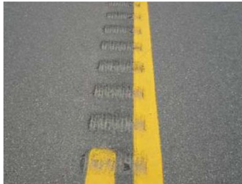
Figure 146. Photo. Longitudinal rumble strips. (111)
