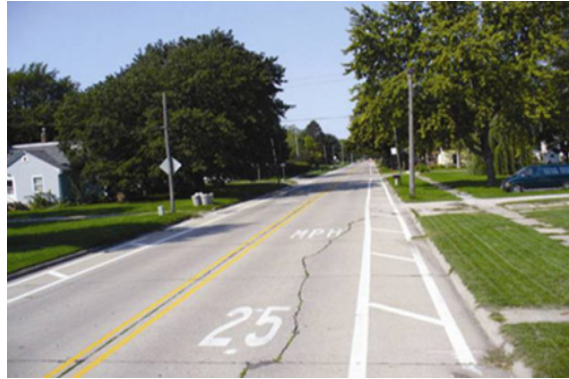
Figure 159. Photo. Add shoulder markings to narrow lane. (53)
