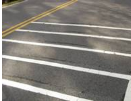
Figure 145. Photo. Transverse rumble strips. (104)
