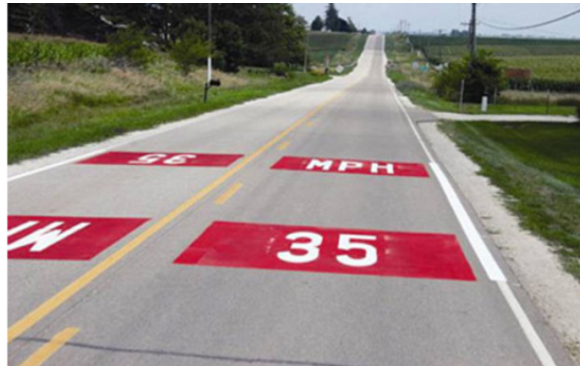
Figure 155. Photo. Enhanced speed limit legend with colored surfacing. (123)
