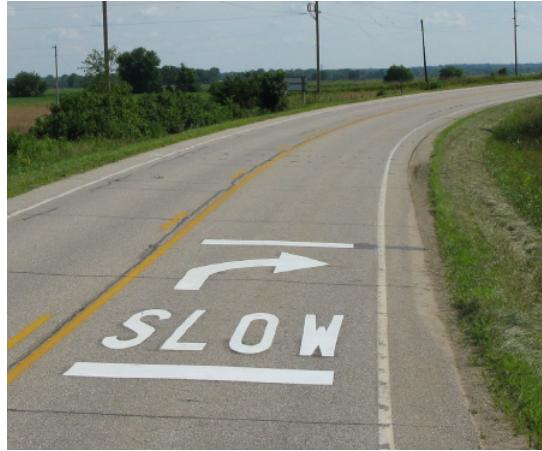
Figure 156. Photo. Slow pavement legend. (52)
