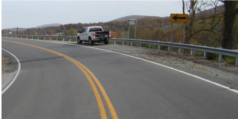
Figure 168. Photo. One-direction large arrow (W1-6) sign.
