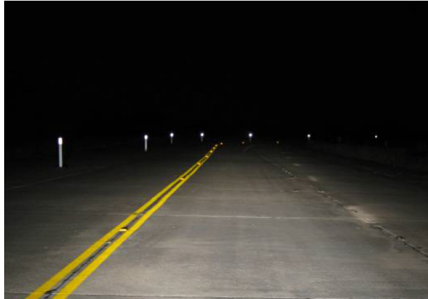
Figure 175. Photo. Delineator post. (151)
