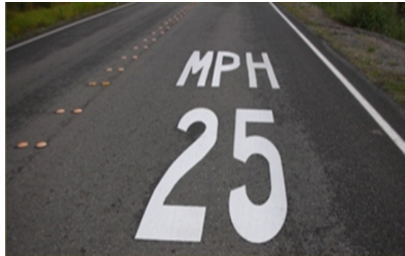
Figure 154. Photo. Speed limit pavement legend. (126)
