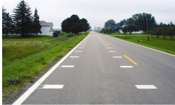
Figure 165. Photo. Transverse pavement markings with speed feedback sign. (53)
