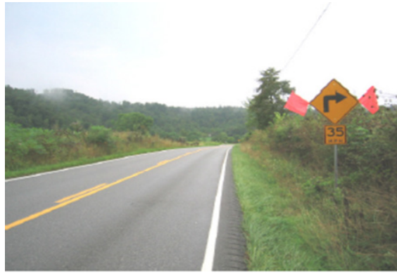
Figure 170. Photo. Curve warning sign with flags. (118)
