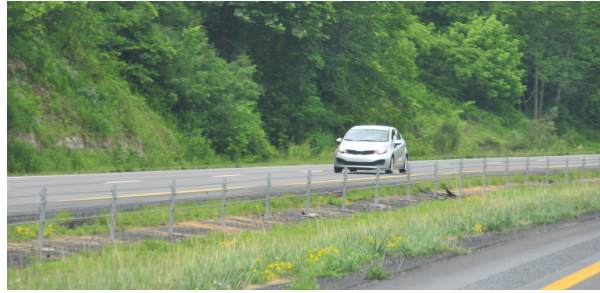
Figure 176. Photo. Median barriers.
