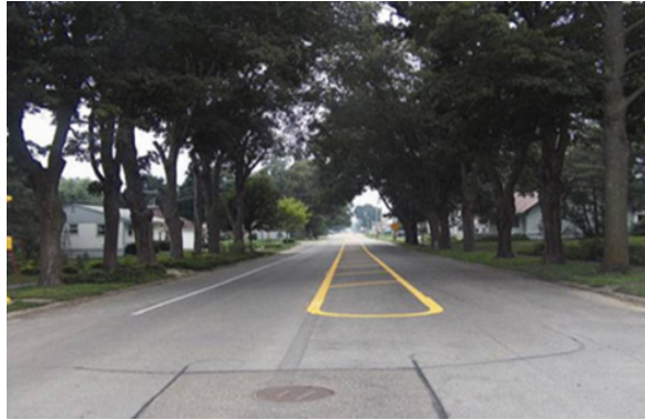
Figure 160. Photo. Add centerline and edge line. (53)
