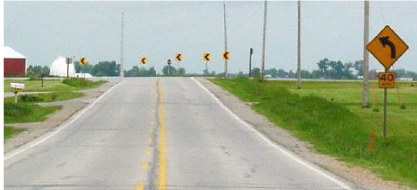
Figure 174. Photo. Curve warning sign and chevron sign.
