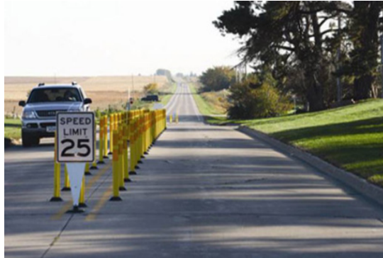
Figure 144. Photo. Tubular channelizers. (53)
