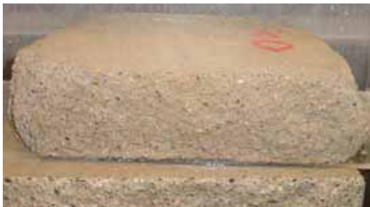
Figure 205. Photo. Non-SHA-approved cap from manufacturer A (water exposure).
