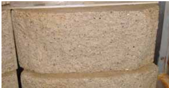
Figure 206. Photo. Surface of non-SHA-approved block from manufacturer A (3 percent NaCl solution).
