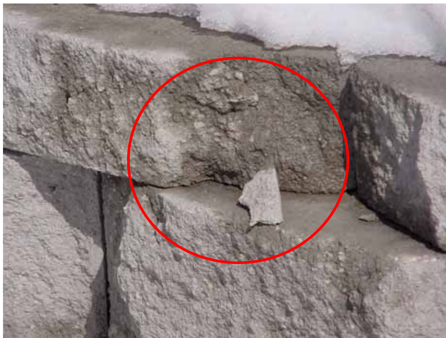
Figure 48. Photo. Detached split face delamination under frost conditions in field SRW units.
