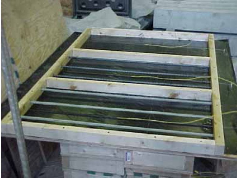
Figure 38. Photo. Concrete slab molds before concrete cast.
