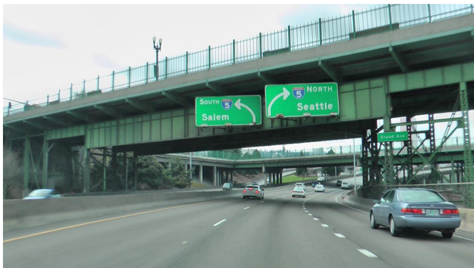
Figure 11. Photo. Example of mismatch between direction of arrows on signs and perceived roadway direction.
