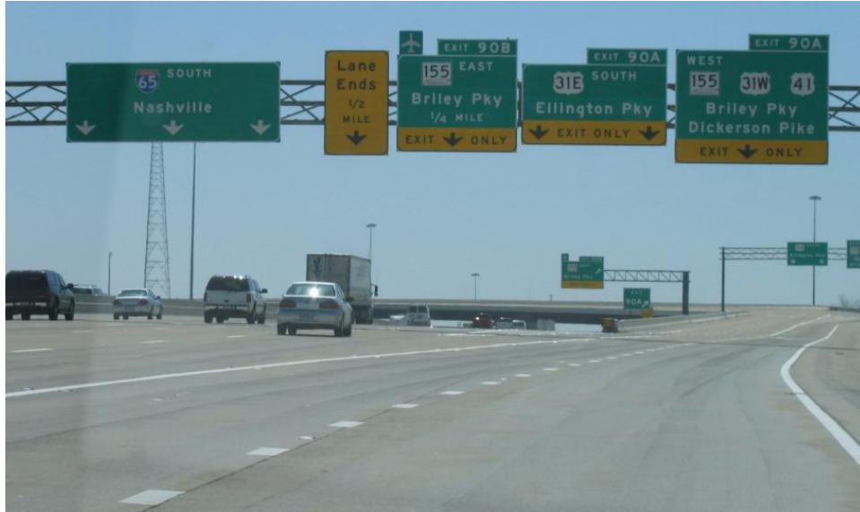
Figure 8. Photo. Example of information overload on a sign structure.
