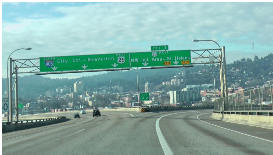
Figure 9. Photo. Example of confusing destination grouping caused by perceptual cues from sign elements.
