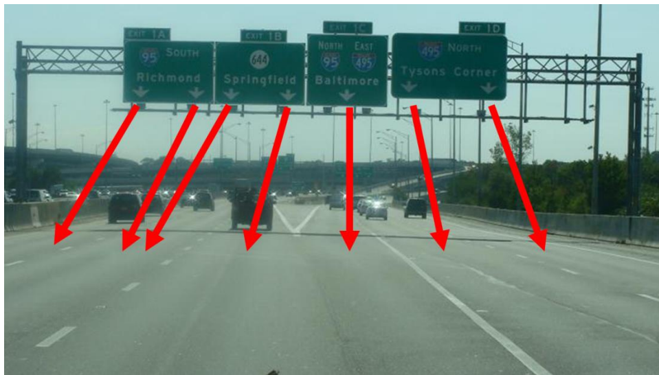
Figure 13. Photo. Example of perceived misalignment between down arrows and lanes.
