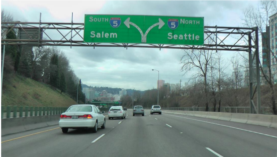
Figure 14. Photo. Example of difficult-to-see lane lines on a diagrammatic sign.
