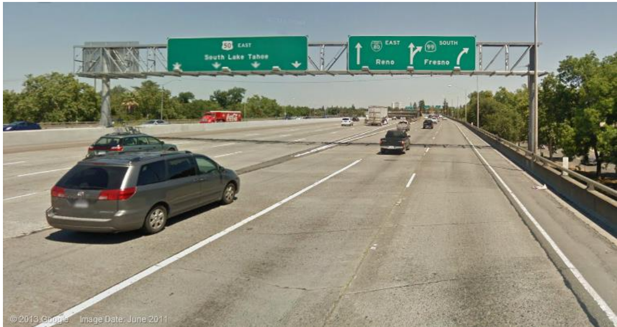
Figure 5. Photo. Example of alternate APL destination name layout. (4)
