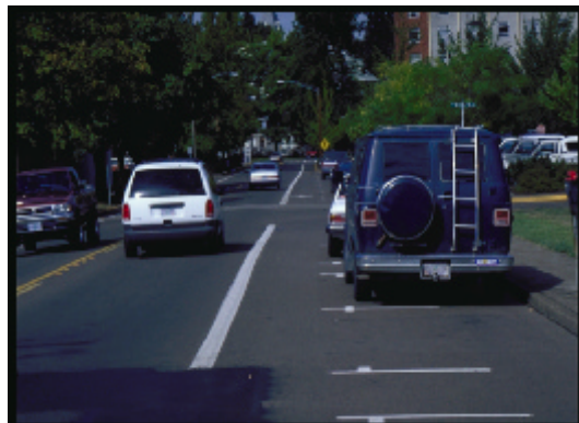
Figure 17. Combination BL with parking T's.
