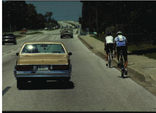
Figure 5. Vehicle encroachment into the adjacent travel lane when passing bicyclists in a WCL.
