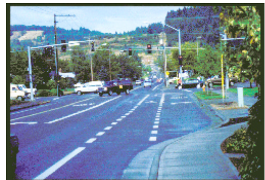
Figure 21. Dashed BL stripe at right-turn situation.
