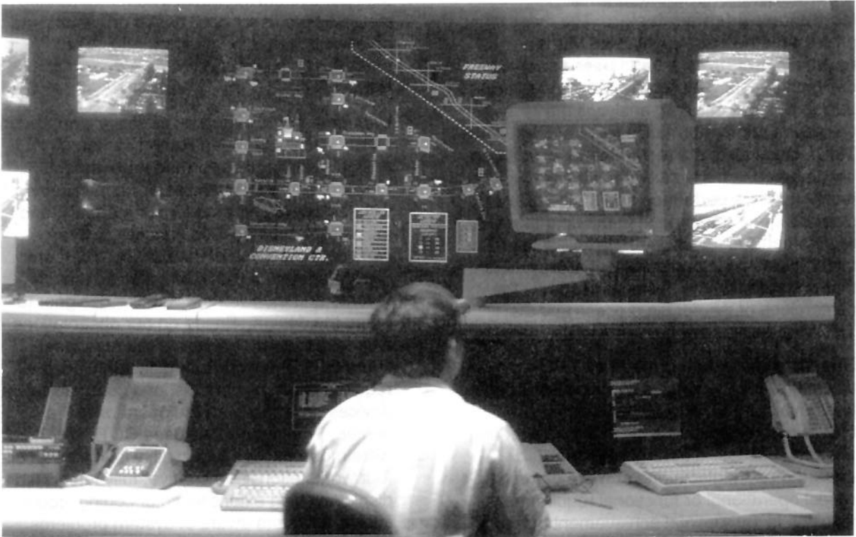
Figure 25. Example of a monitor located above the operator's seated line of regard.
