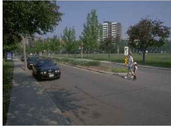
Figure 35. Raised medians and pedestrian islands may provide a measure of safety to pedestrians.
