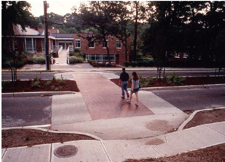
Figure 44. Many traffic-calming measures create an improved environment for pedestrians by reducing vehicle speeds or volumes, and/or shortening crossing distances for pedestrians.
