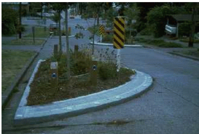
Figure 45. Street narrowing can reduce vehicle speeds and provide pedestrians with a narrower street to cross.
