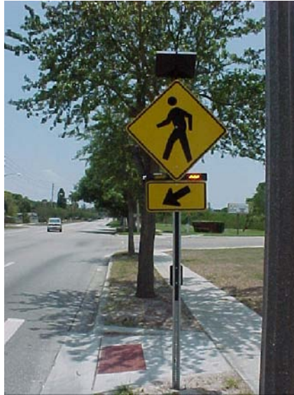
Figure 3. Photo. RRFB with two forward-facing LED flashers and a side-mounted LED flasher.
