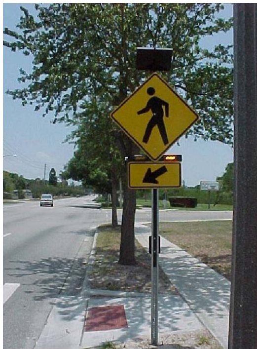
Figure 6. Photo. Example of an RRFB.
