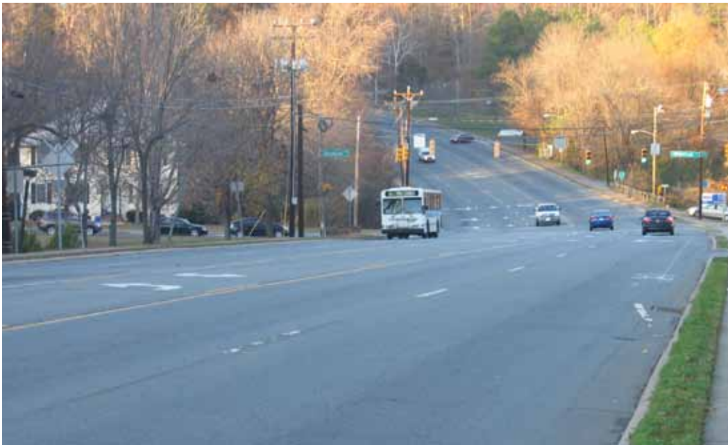
Figure 11. Photo. Outbound view of MLK Boulevard.
