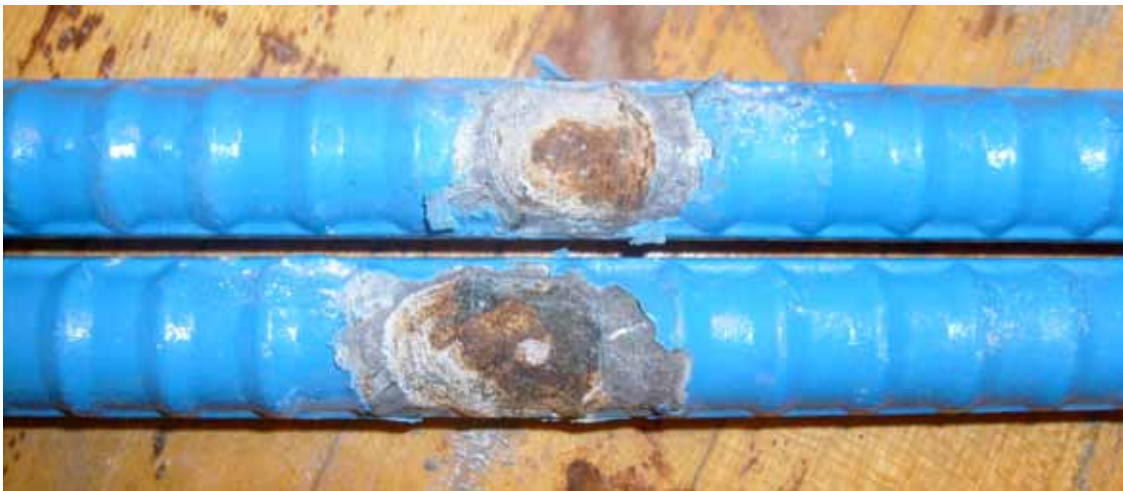
Figure 158. Photo. MC top bars from field test specimen with simulated cracks after 250 weeks.
