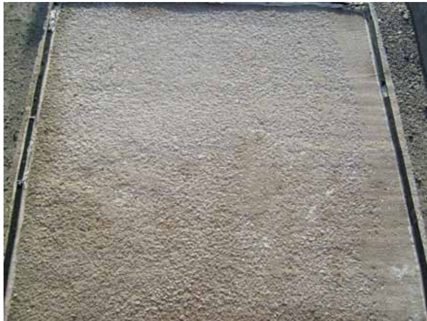
Figure 154. Photo. Field test specimen without simulated cracks containing conventional ECR and Hycrete™ corrosion inhibitor at 250 weeks.
