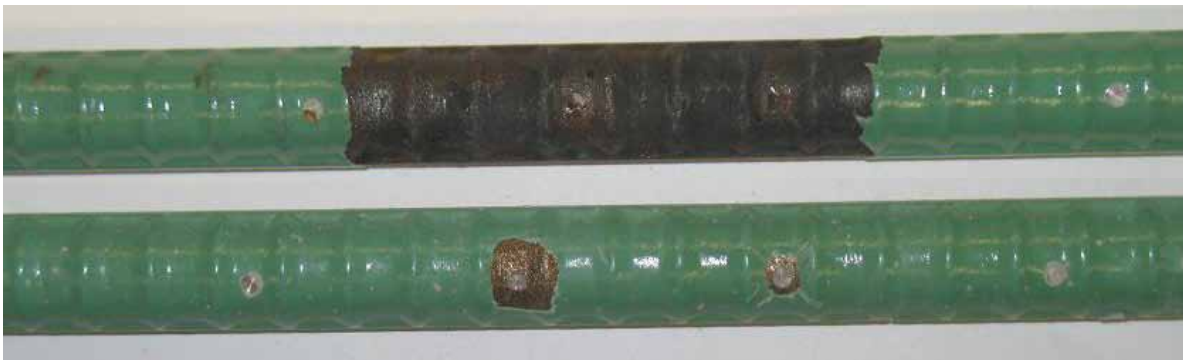
Figure 107. Photo. DuPont™ high-adhesion epoxy-coated top and bottom bars from southern exposure specimen after 96 weeks.
