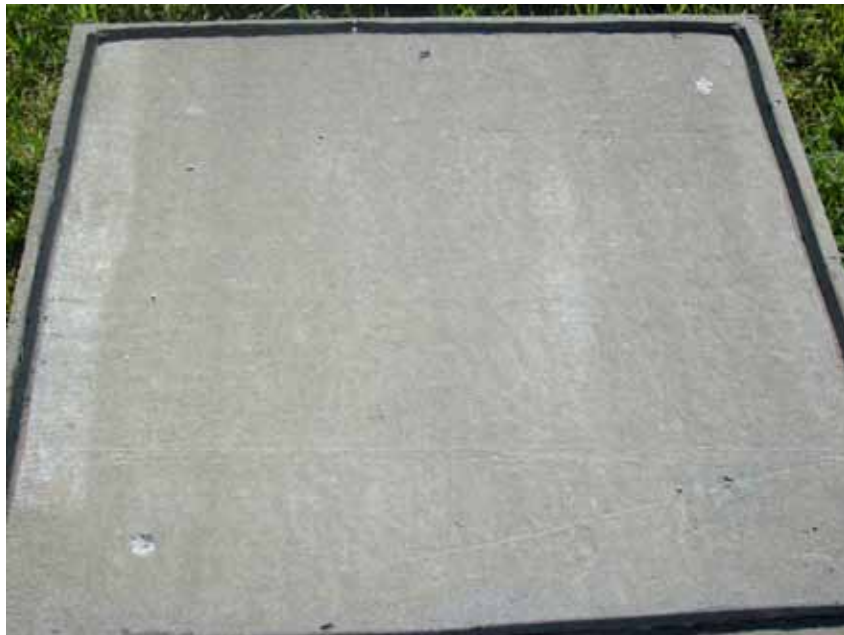
Figure 152. Photo. Field test specimen without simulated cracks containing conventional epoxy-coated steel at 254 weeks.
