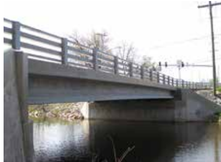
Ultra-high performance concrete (UHPC) is among the innovations being promoted by the Highways for LIFE program's 2012 funding. Structures built using UHPC across the country include the Route 31 bridge in Lyons, NY.
