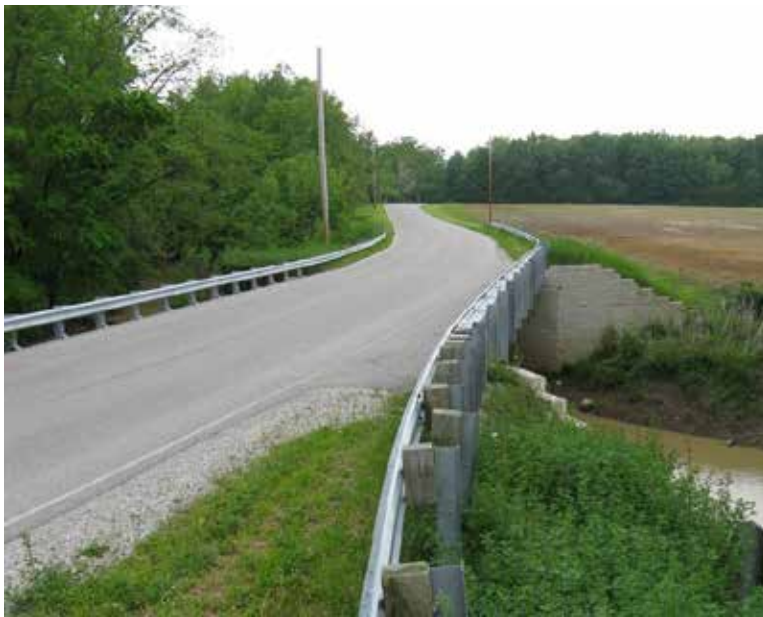
(left) The Bowman Road Bridge in Defiance County, OH, was the first bridge in the world to use the Geosynthetic Reinforced Soil Integrated Bridge System.
