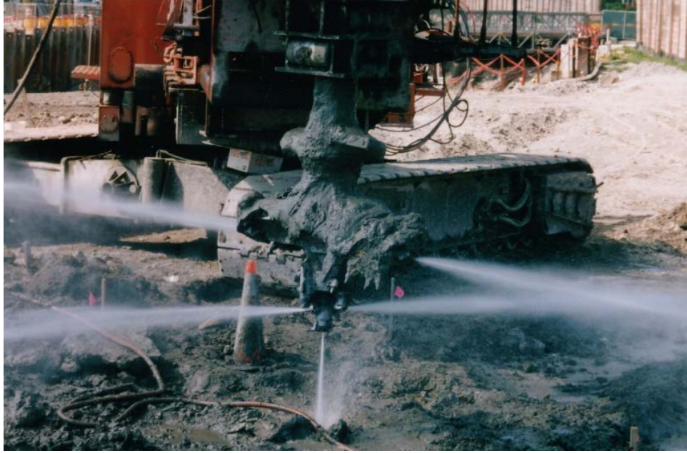
Figure 147. Photo. Example of a WJE tool. (127)
