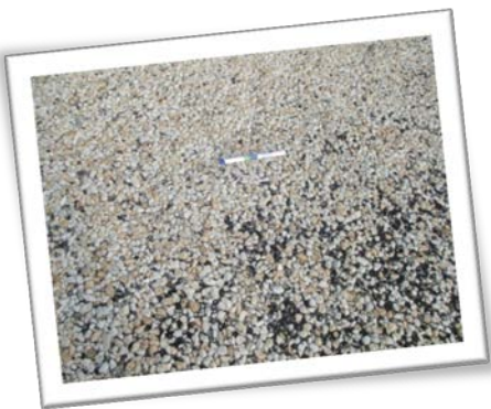
Chip Seal Surface
