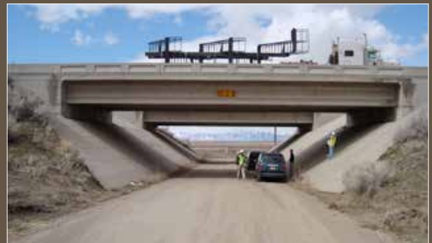
Figure 9. Utah pilot bridge.
