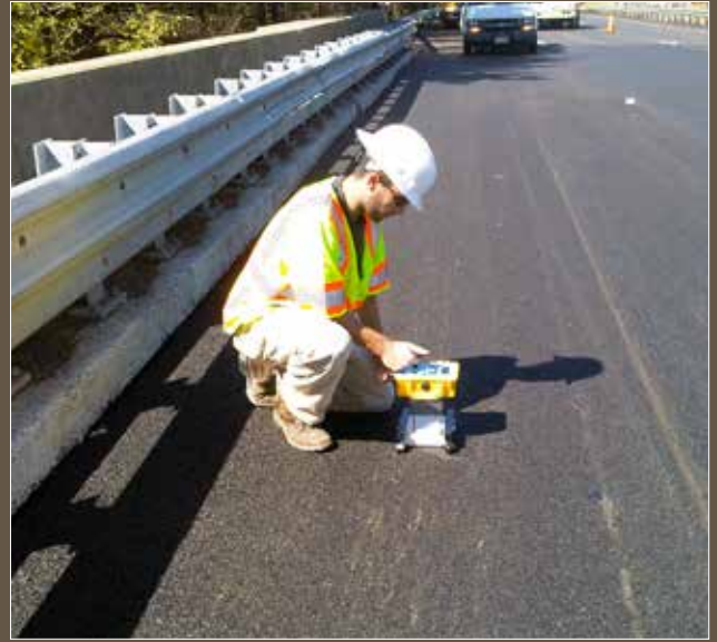
Figure 12. Hydrotracker used on NJ pilot study bridge.
