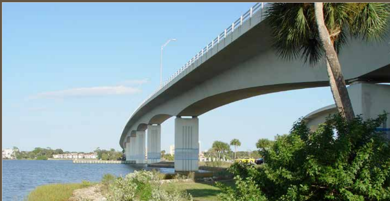
Figure 1. Seabreeze Bridge in Daytona, FL.
