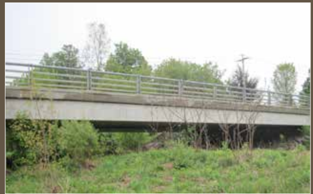
Figure 8. New York pilot bridge.
