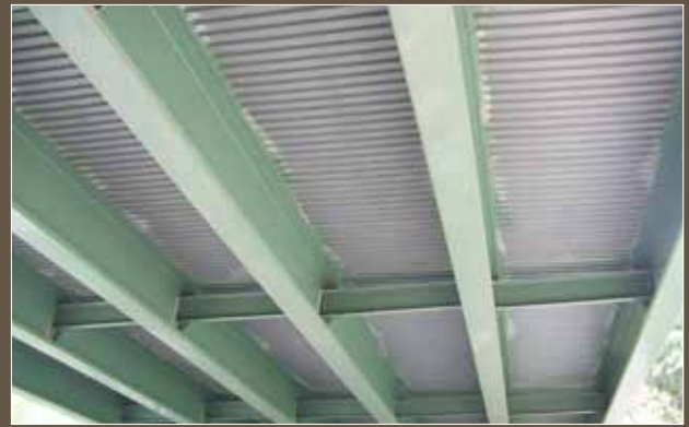
Figure 7. New Jersey pilot bridge.
