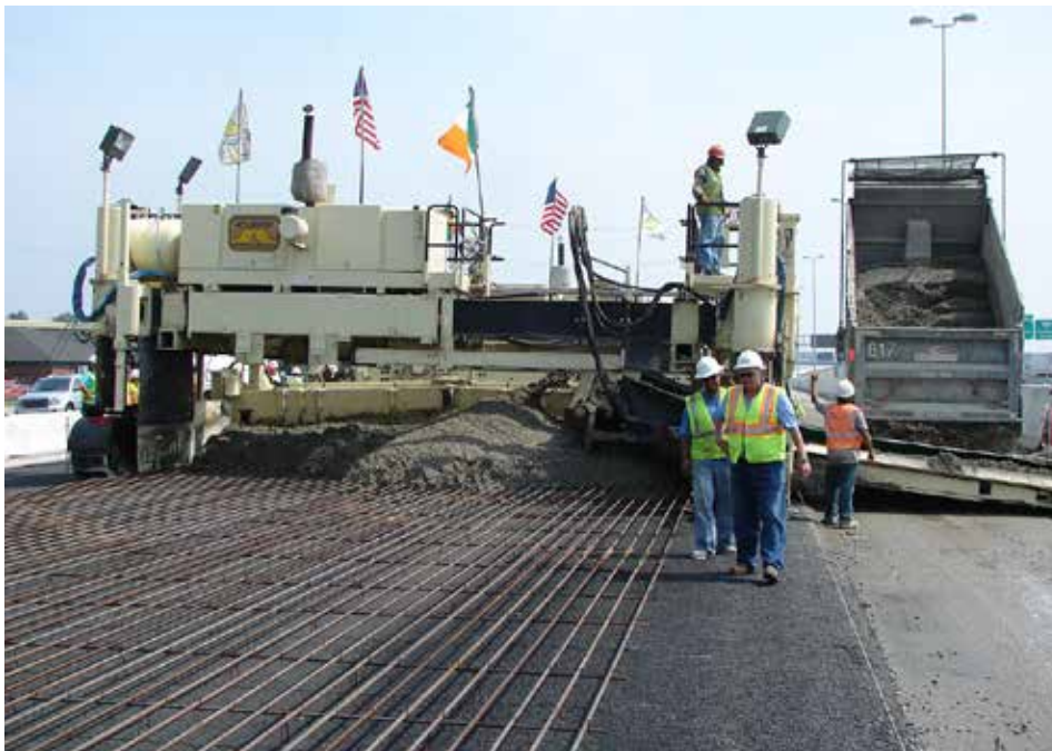
A typical paving operation for CRCP. The pavement is reinforced with continuous steel bars and has minimal maintenance requirements.
