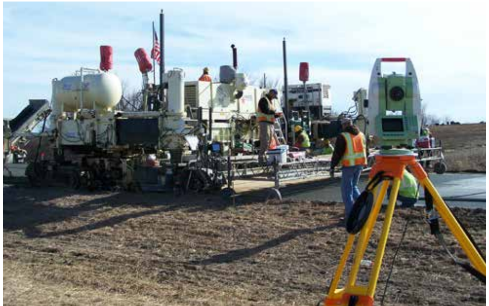
Online training sponsored by the American Concrete Pavement Association and Federal Highway Administration explains the proper use of stringless paving technology.
