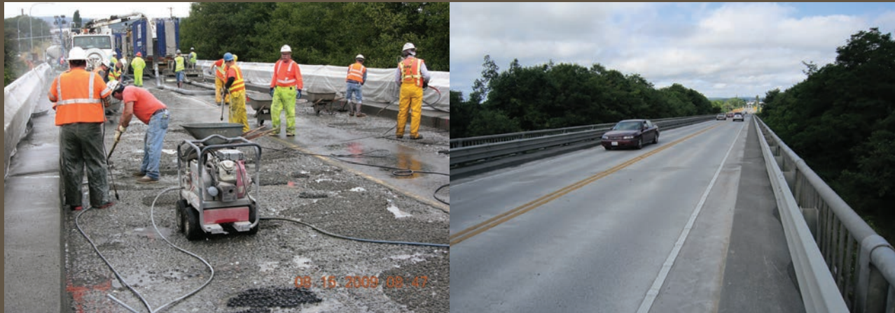
Figure 1. SR532 near Stanwood, WA during construction.
