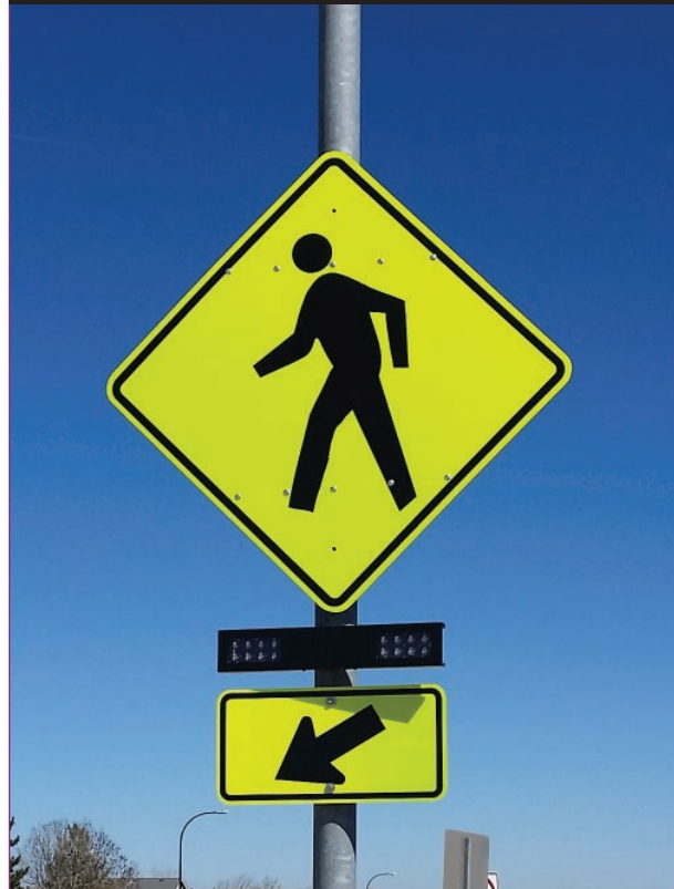
Figure 2. Example of beacons placed below sign.
