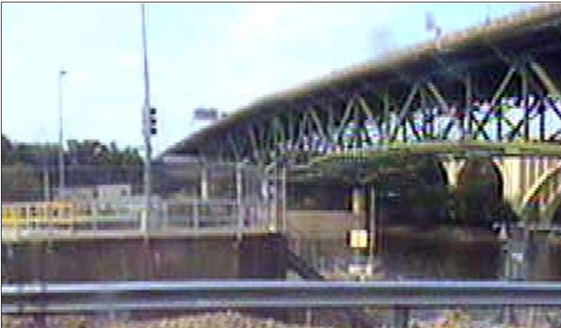
Figure 10. Close-up of first image of collapse sequence, captured by surveillance camera at 18:04:57. The south (near) end of the center span can be seen to have dropped from its position as shown in precollapse images (compare with figure 9).
