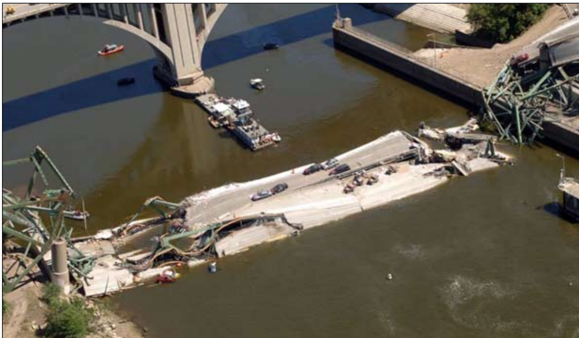
Figure 14. Collapsed bridge center section, looking southeast.
