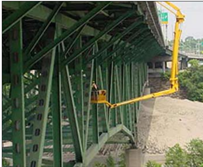
A snooper being used to inspect the I-35W bridge
