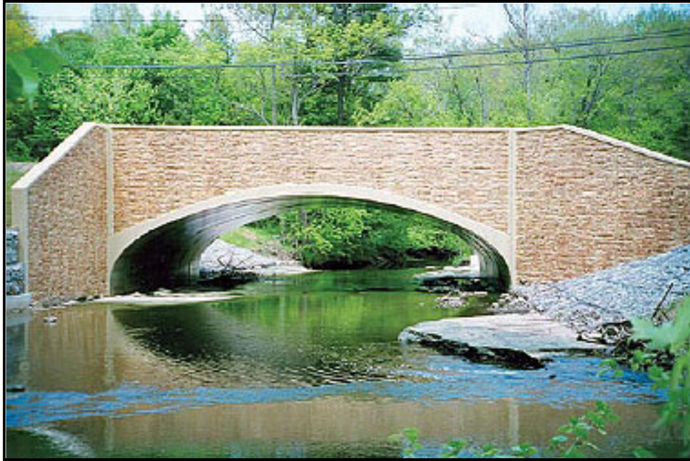
Figure 6.13. Open-bottom culvert on Whitehall Road over Euclid Creek in Cuyahoga County, OH.
